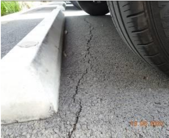
Figure 453 – Crack propagation through car park pavement
