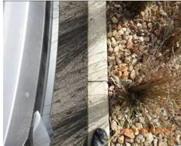
Figure 1150 – Crack propagation through car park kerb
