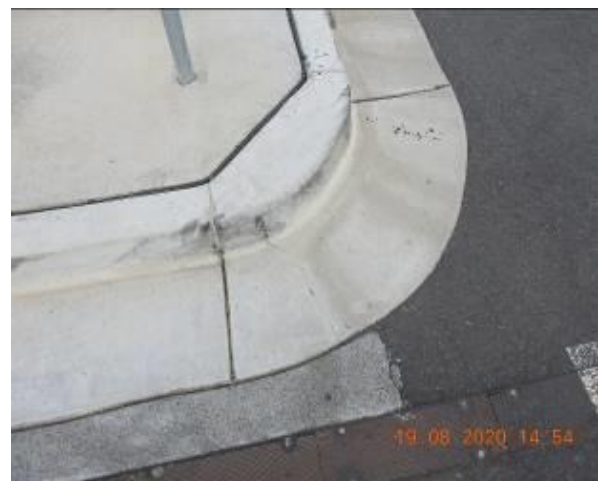
Figure 144 – Crack propagation through car park kerb and gutter
