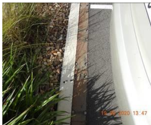
Figure 768 – Crack propagation through car park kerb and service pit
