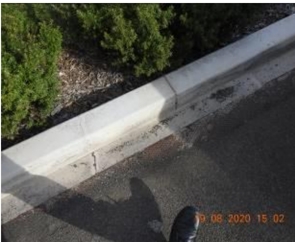
Figure 203 – Crack propagation through car park kerb and gutter
