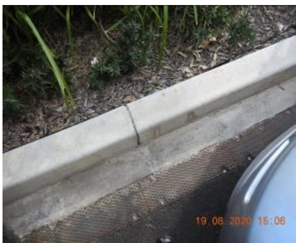
Figure 225 – Crack propagation through car park kerb and gutter
