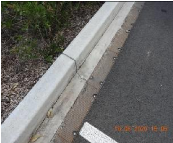
Figure 219 – Crack propagation through car park kerb and gutter
