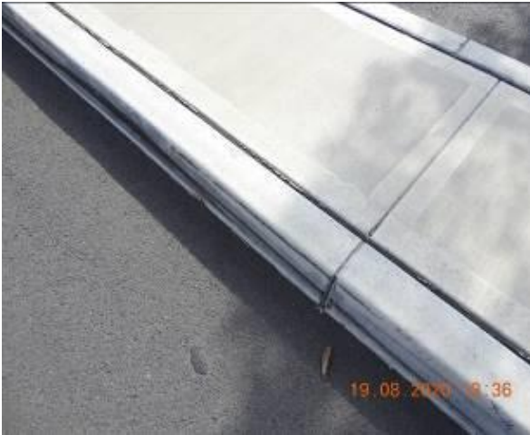
Figure 681 – Crack propagation through traffic island kerb
