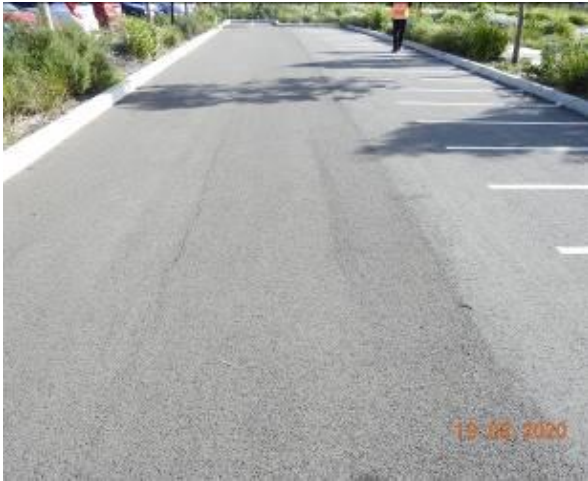
Figure 507 – Crack propagation through car park pavement
