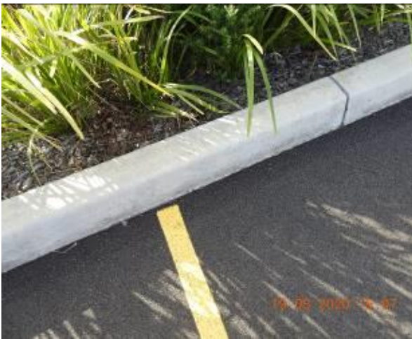
Figure 237 – General condition of car park kerb
