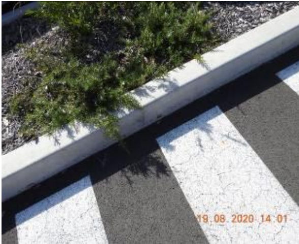
Figure 903 – Crack propagation through car park kerb
