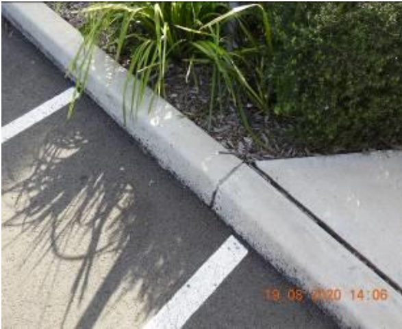
Figure 951 – Crack propagation through car park kerb
