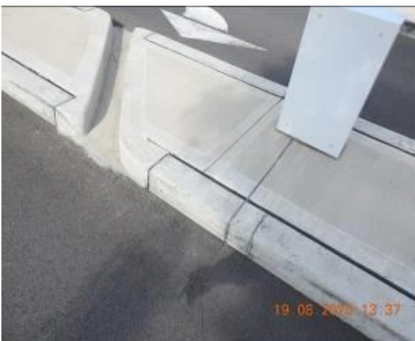
Figure 685 – Crack propagation through traffic island kerb
