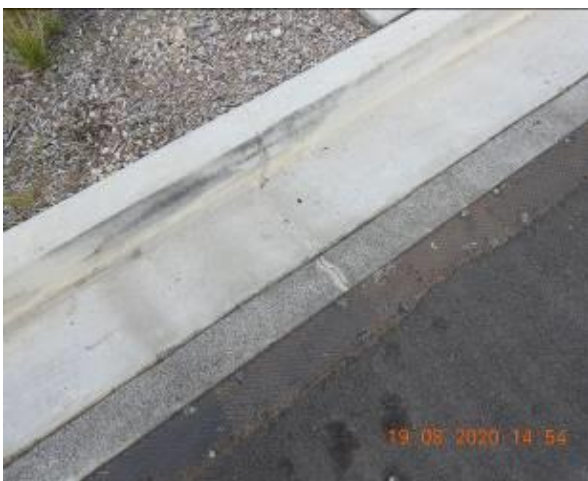
Figure 143 – Crack propagation through car park kerb and gutter
