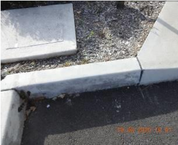
Figure 235 – Hairline cracking through car park kerb
