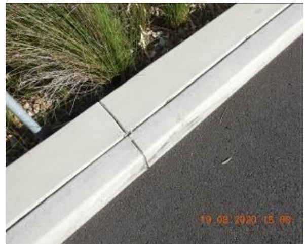
Figure 262 – Crack propagation through car park kerb
