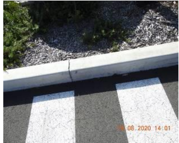
Figure 904 – Crack propagation through car park kerb
