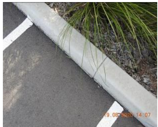
Figure 956 – Crack propagation through car park kerb
