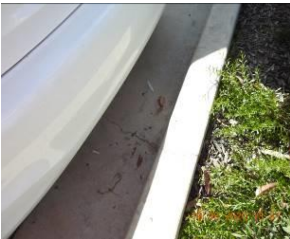
Figure 799 – Crack propagation through car park kerb gutter
