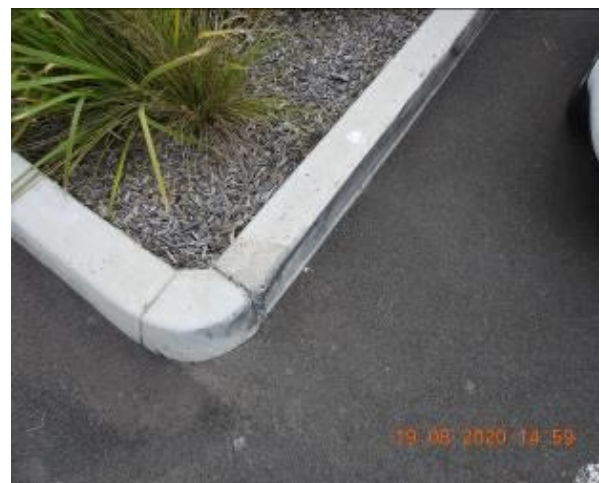
Figure 160 – Crack propagation through car park kerb
