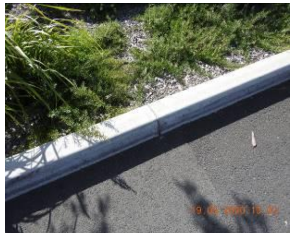
Figure 638 – Crack propagation through car park kerb
