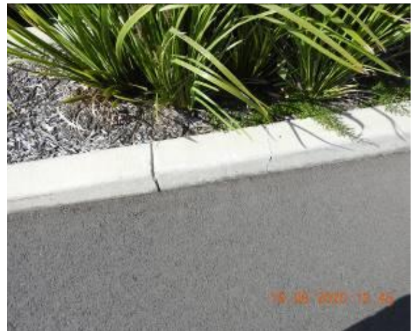
Figure 750 – Crack propagation through car park kerb
