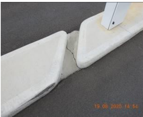
Figure 155 – Crack propagation through traffic island kerb
