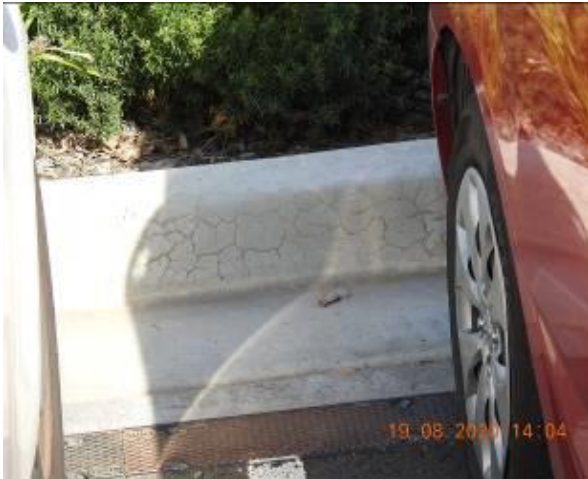
Figure 939 – Hairline cracking through car park kerb
