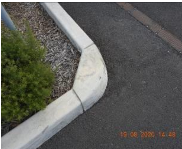
Figure 77 – Crack propagation through car park kerb
