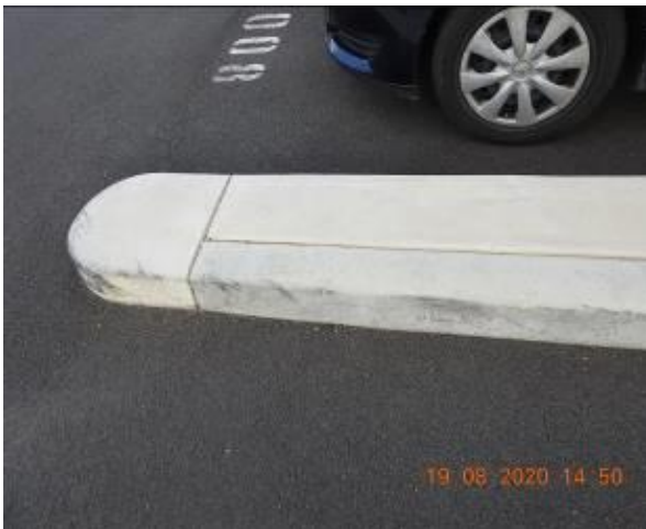
Figure 93 – Hairline cracking through car park kerb
