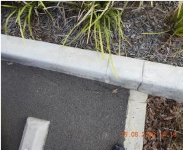
Figure 1083 – Crack propagation through car park kerb
