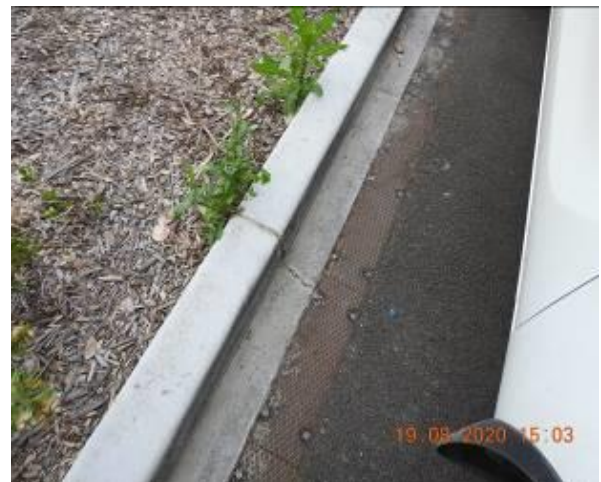
Figure 204 – Crack propagation through car park kerb and gutter
