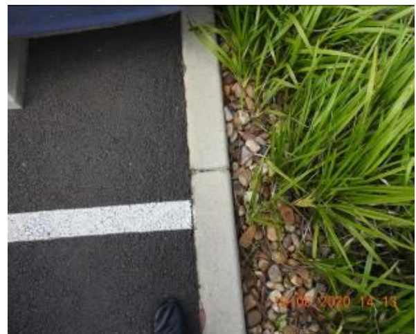
Figure 1022 – Crack propagation through car park kerb
