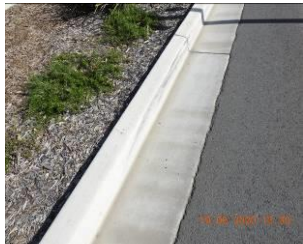
Figure 608 – Crack propagation through car park kerb
