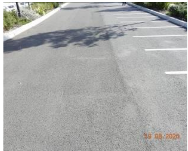
Figure 506 – Crack propagation through car park pavement
