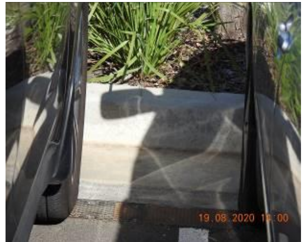
Figure 882 – Hairline cracking through car park kerb
