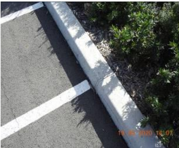
Figure 953 – Crack propagation through car park kerb
