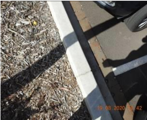
Figure 713 – Crack propagation through car park kerb
