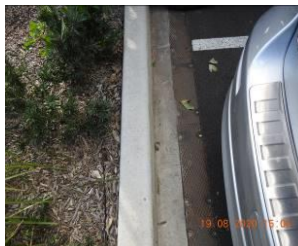
Figure 226 – Hairline cracking through car park gutter
