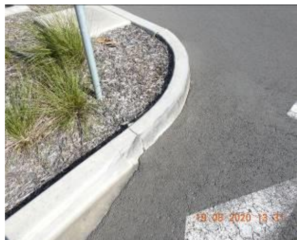
Figure 626 – Crack propagation through car park kerb
