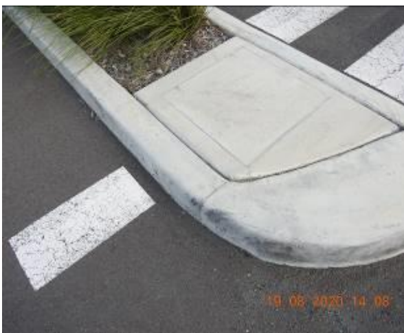
Figure 985 – Hairline cracking through car park kerb
