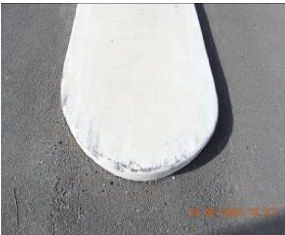
Figure 697 – Loss of material through traffic island kerb
