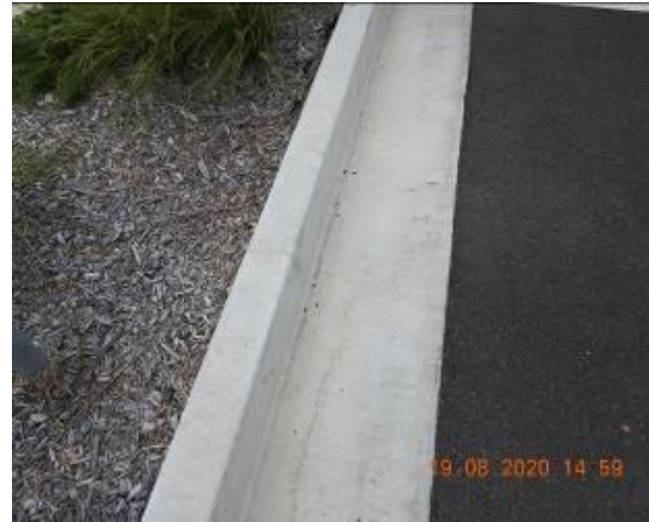
Figure 164 – Crack propagation through car park kerb and gutter
