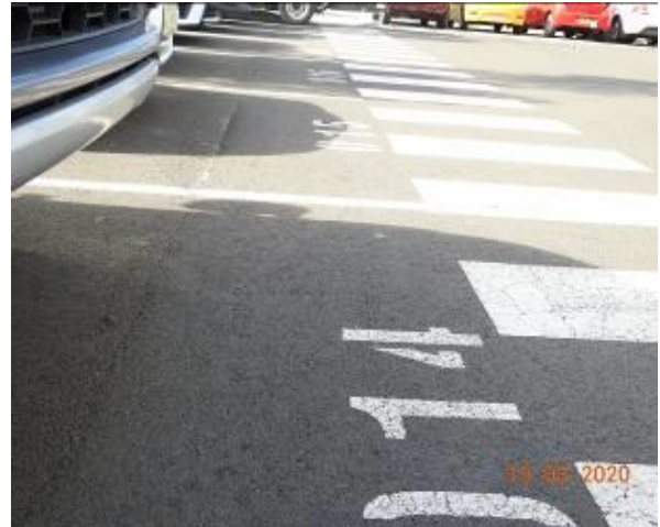
Figure 448 – Crack propagation through car park pavement
