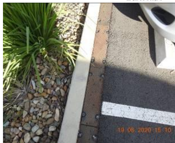
Figure 290 – Evidence of patchwork through car park kerb and service pit
