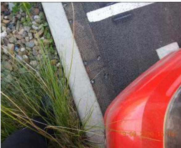
Figure 353 – Crack propagation through car park kerb and service pit
