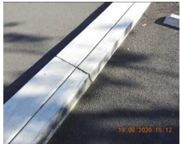
Figure 330 – Crack propagation and loss of material through car park kerb
