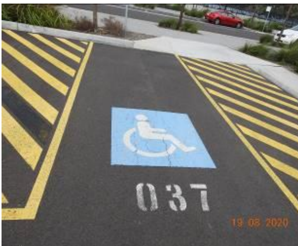
Figure 51 – Crack propagation through car park pavement
