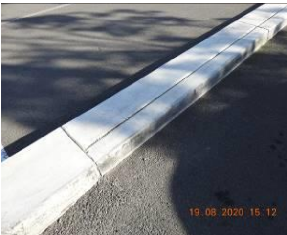
Figure 329 – Crack propagation and loss of material through car park kerb
