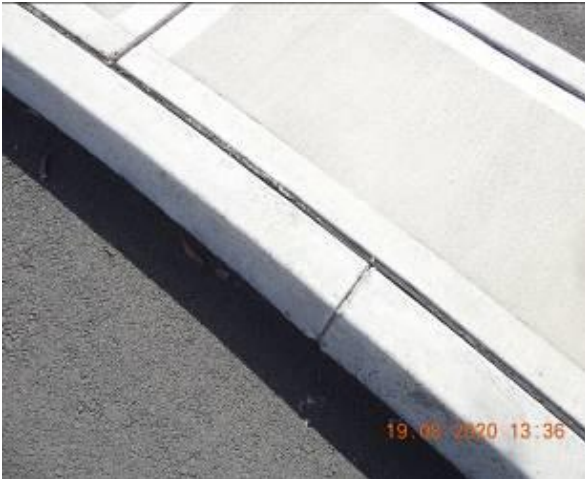
Figure 675 – Crack propagation through traffic island kerb
