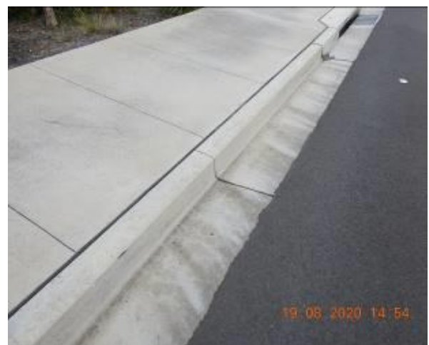
Figure 150 – Hairline cracking through car park kerb
