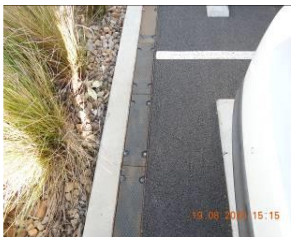
Figure 359 – Crack propagation through car park kerb and service pit
