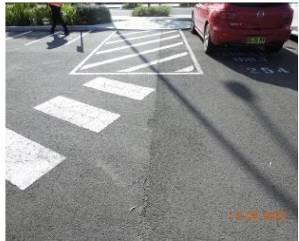
Figure 504 – Loss of material through car park pavement
