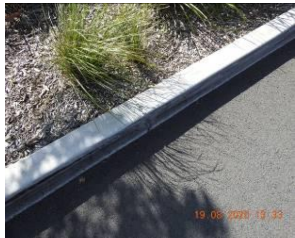
Figure 632 – Crack propagation through car park kerb
