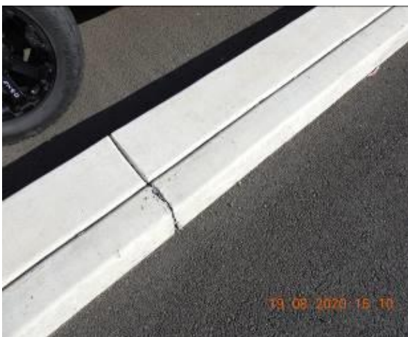
Figure 285 – Crack propagation through car park kerb
