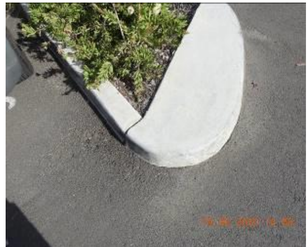
Figure 948 – Hairline cracking through car park kerb
