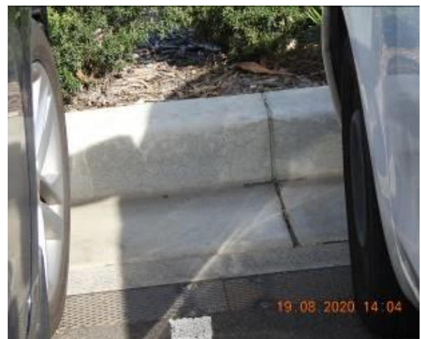
Figure 938 – Hairline cracking through car park kerb
