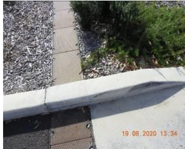
Figure 652 – Crack propagation through car park kerb
