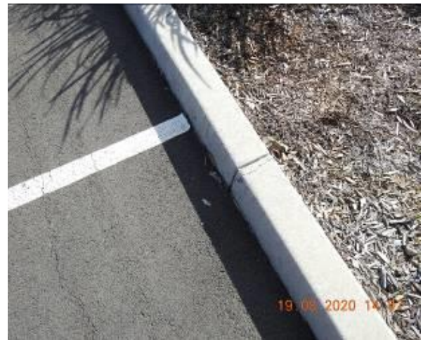
Figure 954 – Crack propagation through car park kerb
