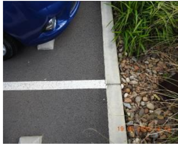
Figure 1074 – Crack propagation through car park kerb
