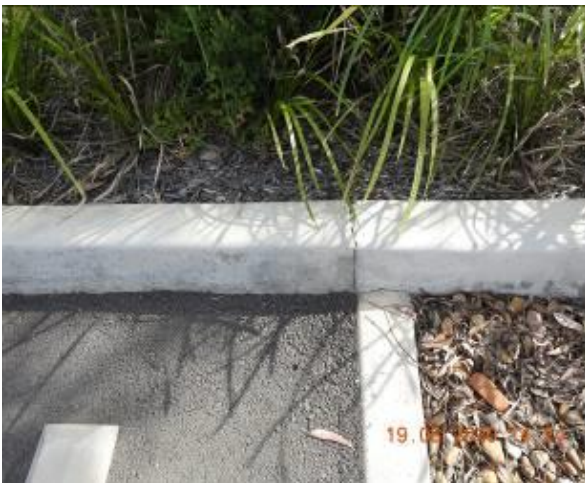
Figure 1169 – Crack propagation through car park kerb
