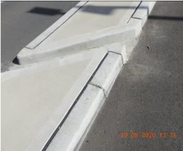
Figure 663 – Crack propagation through traffic island kerb
