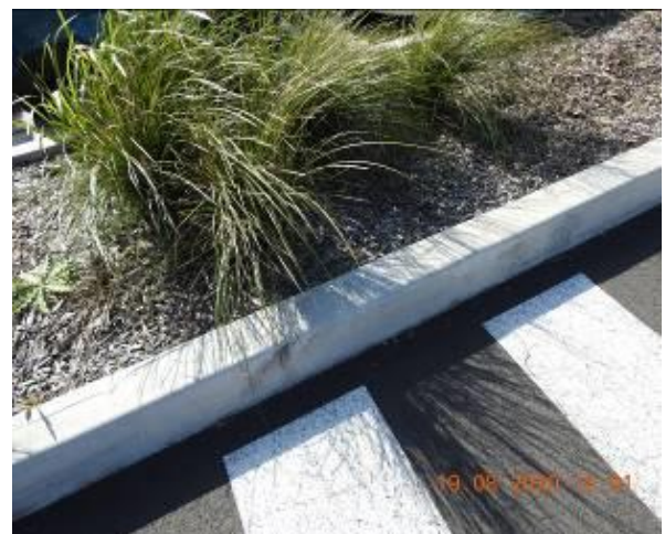
Figure 902 – Crack propagation through car park kerb
