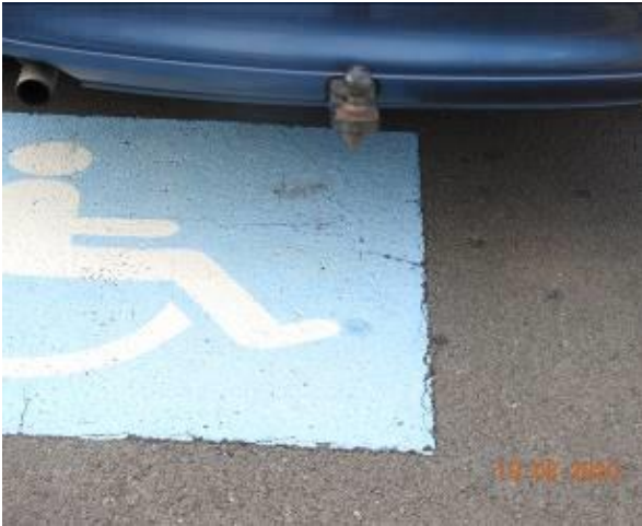
Figure 13 – Crack propagation through car park pavement
