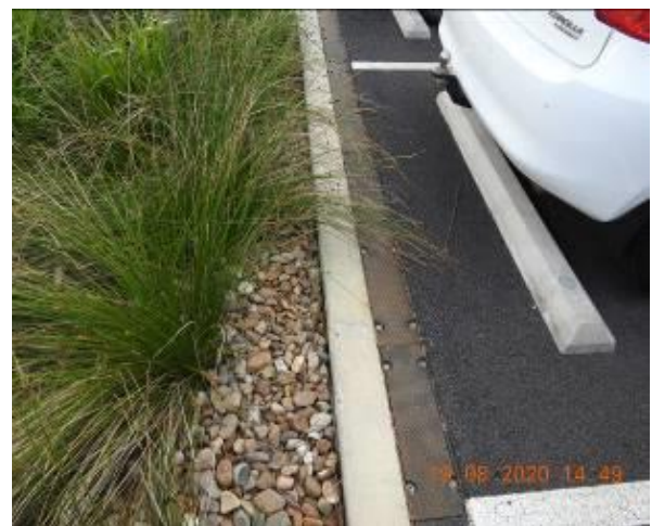
Figure 88 – Evidence of patchwork through car park kerb
