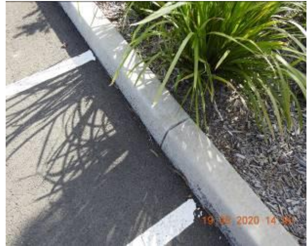
Figure 952 – Crack propagation through car park kerb
