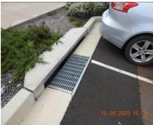
Figure 171 – General condition of kerb inlet pit and stormwater inlet pit
