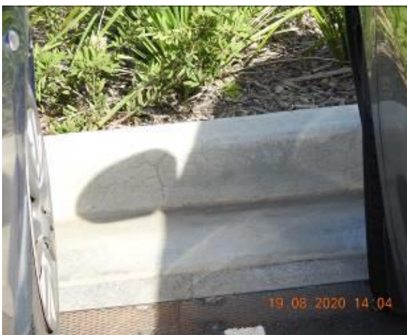
Figure 937 – Hairline cracking through car park kerb
