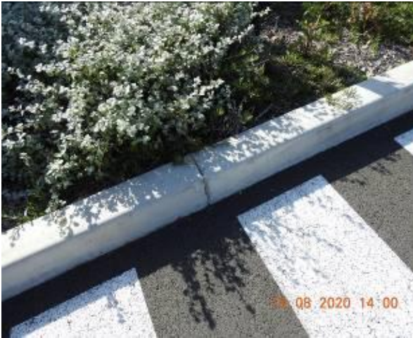
Figure 891 – Crack propagation through car park kerb
