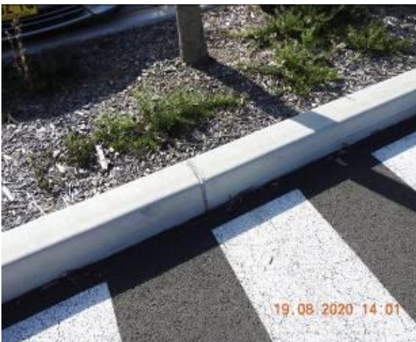
Figure 895 – Crack propagation through car park kerb
