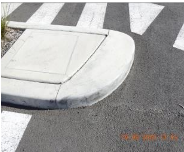
Figure 845 – Hairline cracking through car park kerb
