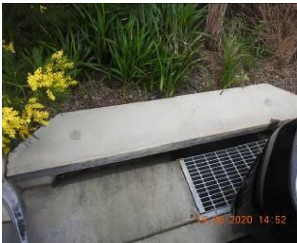
Figure 129 – General condition of kerb inlet pit and stormwater inlet pit
