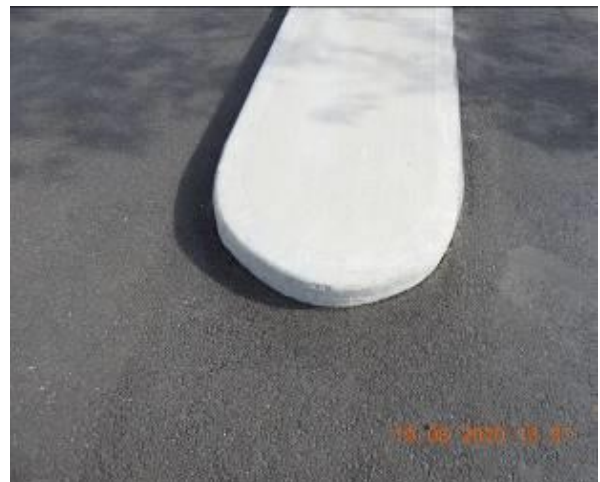
Figure 698 – Loss of material through traffic island kerb
