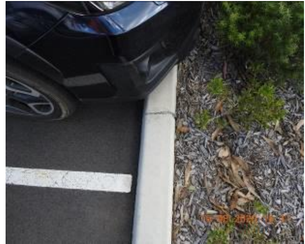
Figure 1000 – Crack propagation through car park kerb
