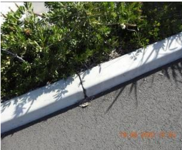
Figure 839 – Crack propagation through car park kerb
