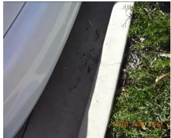
Figure 798 – Crack propagation through car park kerb and gutter
