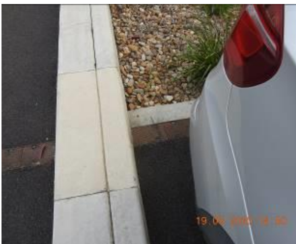
Figure 99 – Evidence of patchwork through car park kerb
