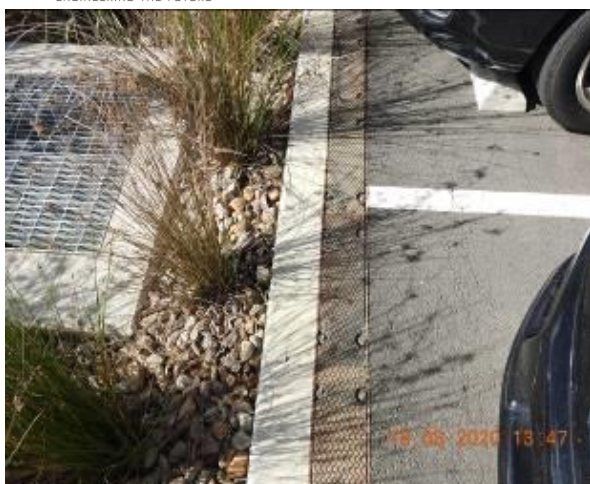
Figure 765 – Crack propagation through car park kerb and General condition of service pit
