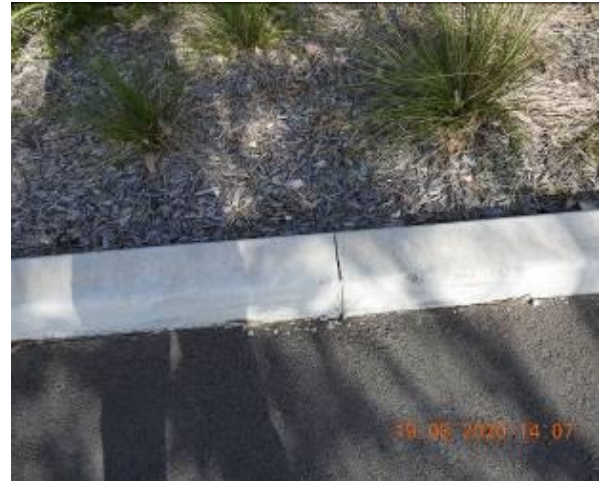
Figure 970 – Crack propagation through car park kerb
