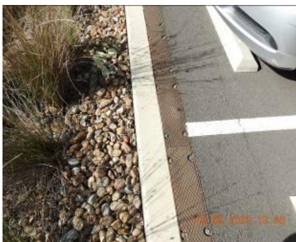
Figure 763 – Crack propagation through car park kerb and General condition of service pit
