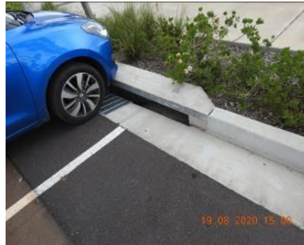
Figure 166 – General condition of kerb inlet pit and stormwater inlet pit
