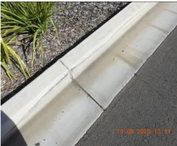
Figure 623 – Crack propagation through car park kerb
