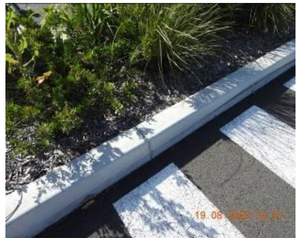
Figure 896 – Crack propagation through car park kerb
