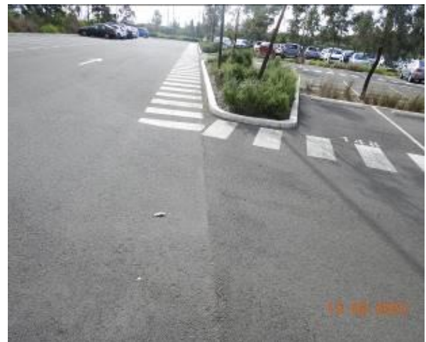
Figure 590 – Evidence of patchwork through car park pavement
