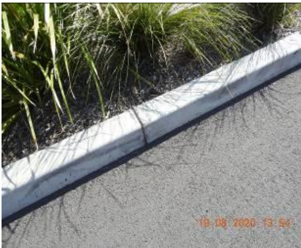
Figure 833 – Crack propagation through car park kerb
