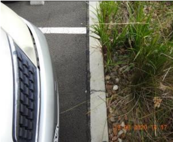
Figure 1053 – Crack propagation through car park kerb
