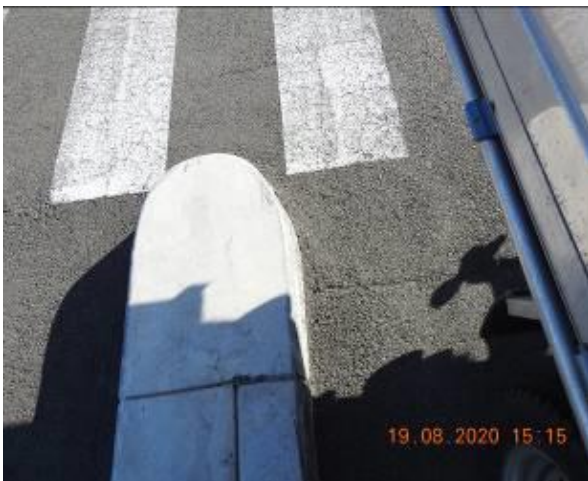
Figure 365 – Hairline cracking through car park kerb
