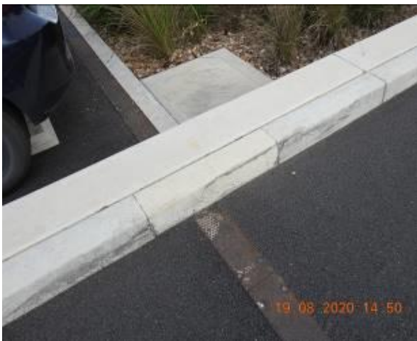
Figure 95 – Hairline cracking through car park kerb
