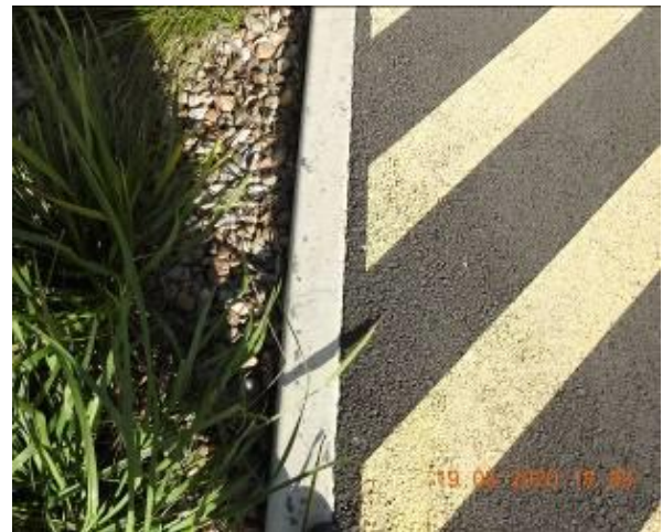
Figure 268 – Crack propagation through car park kerb
