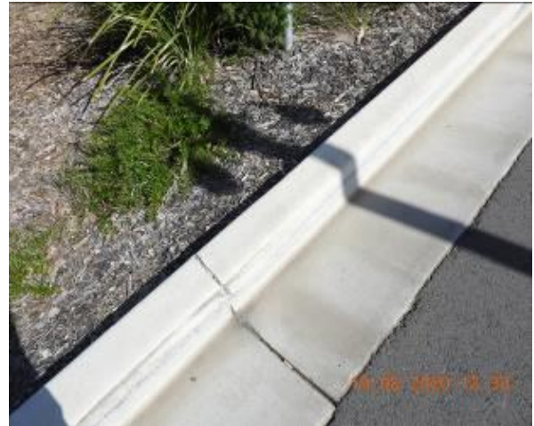
Figure 610 – Crack propagation through car park kerb
