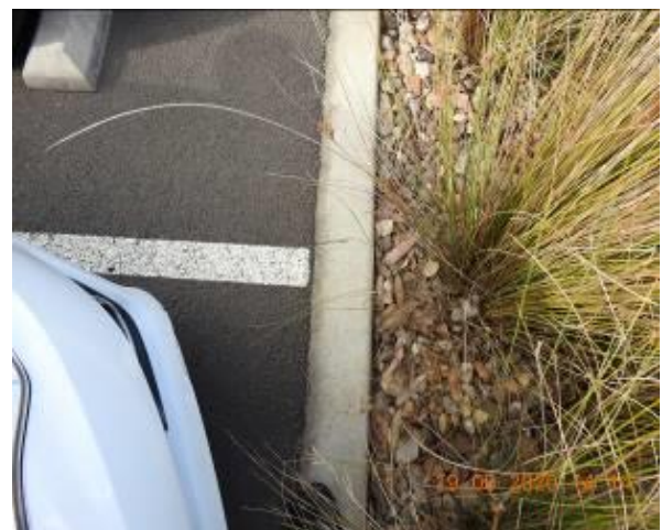
Figure 1028 – Crack propagation through car park kerb
