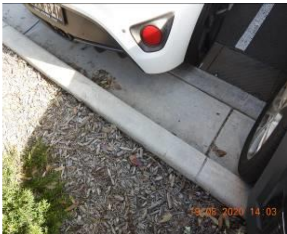
Figure 919 – Hairline cracking through car park kerb
