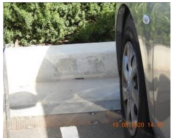
Figure 944 – Hairline cracking through car park gutter
