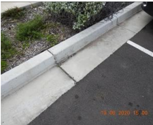
Figure 167 – Crack propagation and loss of material through car park kerb and gutter
