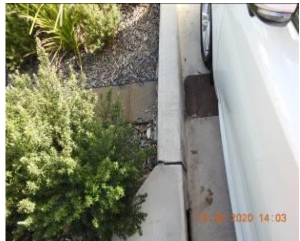
Figure 926 – Crack propagation through car park kerb
