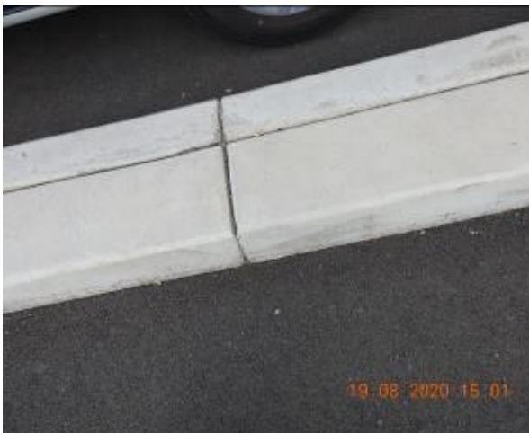
Figure 179 – Crack propagation through car park kerb
