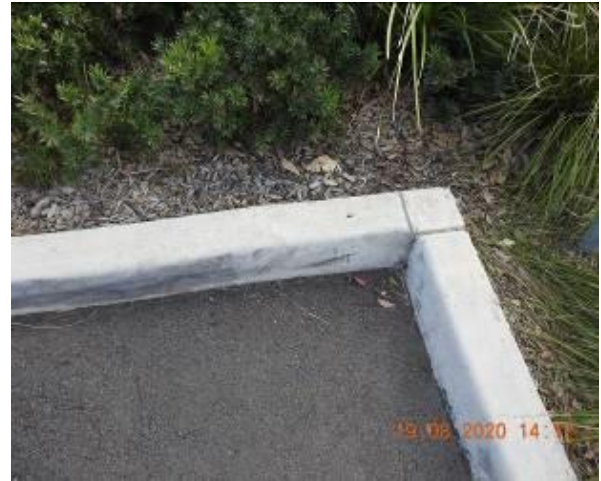
Figure 1012 – Crack propagation through car park kerb
