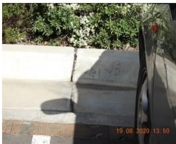
Figure 791 – Crack propagation through car park gutter
