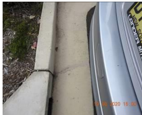
Figure 172 – Evidence of patchwork through and crack propagation through car park gutter
