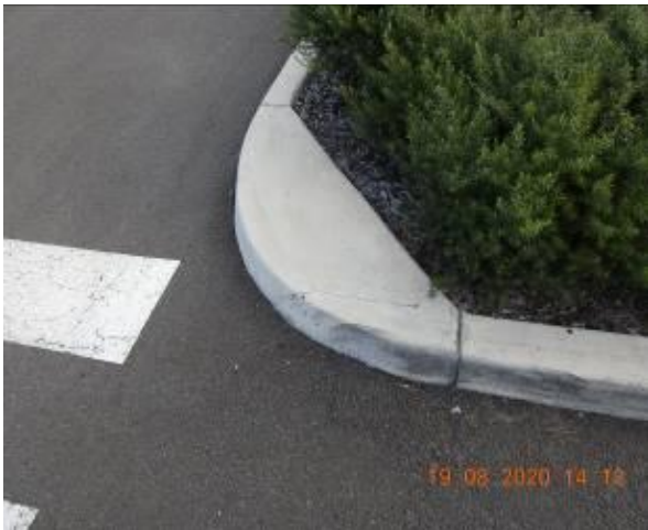
Figure 1013 – Crack propagation through car park kerb
