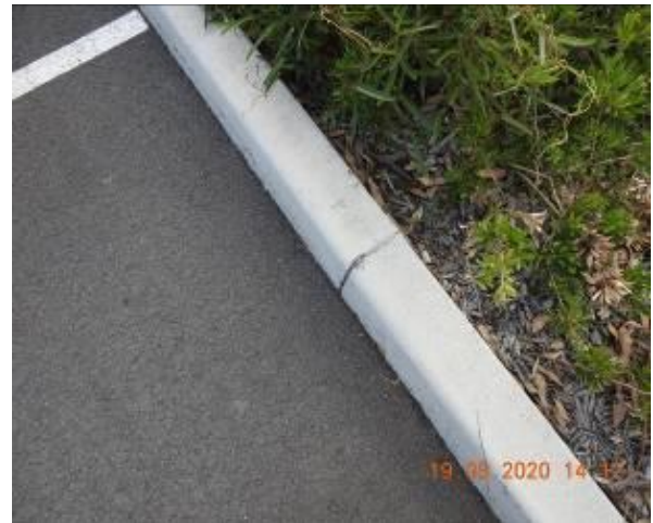
Figure 1008 – Crack propagation through car park kerb
