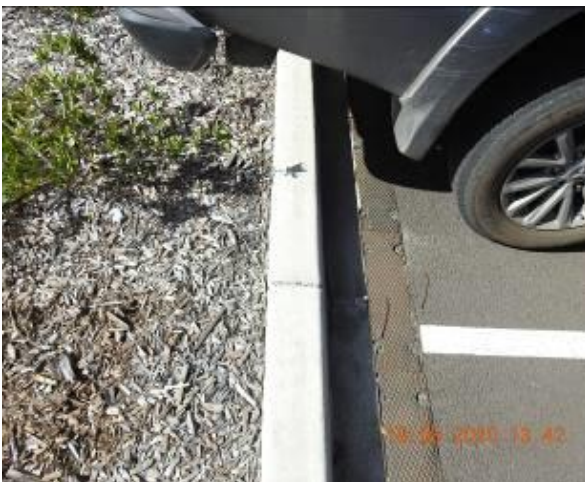
Figure 715 – Crack propagation through car park kerb
