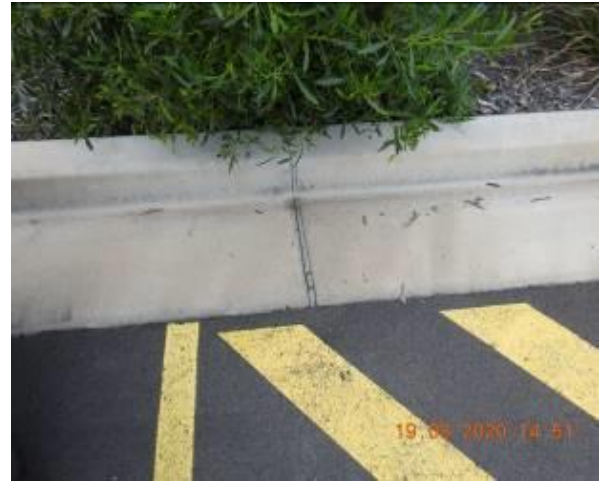
Figure 122 – Loss of material through car park kerb and gutter
