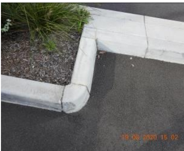
Figure 197 – Crack propagation through car park kerb
