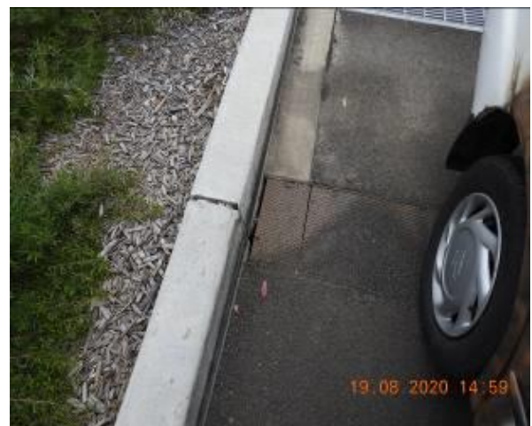
Figure 162 – Crack propagation and loss of material through car park kerb
