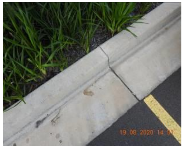
Figure 120 – Crack propagation through car park kerb and gutter
