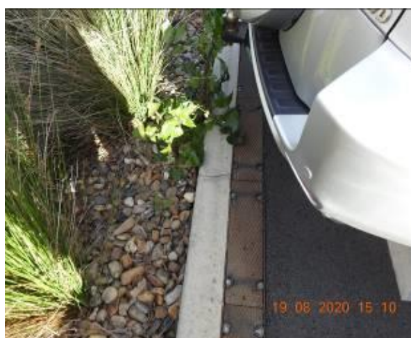
Figure 291 – Crack propagation through car park kerb and service pit
