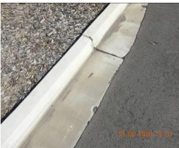
Figure 625 – Crack propagation and loss of material through car park kerb and gutter
