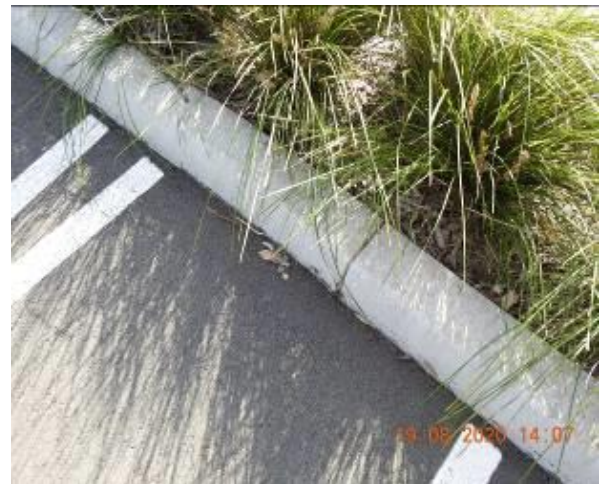
Figure 960 – Crack propagation through car park kerb
