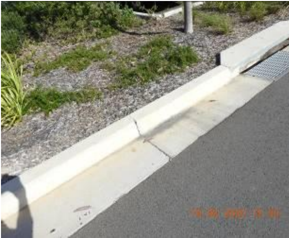
Figure 603 – Crack propagation and loss of material through car park kerb and gutter
