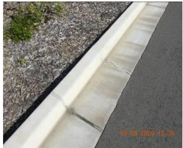
Figure 612 – Crack propagation through car park kerb and gutter
