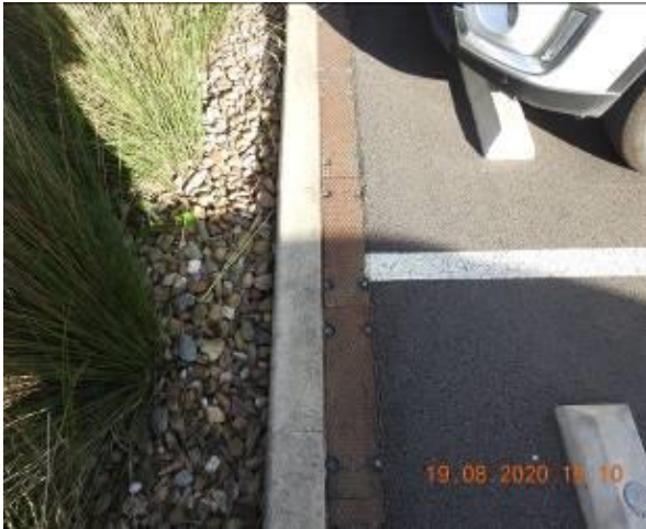
Figure 295 – Crack propagation through car park kerb and service pit
