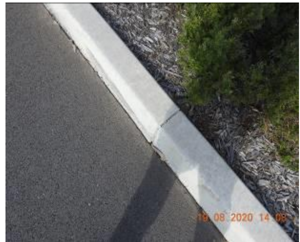
Figure 972 – Crack propagation through car park kerb
