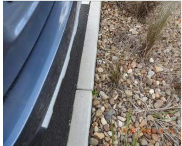
Figure 1096 – Crack propagation through car park kerb
