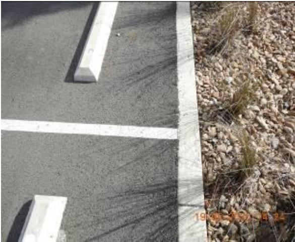
Figure 1167 – Crack propagation through car park kerb
