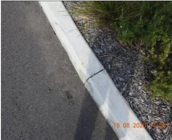
Figure 981 – Crack propagation through car park kerb
