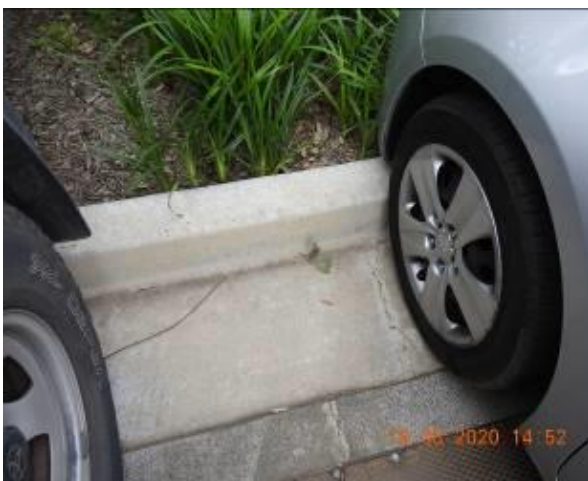
Figure 131 – Crack propagation through car park kerb and gutter
