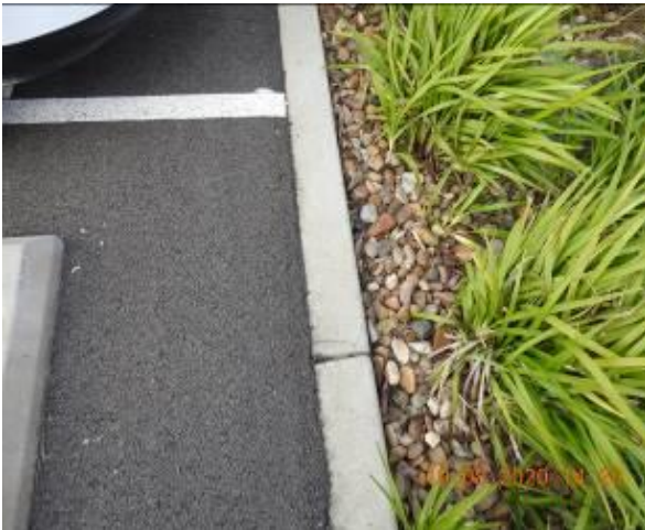
Figure 1097 – Crack propagation through car park kerb
