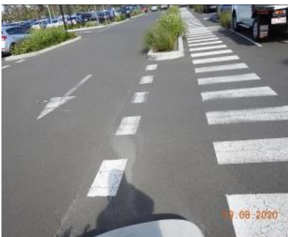
Figure 511 – Crack propagation through car park pavement
