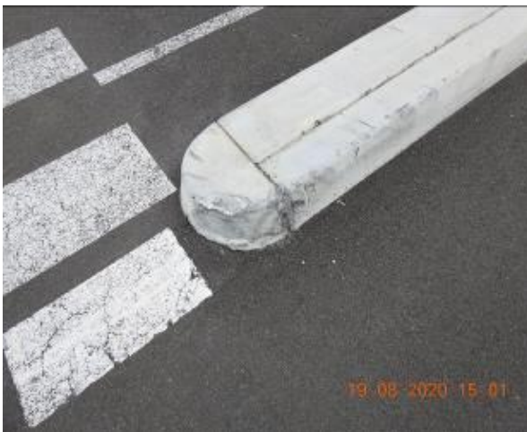
Figure 185 – Loss of material through car park kerb
