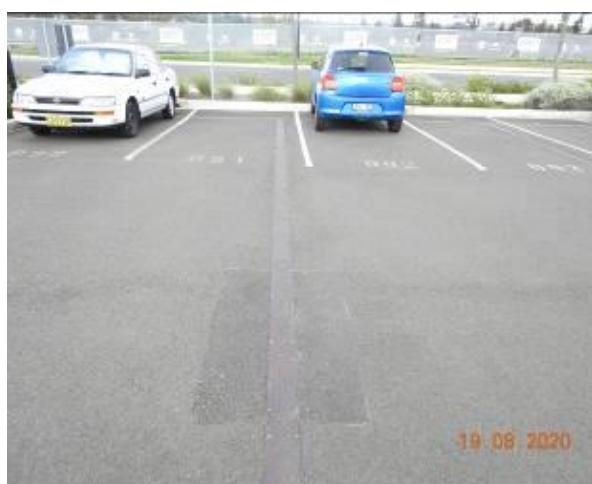
Figure 27 – Evidence of patchwork through car park pavement and general condition of service pit
