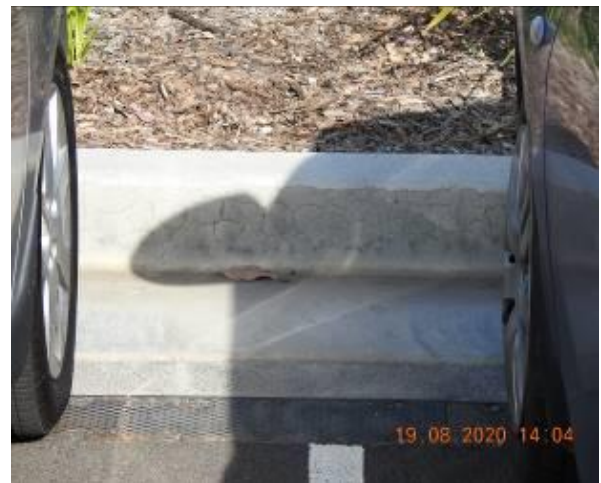
Figure 936 – Hairline cracking through car park kerb
