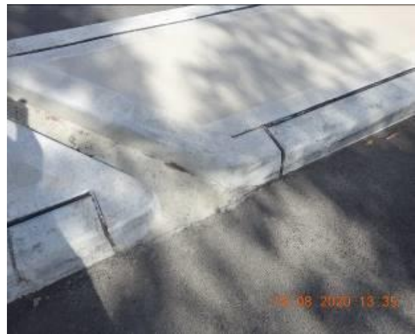
Figure 662 – Crack propagation through traffic island kerb
