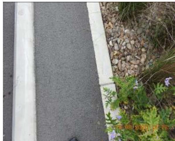
Figure 1076 – Crack propagation through car park kerb
