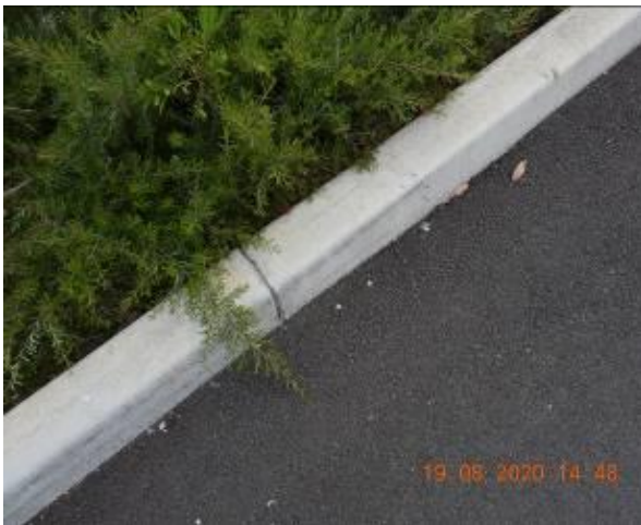
Figure 75 – Crack propagation through car park kerb
