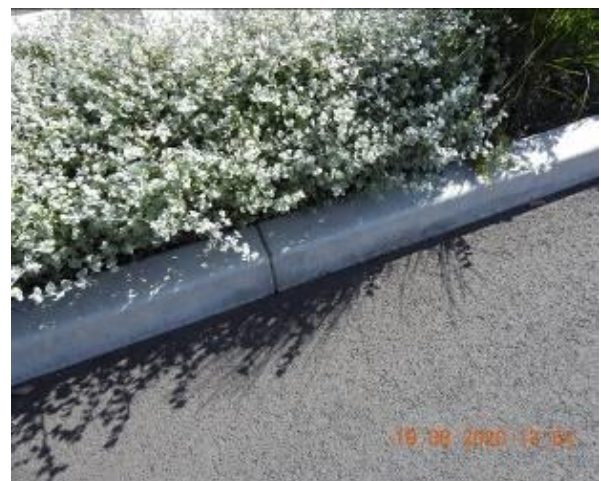
Figure 830 – Crack propagation through car park kerb
