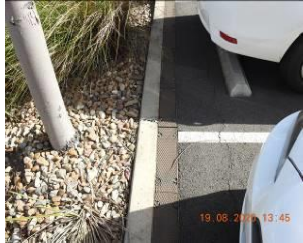
Figure 742 – Crack propagation and loss of material through car park kerb and General condition of service pit
