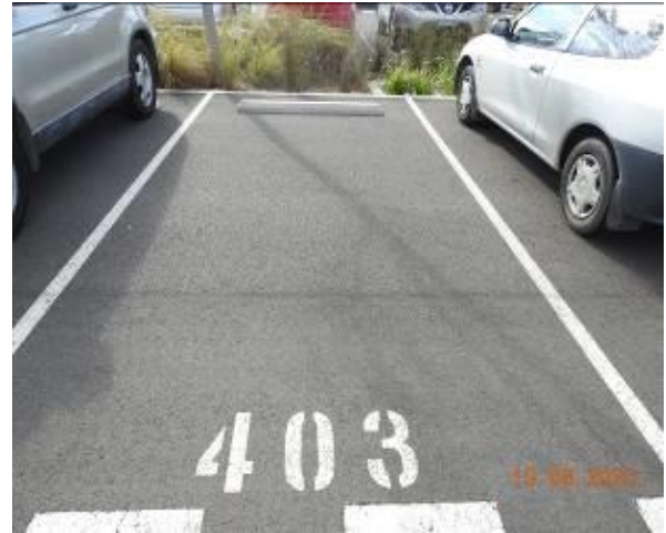
Figure 562 – Crack propagation through car park pavement
