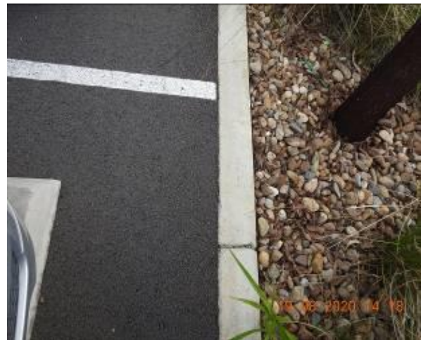
Figure 1080 – Crack propagation through car park kerb
