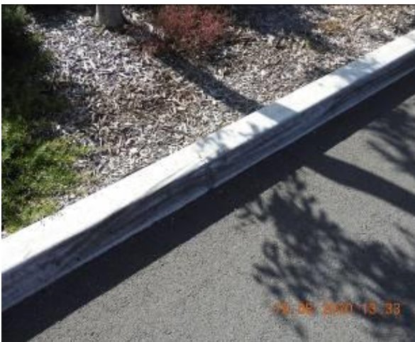
Figure 631 – Crack propagation through car park kerb
