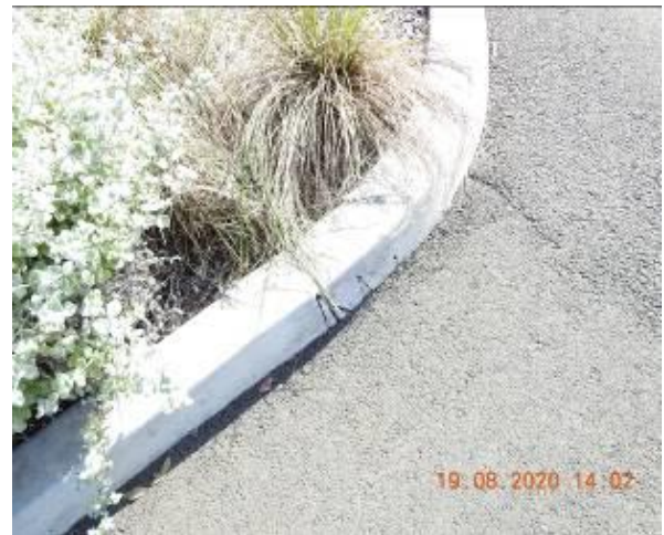
Figure 912 – Hairline cracking through car park kerb
