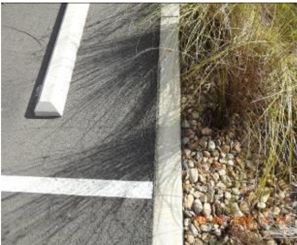
Figure 1151 – Crack propagation through car park kerb
