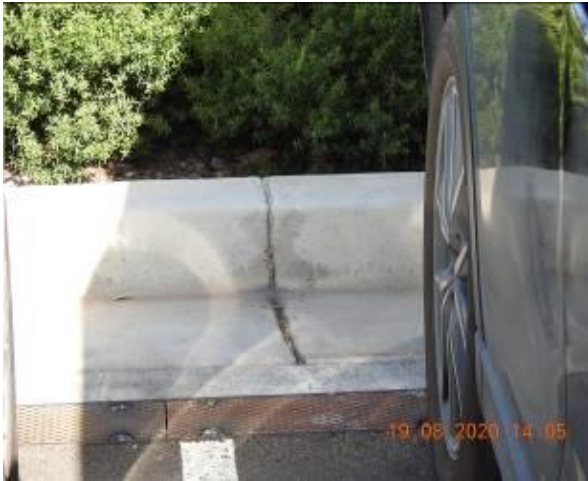
Figure 945 – Crack propagation through car park kerb
