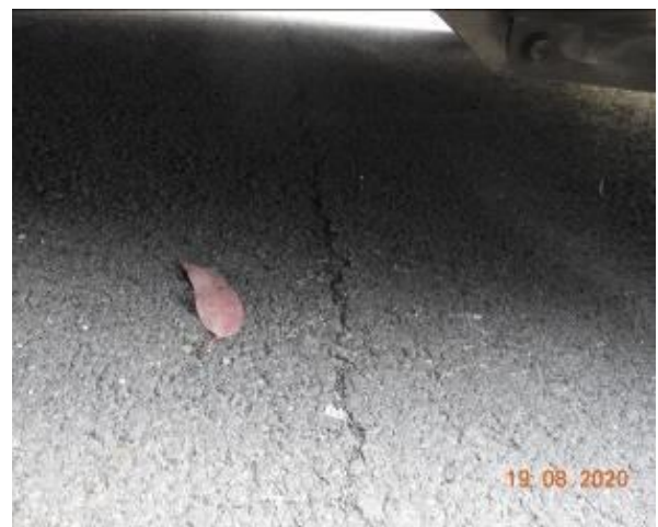
Figure 518 – Crack propagation through car park pavement
