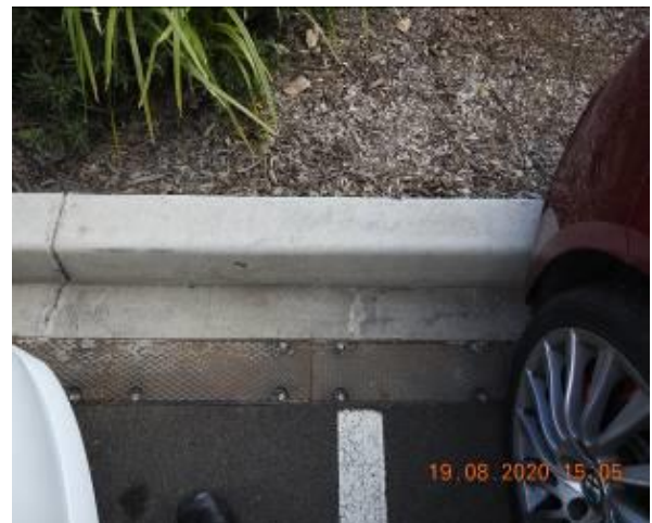
Figure 222 – Crack propagation through car park gutter
