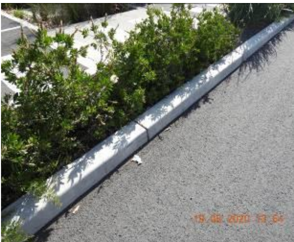
Figure 823 – Hairline cracking through car park kerb
