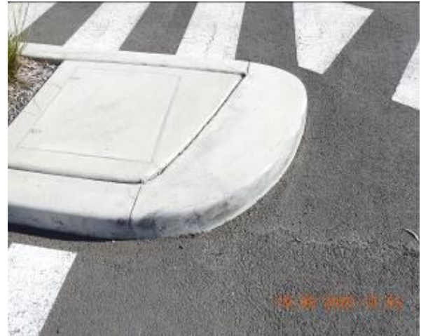
Figure 844 – Hairline cracking through car park kerb
