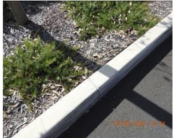
Figure 646 – Crack propagation through car park kerb
