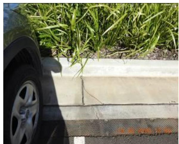
Figure 878 – Hairline cracking through car park kerb
