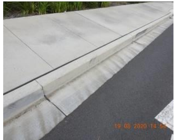
Figure 148 – Hairline cracking through car park kerb
