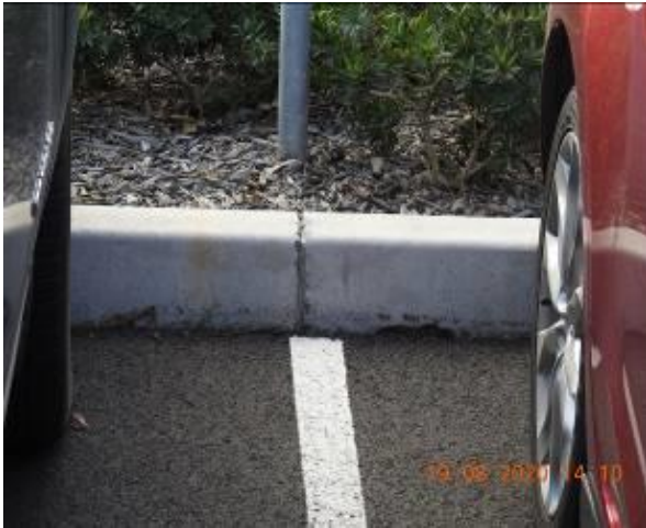
Figure 993 – Crack propagation through car park kerb
