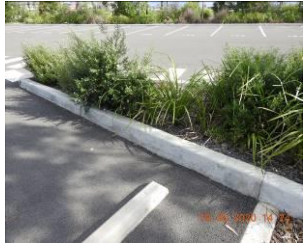
Figure 1168 – Crack propagation through car park kerb
