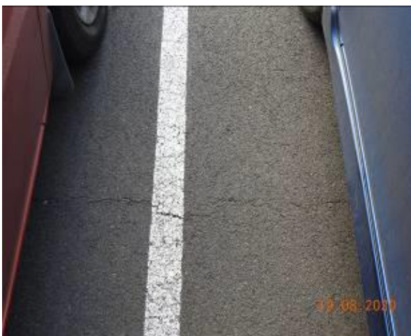
Figure 517 – Crack propagation through car park pavement
