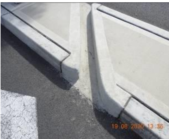
Figure 679 – Crack propagation through traffic island kerb
