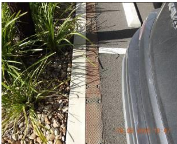
Figure 769 – Crack propagation through car park kerb and service pit
