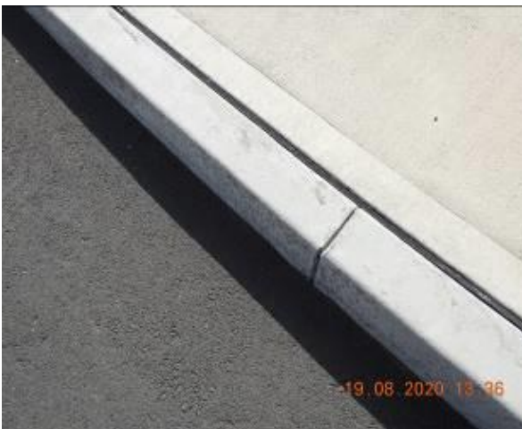
Figure 673 – Crack propagation through traffic island kerb
