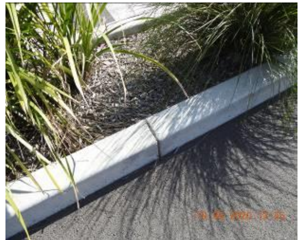
Figure 840 – Crack propagation through car park kerb
