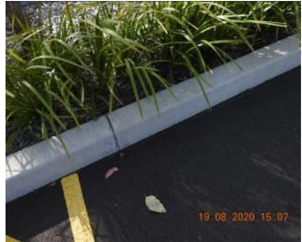
Figure 248 – Crack propagation through car park kerb
