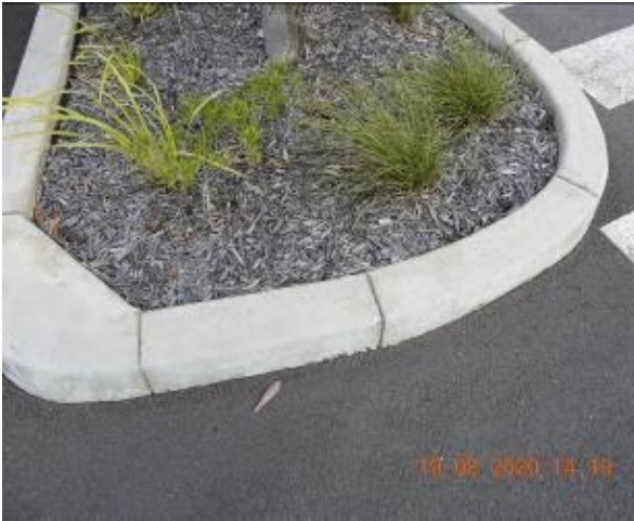
Figure 1089 – Crack propagation through car park kerb
