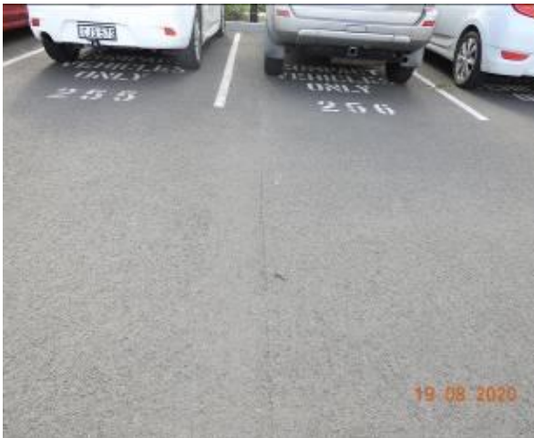
Figure 483 – Crack propagation through car park pavement
