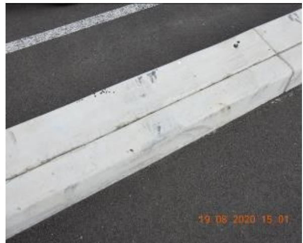
Figure 186 – Hairline cracking through car park kerb
