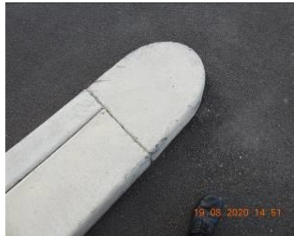
Figure 112 – Hairline cracking through car park kerb
