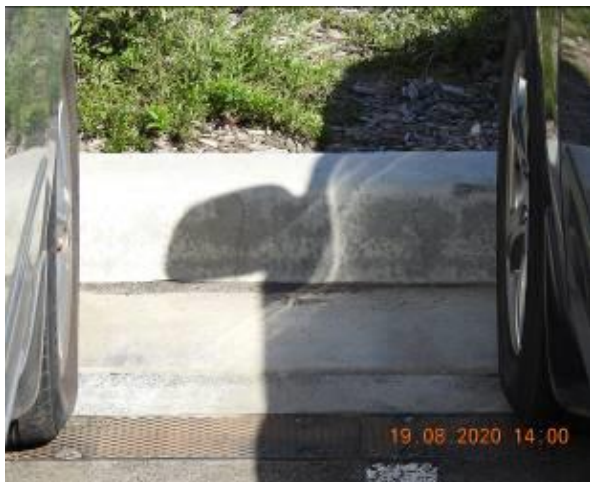
Figure 883 – Hairline cracking through car park kerb
