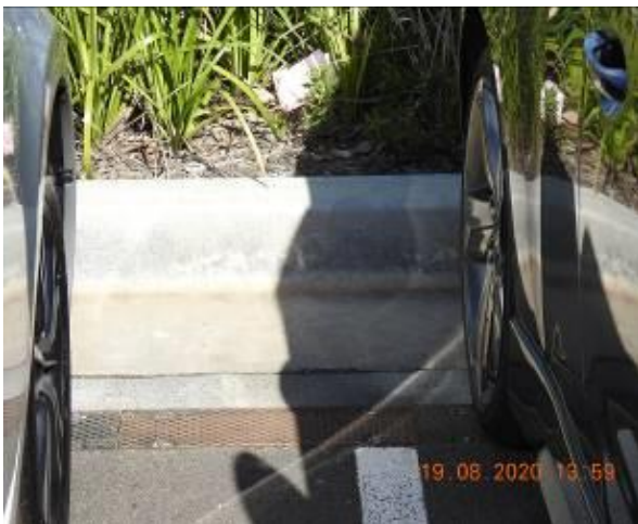
Figure 875 – Hairline cracking through car park kerb
