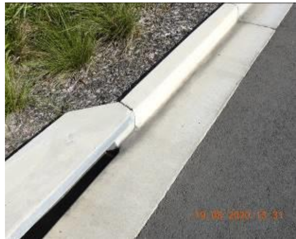
Figure 618 – Crack propagation through car park kerb
