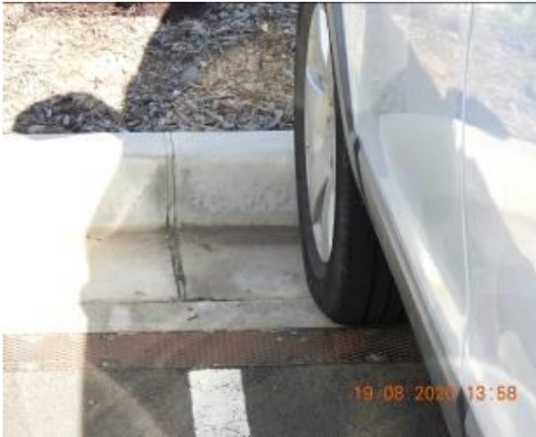
Figure 873 – Crack propagation through car park kerb
