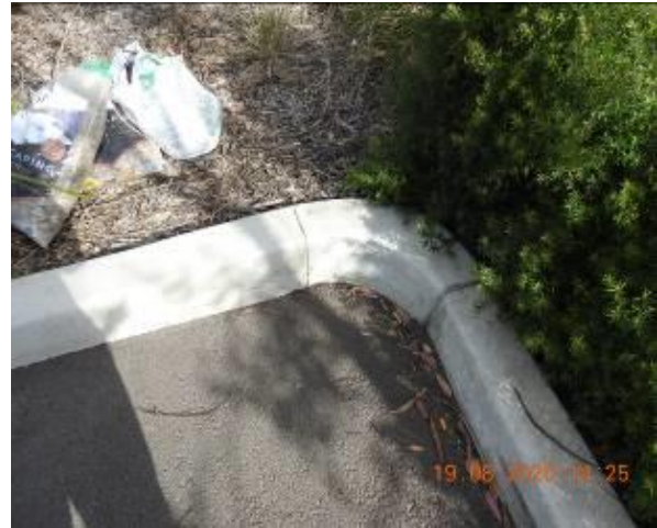
Figure 1174 – Crack propagation through car park kerb
