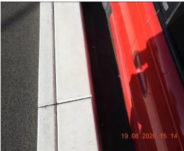
Figure 351 – Crack propagation through car park kerb
