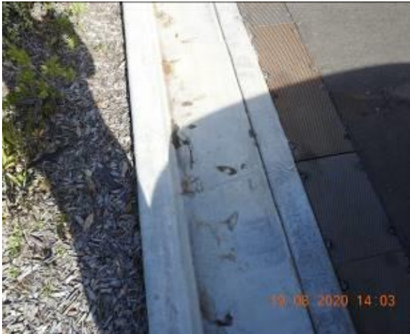
Figure 921 – Crack propagation through car park kerb and gutter
