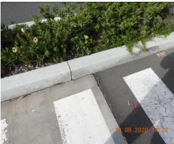
Figure 1129 – Crack propagation through car park kerb
