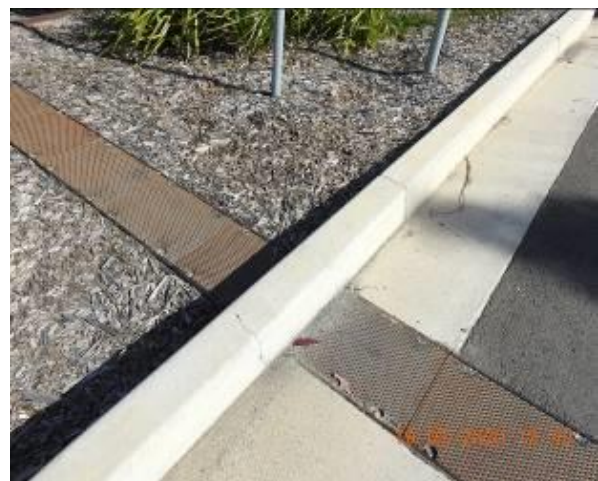
Figure 602 – Crack propagation through car park kerb
