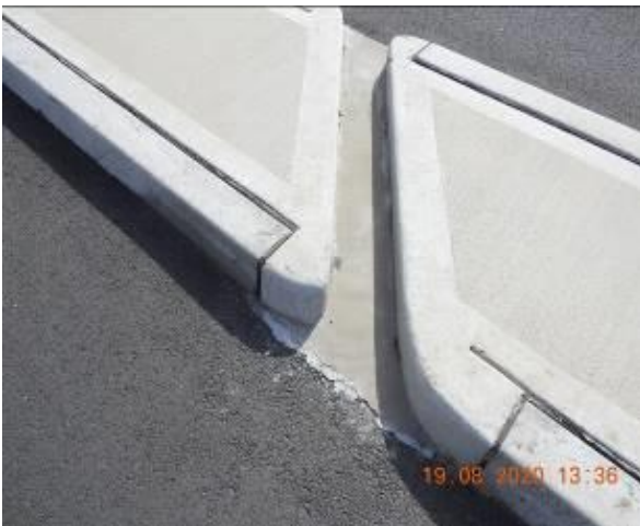
Figure 677 – Crack propagation through traffic island kerb
