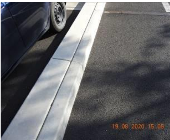
Figure 281 – Crack propagation through car park kerb
