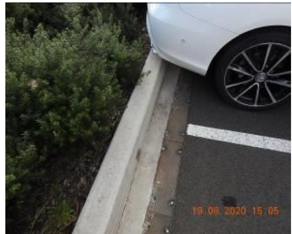
Figure 220 – Crack propagation through car park kerb and gutter
