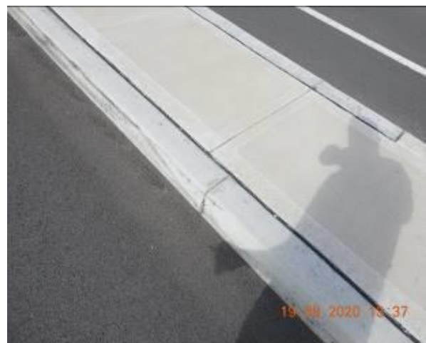
Figure 686 – Crack propagation through traffic island kerb
