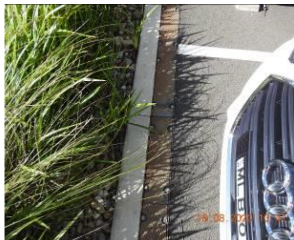
Figure 770 – Crack propagation through car park kerb and service pit
