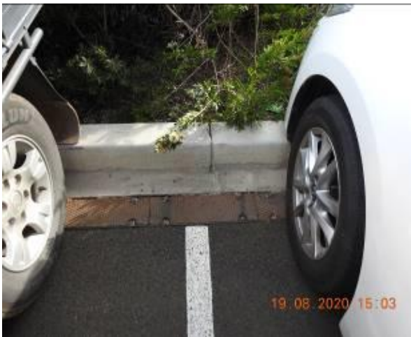
Figure 207 – Crack propagation through car park kerb and gutter
