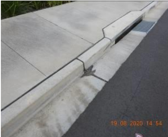
Figure 151 – Hairline cracking through car park kerb
