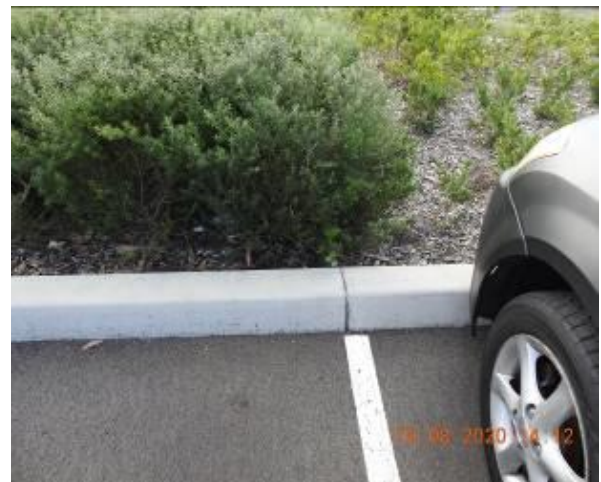
Figure 1004 – Crack propagation through car park kerb
