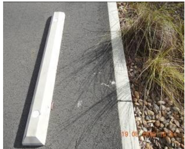
Figure 1164 – Crack propagation through car park kerb
