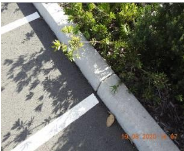
Figure 961 – Crack propagation through car park kerb
