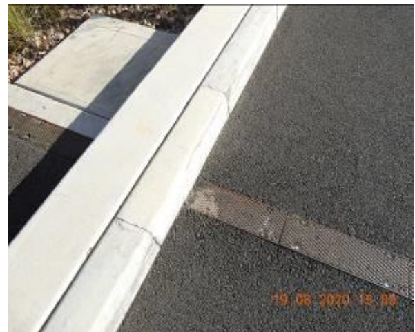
Figure 282 – Crack propagation through car park kerb
