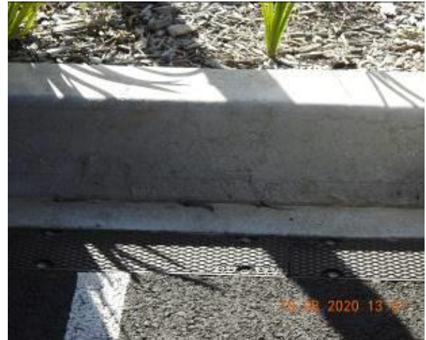
Figure 862 – Hairline cracking through car park kerb
