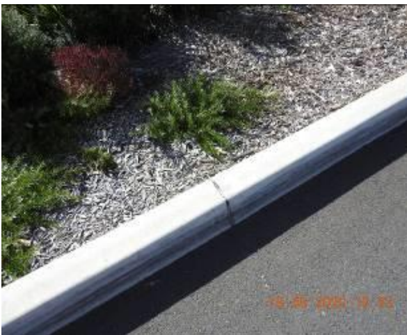
Figure 643 – Crack propagation through car park kerb
