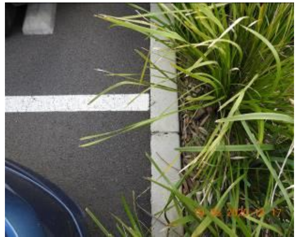
Figure 1062 – Crack propagation through car park kerb
