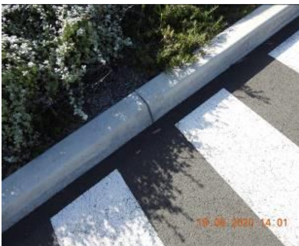
Figure 907 – Crack propagation through car park kerb
