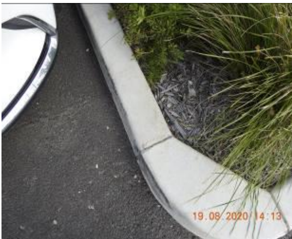
Figure 1015 – Crack propagation through car park kerb
