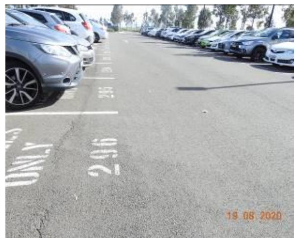
Figure 488 – Evidence of patchwork through car park pavement
