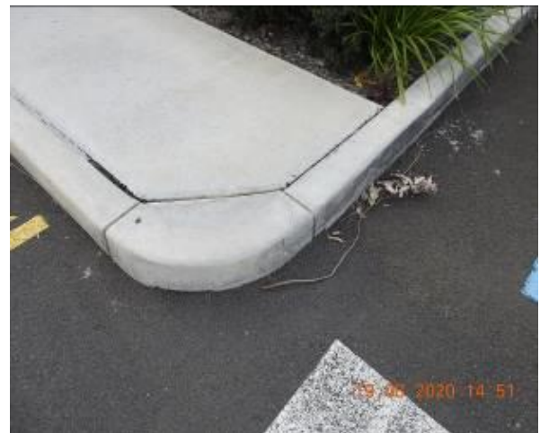
Figure 114 – Crack propagation through car park kerb
