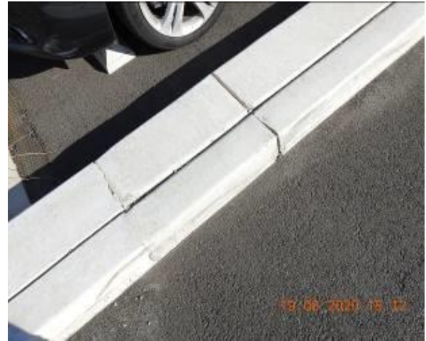
Figure 320 – Crack propagation through car park kerb
