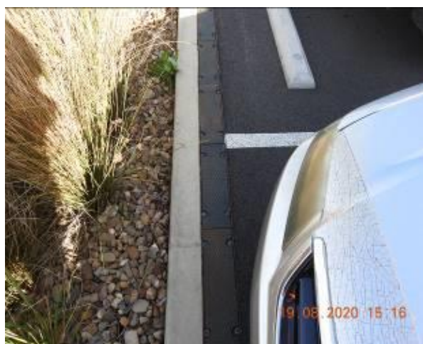
Figure 377 – Crack propagation through car park kerb and service pit
