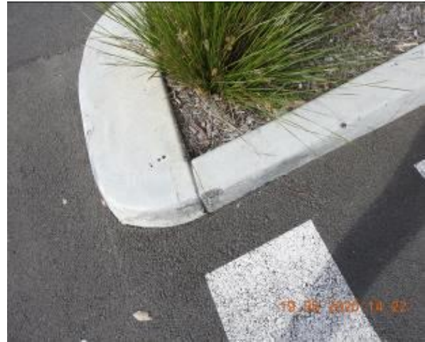
Figure 1126 – Crack propagation through car park kerb
