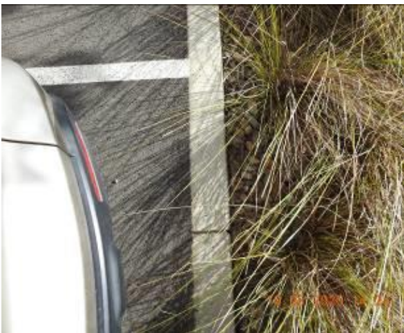
Figure 1159 – Crack propagation through car park kerb
