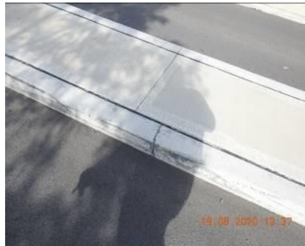
Figure 684 – Crack propagation through traffic island kerb
