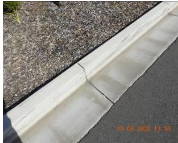
Figure 606 – Crack propagation and loss of material through car park kerb
