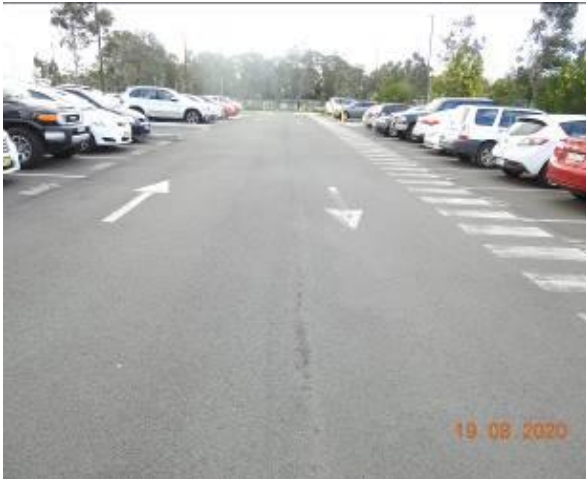
Figure 7 – Loss of material through car park pavement
