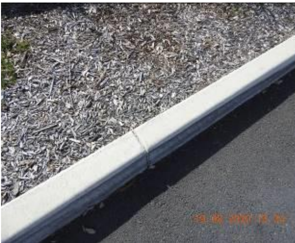
Figure 647 – Crack propagation through car park kerb
