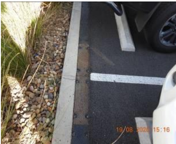
Figure 381 – Crack propagation through car park kerb and service pit
