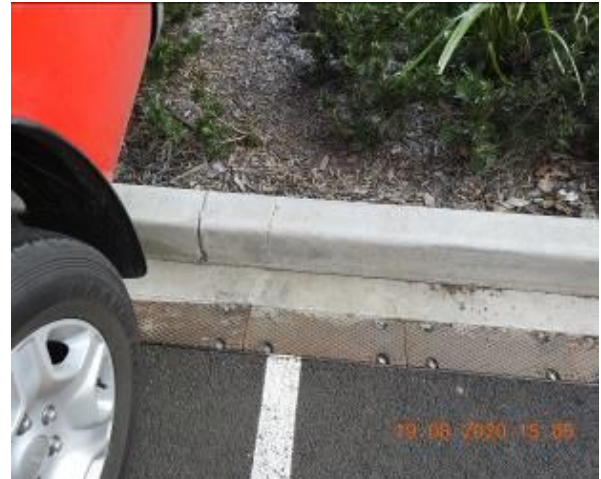
Figure 218 – Crack propagation through car park kerb and gutter
