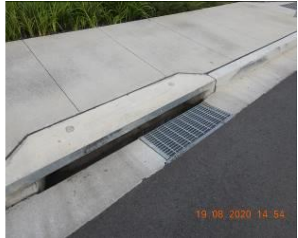
Figure 152 – General condition of kerb inlet pit and stormwater inlet pit
