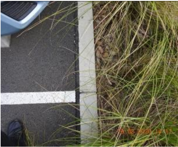
Figure 1055 – Crack propagation through car park kerb
