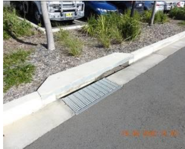
Figure 604 – General condition of kerb inlet pit and stormwater inlet pit
