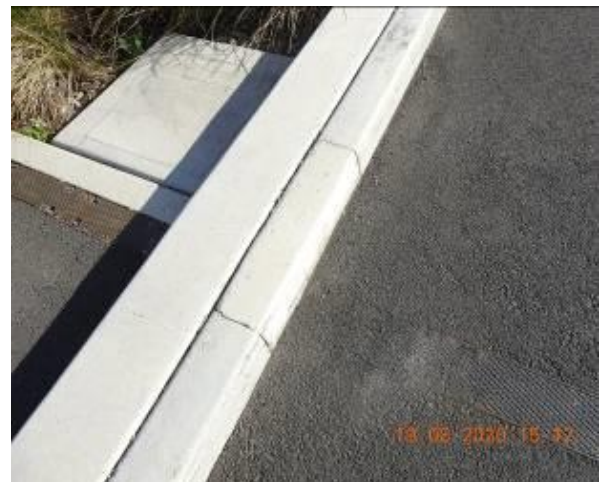
Figure 318 – Crack propagation through car park kerb
