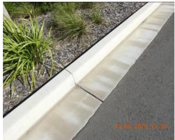
Figure 614 – Crack propagation through car park kerb
