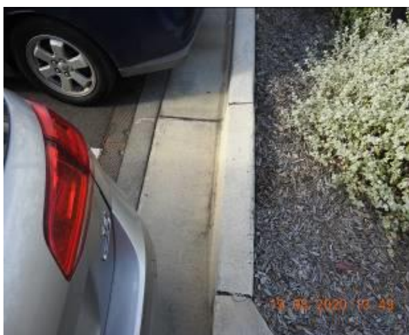
Figure 781 – Crack propagation through car park gutter
