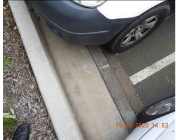
Figure 134 – Crack propagation through car park kerb and gutter
