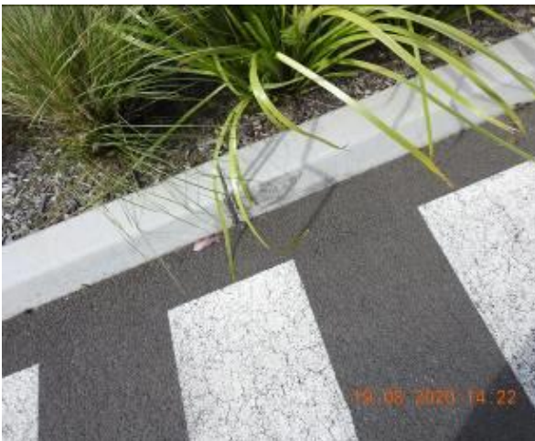
Figure 1127 – Crack propagation through car park kerb
