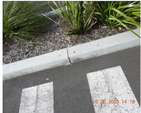
Figure 1044 – Crack propagation through car park kerb
