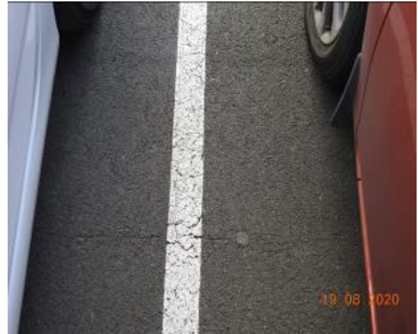
Figure 520 – Crack propagation through car park pavement
