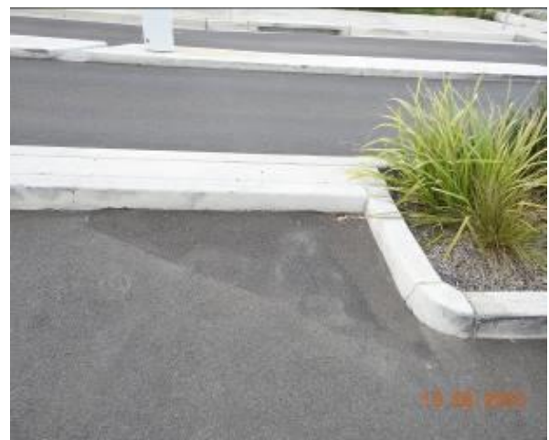
Figure 24 – Evidence of patchwork through car park pavement
