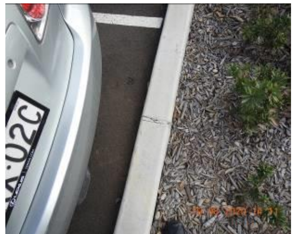
Figure 998 – Crack propagation through car park kerb
