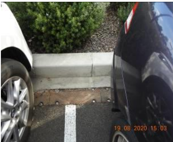
Figure 209 – Crack propagation through car park kerb and gutter
