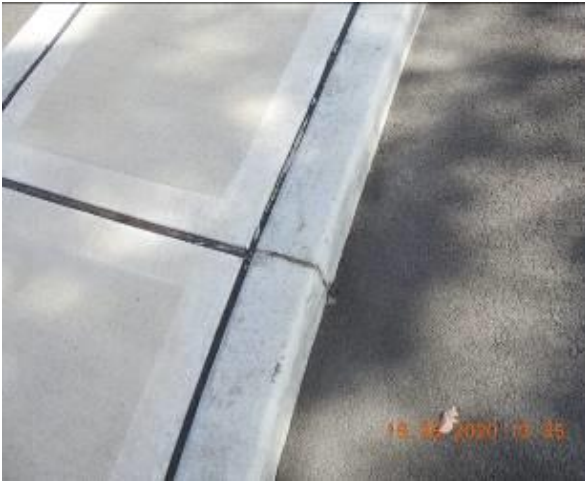
Figure 669 – Crack propagation through traffic island kerb
