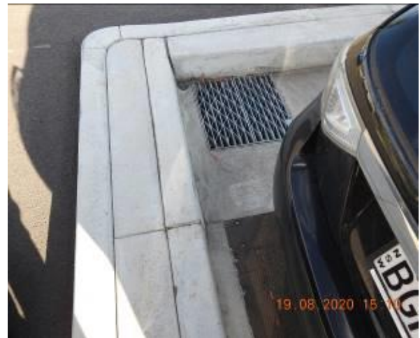
Figure 298 – General condition of car park kerb and stormwater inlet pit
