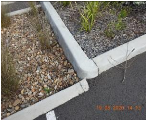
Figure 1019 – Crack propagation through car park kerb
