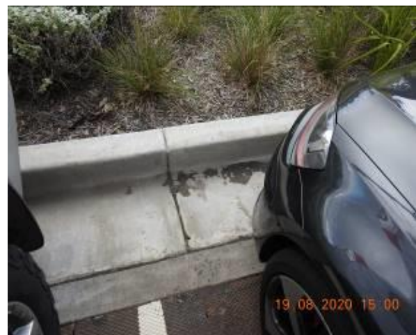
Figure 174 – Hairline cracking through car park kerb and gutter
