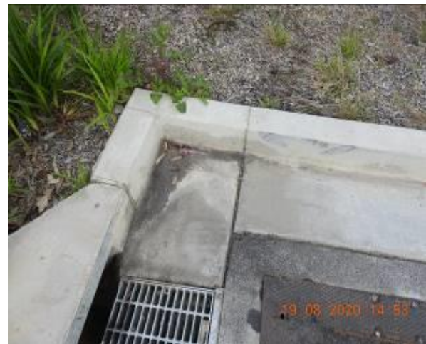
Figure 142 – Crack propagation through car park kerb
