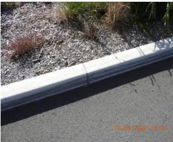
Figure 637 – Crack propagation through car park kerb
