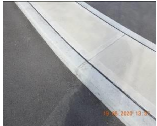
Figure 690 – Crack propagation through traffic island kerb
