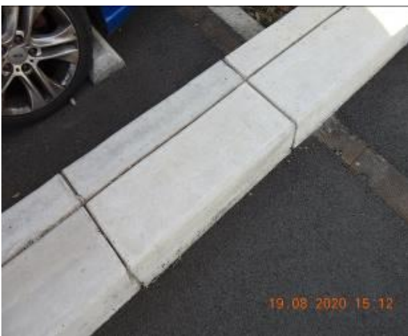
Figure 323 – Crack propagation through car park kerb
