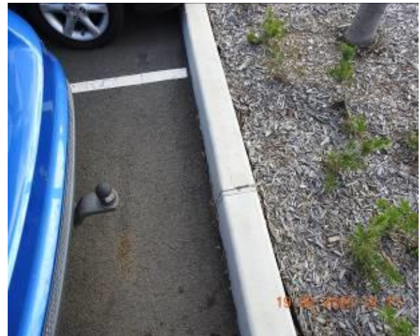
Figure 1002 – Crack propagation through car park kerb
