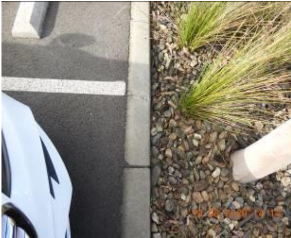
Figure 1029 – Crack propagation through car park kerb
