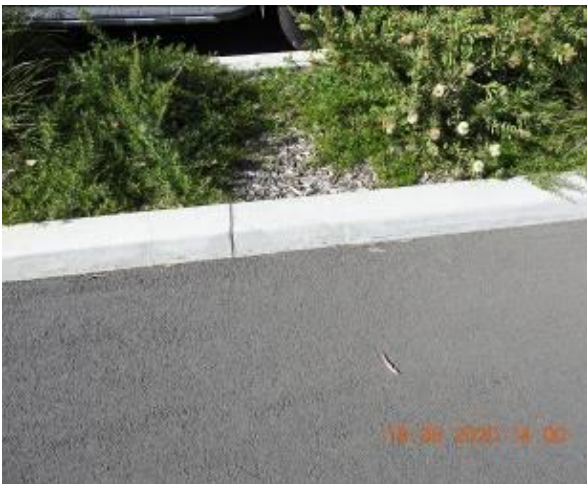
Figure 887 – Crack propagation through car park kerb
