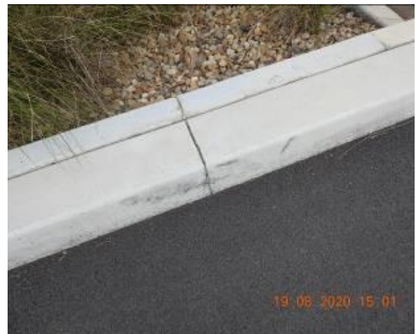
Figure 180 – Crack propagation through car park kerb
