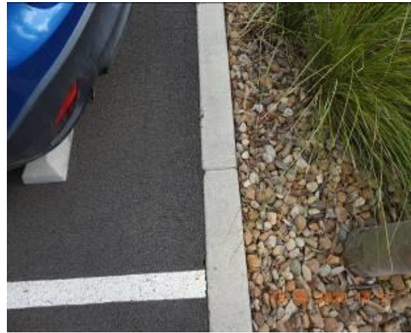
Figure 1056 – Crack propagation through car park kerb
