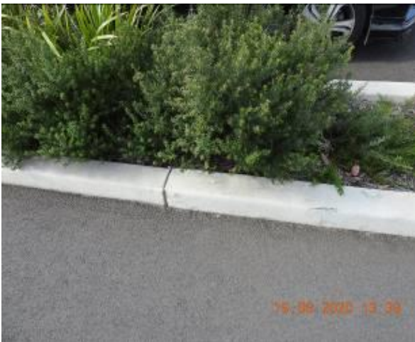
Figure 701 – Crack propagation through car park kerb
