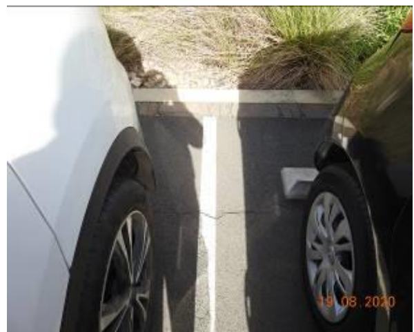
Figure 452 – Crack propagation through car park pavement
