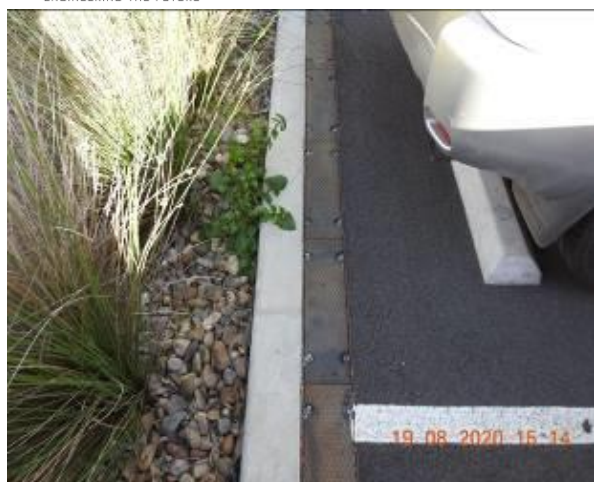
Figure 355 – Evidence of patchwork through car park kerb and service pit
