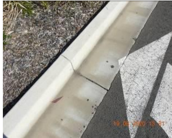
Figure 622 – Crack propagation through car park kerb
