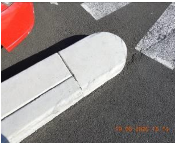
Figure 347 – Crack propagation and loss of material through car park kerb
