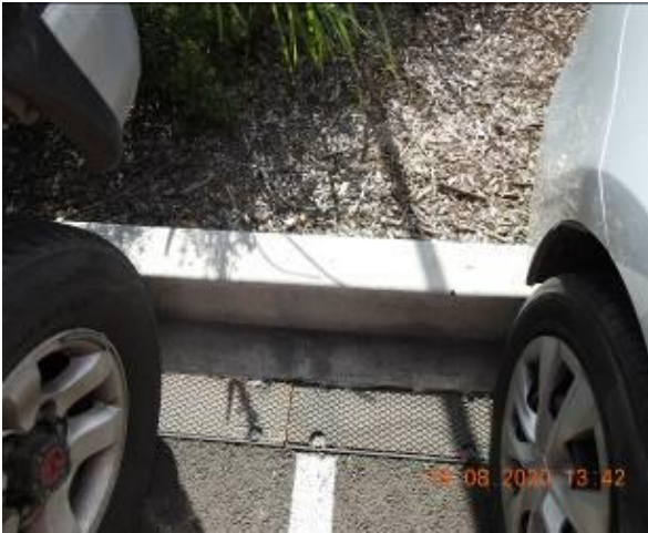
Figure 717 – Crack propagation through car park gutter
