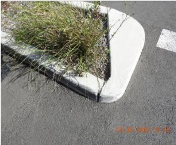
Figure 747 – Loss of material through car park kerb
