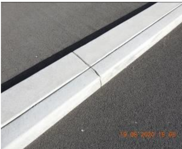
Figure 263 – Crack propagation through car park kerb
