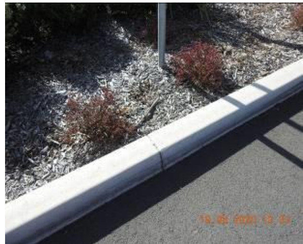
Figure 636 – Crack propagation through car park kerb
