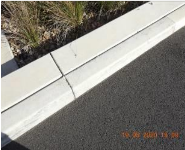
Figure 283 – Crack propagation through car park kerb
