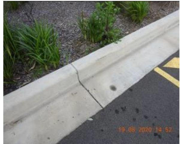
Figure 124 – Crack propagation through car park kerb and gutter
