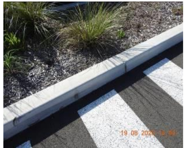
Figure 894 – Crack propagation through car park kerb
