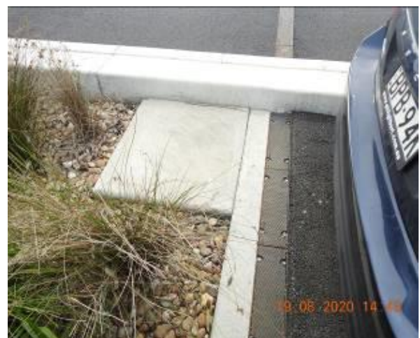
Figure 90 – Crack propagation through car park kerb and general condition of service pit
