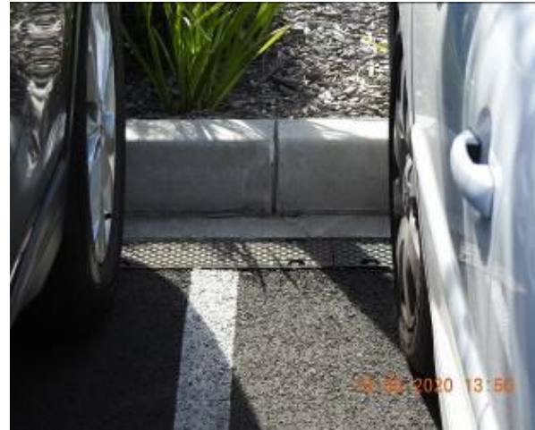
Figure 856 – Crack propagation through car park kerb and gutter
