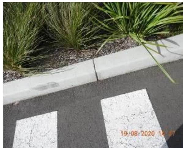
Figure 1196 – Crack propagation through car park kerb
