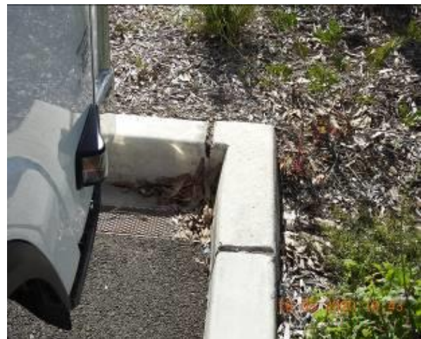
Figure 722 – Crack propagation and loss of material through car park kerb
