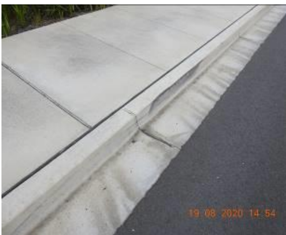
Figure 149 – Hairline cracking through car park kerb
