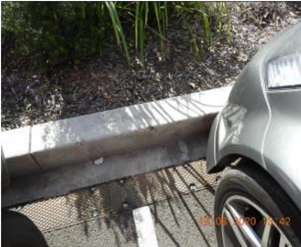
Figure 711 – Crack propagation through car park gutter
