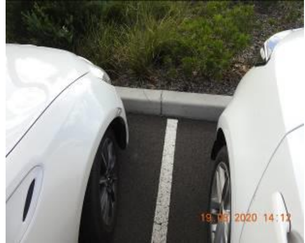
Figure 1006 – Crack propagation through car park kerb
