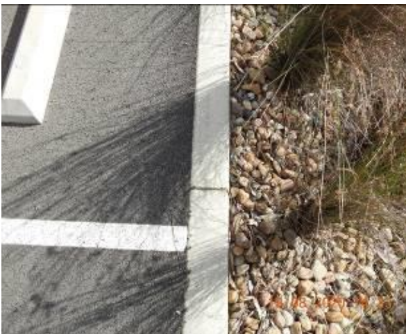
Figure 1147 – Crack propagation through car park kerb
