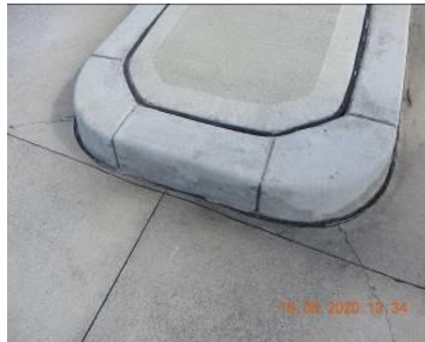
Figure 654 – Hairline cracking through traffic island kerb
