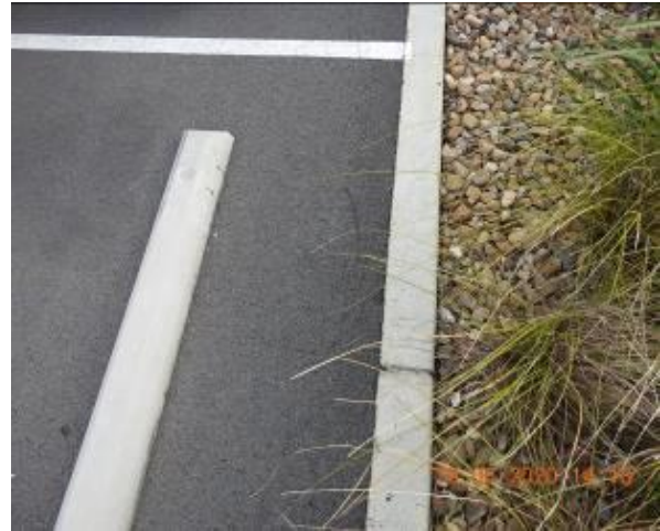
Figure 1072 – Crack propagation through car park kerb
