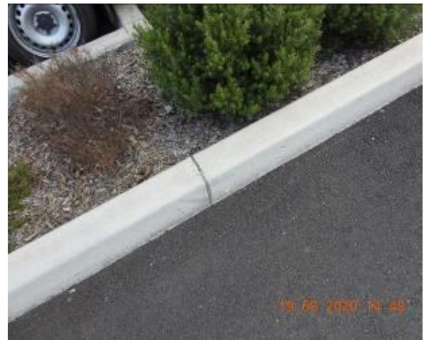
Figure 76 – Crack propagation through car park kerb
