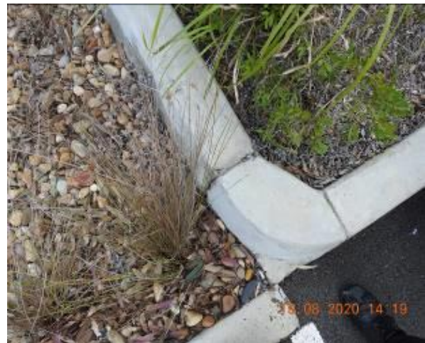
Figure 1092 – Crack propagation through car park kerb
