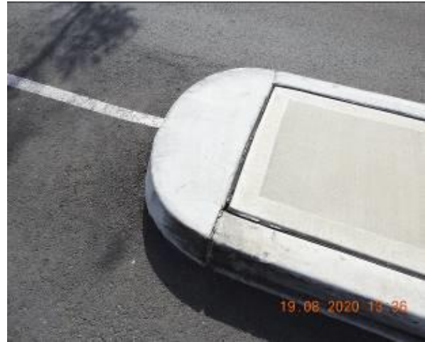
Figure 682 – Crack propagation through traffic island kerb
