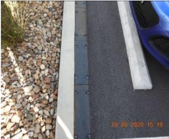
Figure 379 – Hairline cracking through car park kerb and service pit
