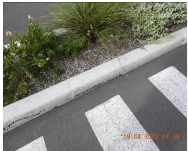
Figure 1046 – Crack propagation through car park kerb
