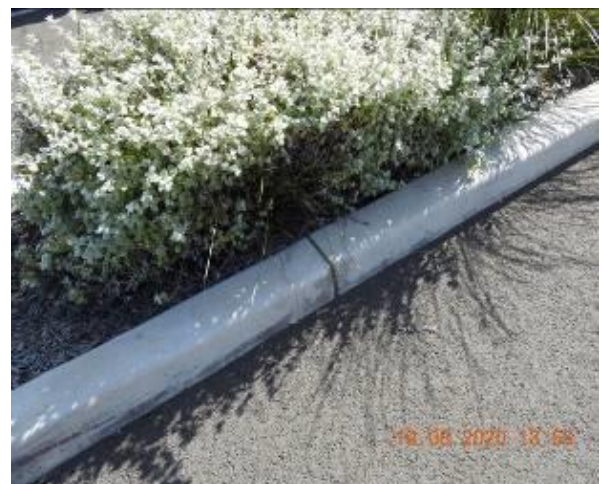
Figure 836 – Crack propagation through car park kerb
