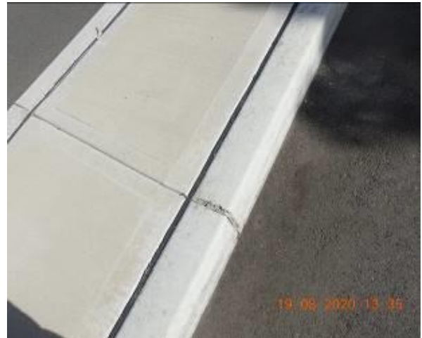
Figure 666 – Loss of material through traffic island kerb
