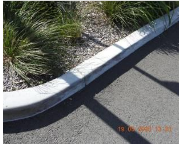
Figure 628 – Crack propagation through car park kerb
