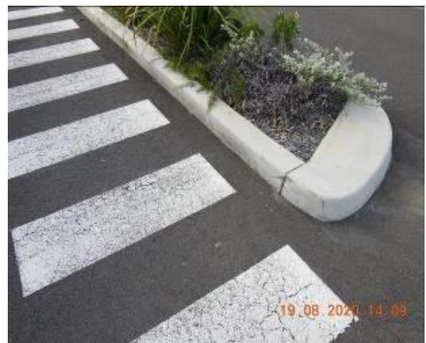
Figure 986 – Hairline cracking through car park kerb
