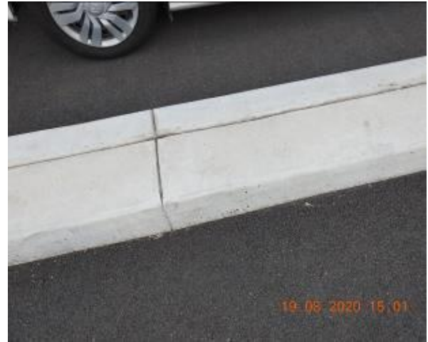
Figure 182 – Crack propagation through car park kerb
