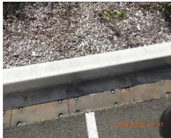
Figure 710 – Crack propagation through car park kerb
