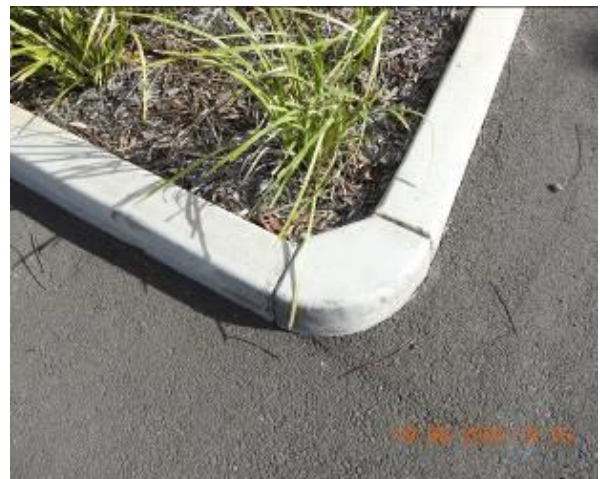
Figure 1172 – Crack propagation through car park kerb
