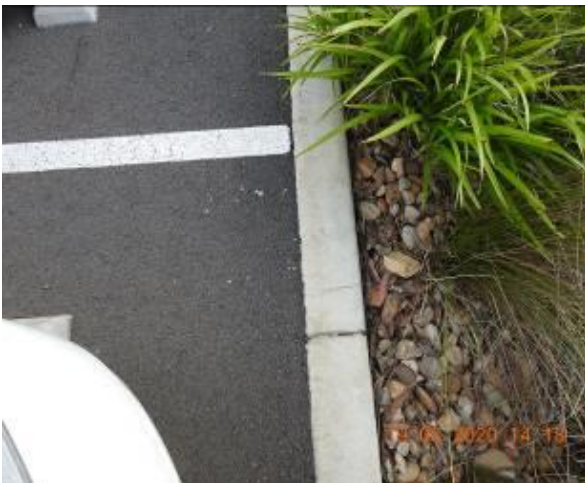
Figure 1079 – Crack propagation through car park kerb
