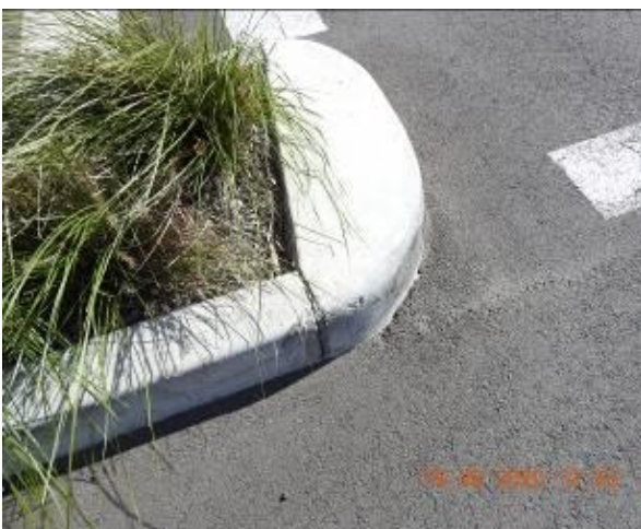
Figure 841 – Crack propagation through car park kerb
