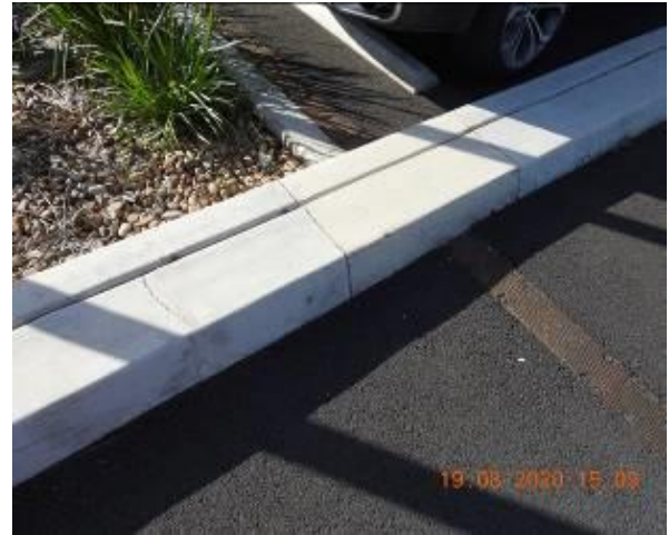
Figure 278 – Crack propagation through car park kerb
