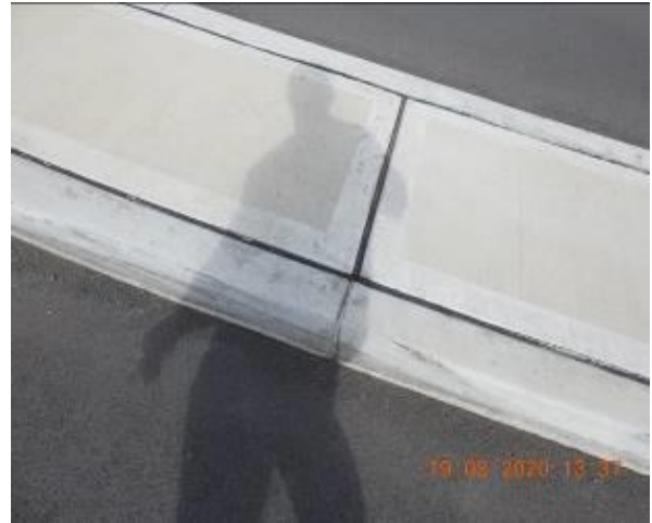
Figure 688 – Crack propagation through traffic island kerb
