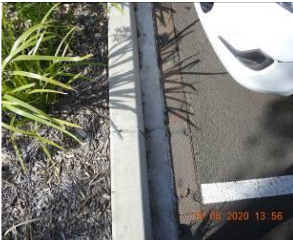
Figure 851 – Crack propagation through car park gutter
