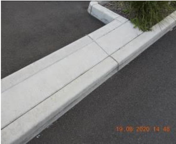
Figure 73 – Hairline cracking through car park kerb
