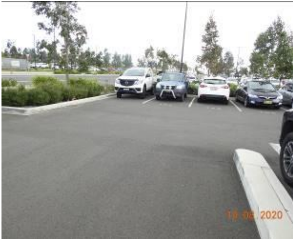
Figure 31 – General condition of car park pavement
