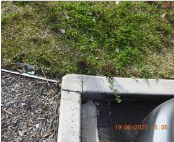
Figure 229 – Loss of material through car park kerb
