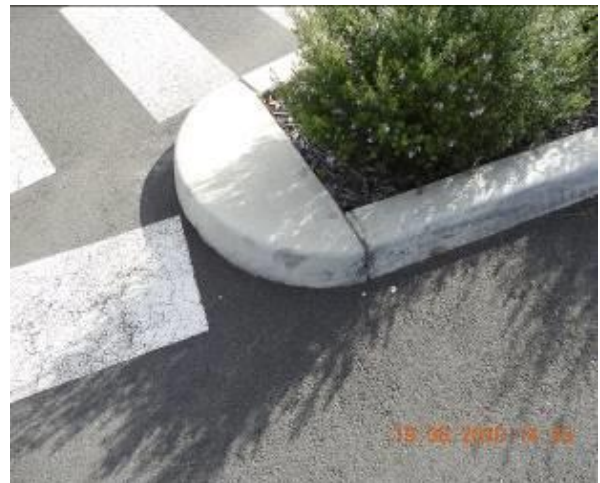
Figure 1170 – Crack propagation through car park kerb
