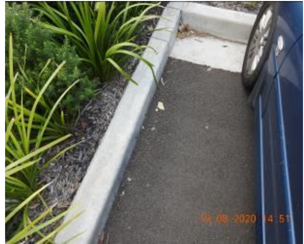
Figure 116 – Hairline cracking through car park kerb
