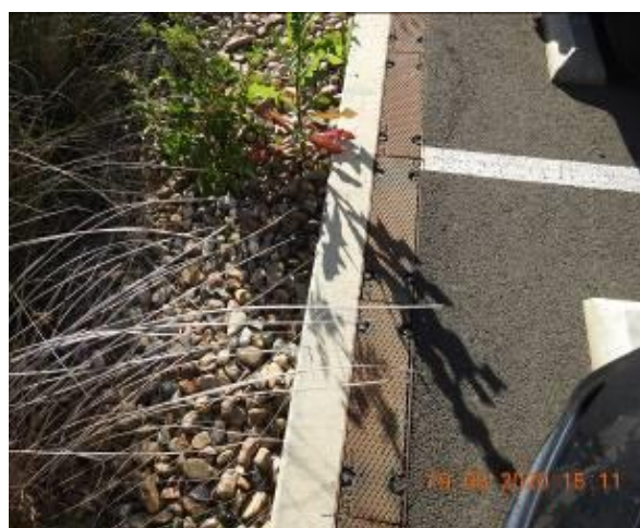
Figure 306 – Evidence of patchwork through car park kerb and General condition of service pit
