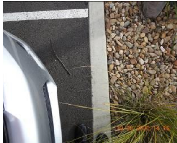
Figure 1050 – Crack propagation through car park kerb
