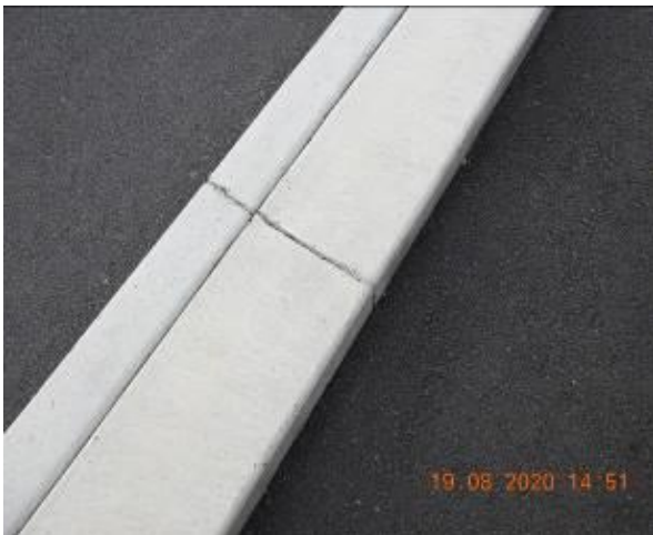
Figure 111 – Crack propagation through car park kerb
