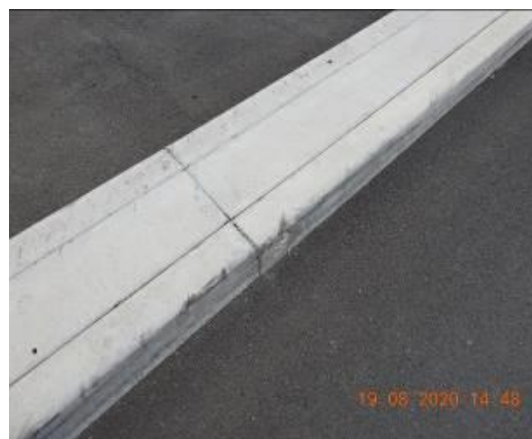
Figure 72 – Crack propagation through car park kerb
