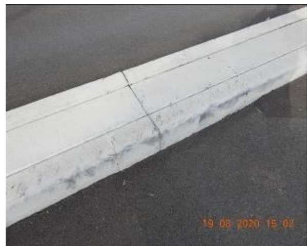
Figure 198 – Crack propagation through car park kerb
