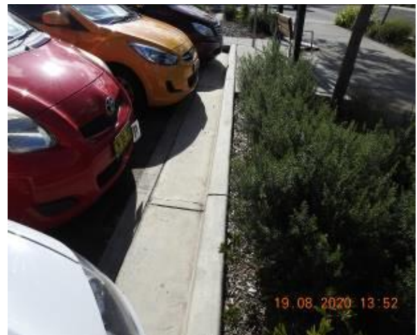
Figure 806 – Crack propagation through car park kerb and gutter
