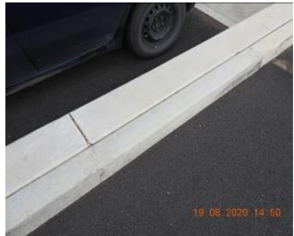
Figure 94 – Hairline cracking through car park kerb
