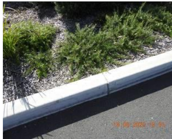
Figure 642 – Crack propagation through car park kerb
