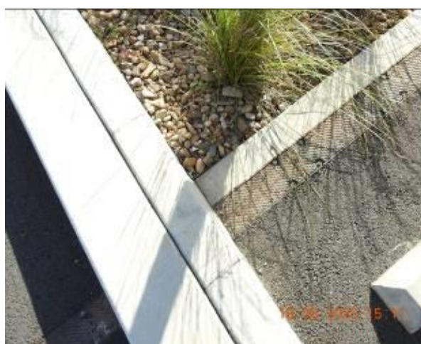
Figure 303 – Crack propagation through car park kerb
