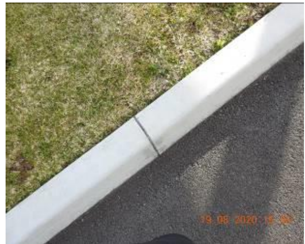
Figure 232 – Crack propagation through car park kerb
