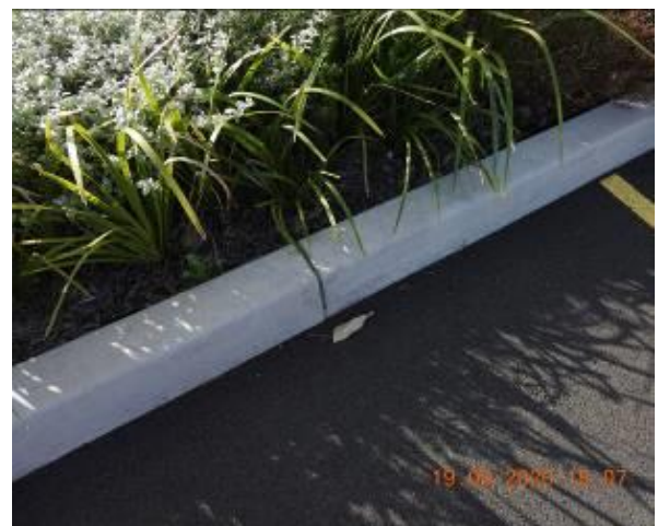
Figure 246 – Crack propagation through car park kerb
