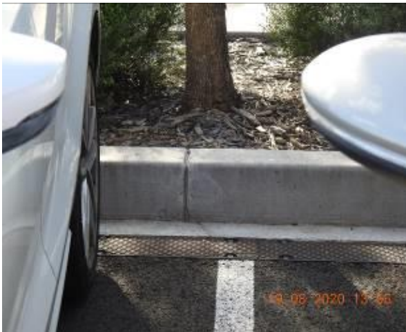
Figure 857 – Crack propagation through car park kerb and gutter
