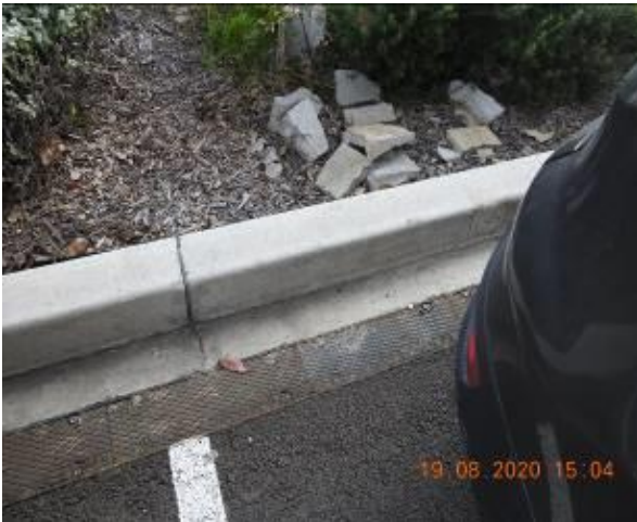
Figure 213 – Crack propagation through car park gutter
