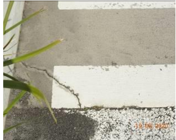
Figure 574 – Crack propagation through car park pavement
