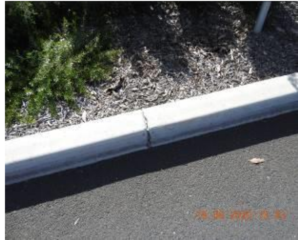
Figure 640 – Crack propagation through car park kerb
