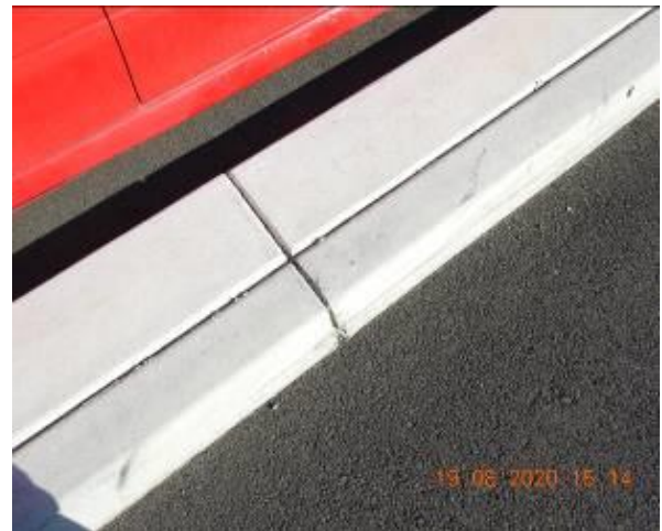
Figure 346 – Crack propagation through car park kerb
