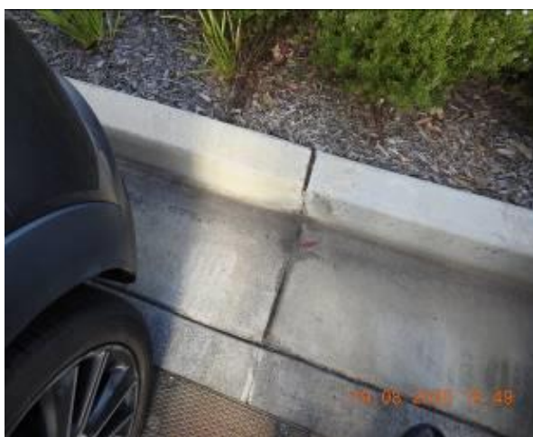
Figure 779 – Crack propagation through car park gutter
