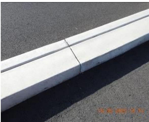
Figure 341 – Crack propagation through car park kerb
