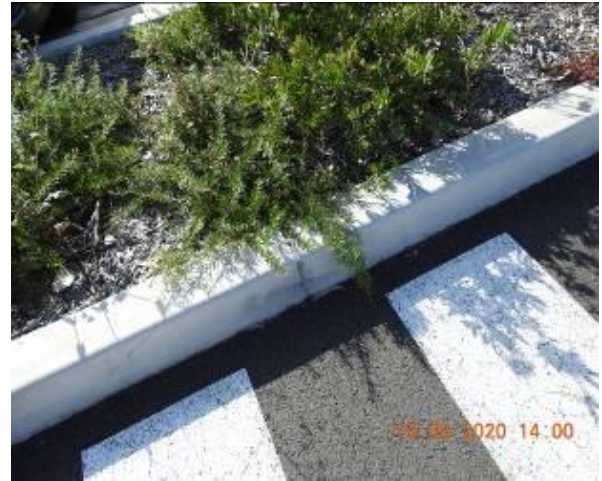
Figure 892 – Crack propagation through car park kerb
