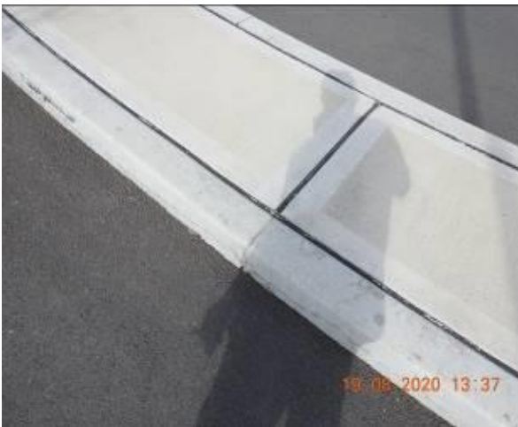
Figure 689 – Crack propagation through traffic island kerb
