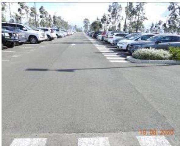
Figure 463 – Evidence of patchwork through car park pavement
