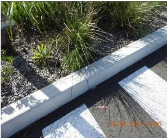
Figure 893 – Crack propagation through car park kerb
