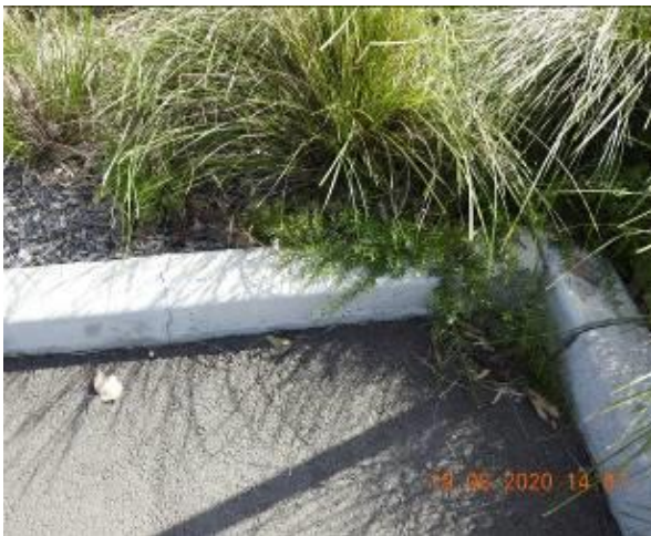
Figure 965 – Crack propagation through car park kerb
