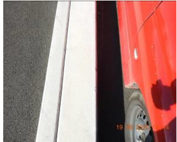
Figure 350 – Loss of material through car park kerb
