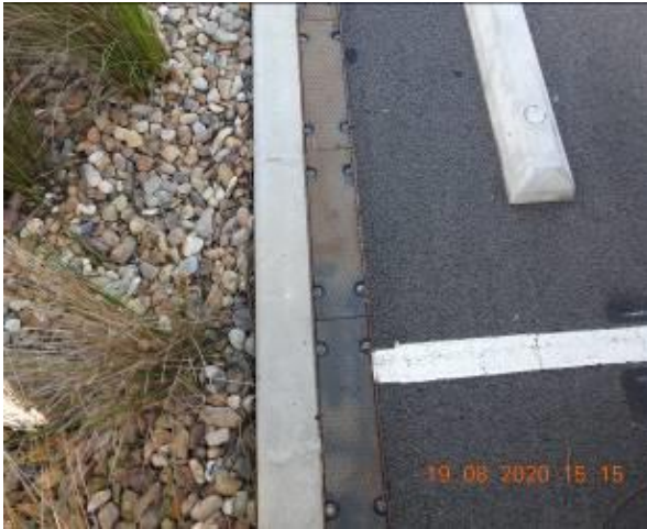
Figure 361 – Evidence of patchwork through car park kerb and service pit
