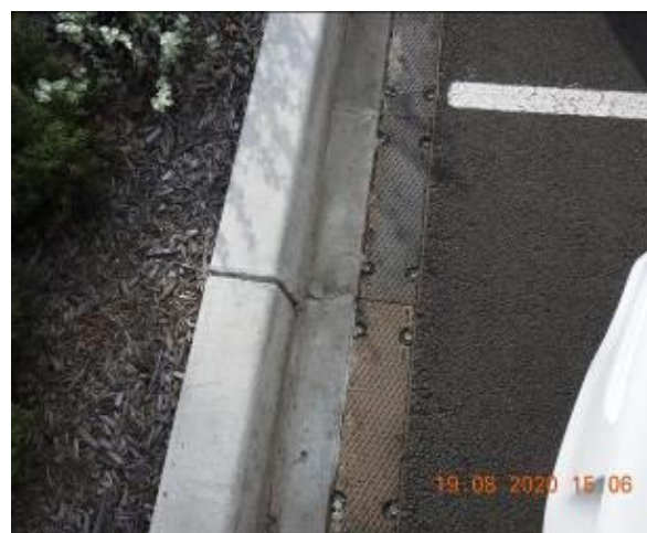
Figure 228 – Crack propagation through car park kerb and gutter
