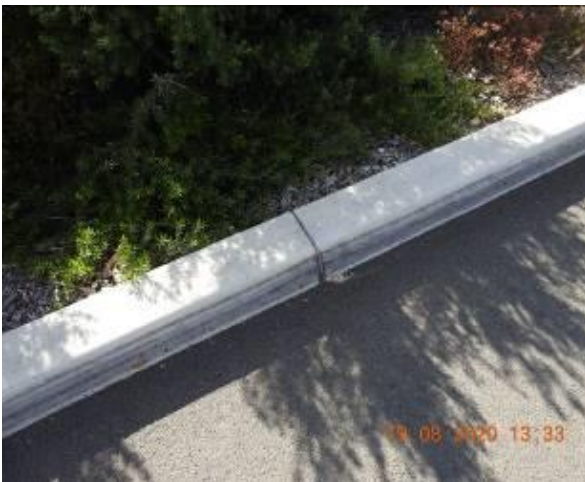
Figure 635 – Crack propagation through car park kerb
