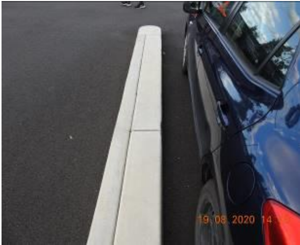
Figure 91 – Crack propagation through car park kerb
