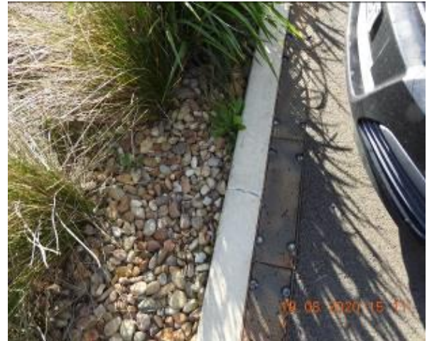
Figure 308 – Crack propagation through car park kerb and service pit
