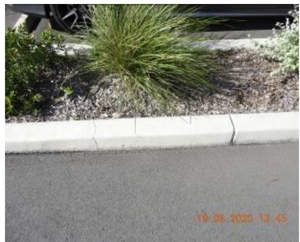
Figure 752 – Crack propagation through car park kerb
