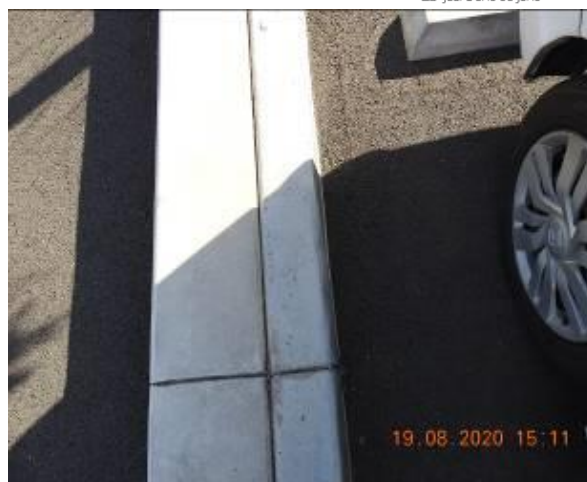
Figure 302 – Crack propagation through car park kerb
