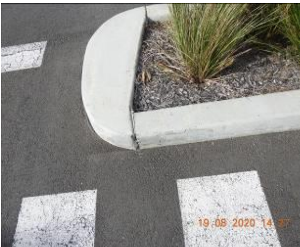
Figure 1195 – Crack propagation and loss of material through car park kerb
