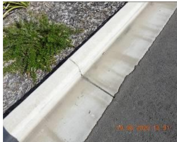
Figure 624 – Crack propagation through car park kerb
