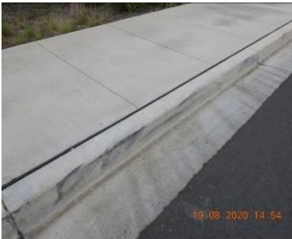
Figure 147 – Hairline cracking through car park kerb
