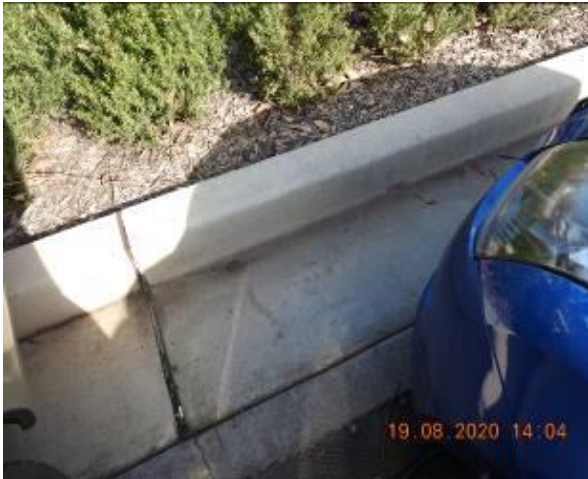
Figure 933 – Crack propagation through car park gutter
