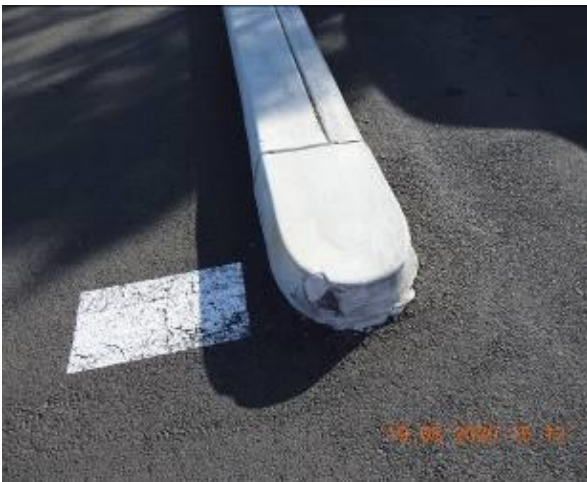
Figure 327 – Loss of material through car park kerb
