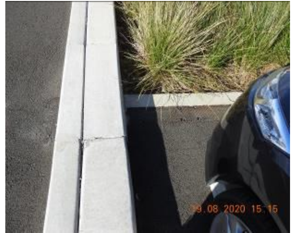
Figure 368 – Crack propagation through car park kerb
