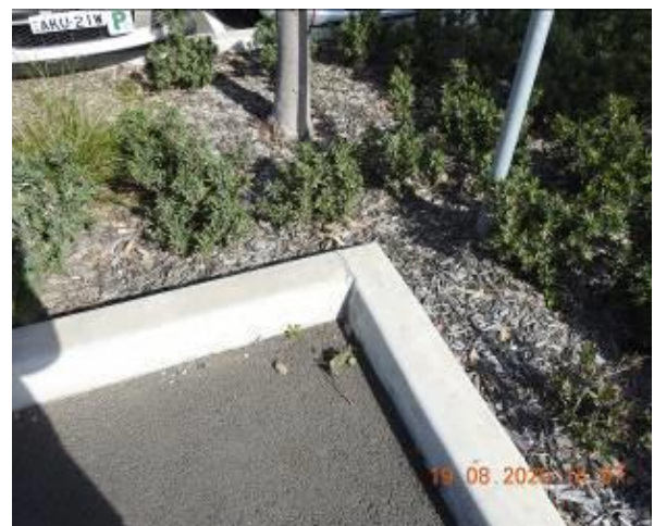
Figure 968 – Crack propagation through car park kerb
