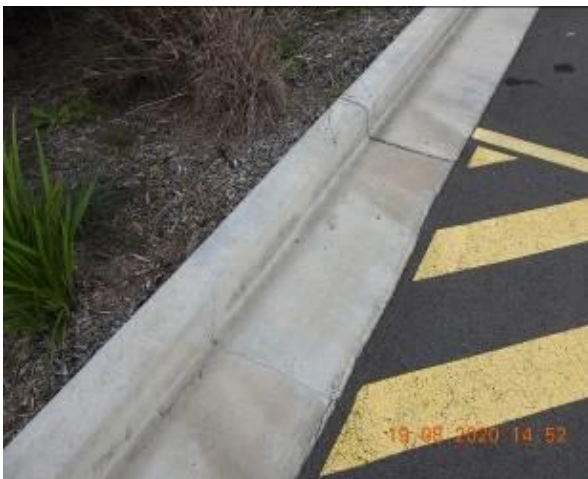
Figure 125 – Crack propagation through car park kerb and gutter
