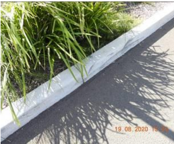
Figure 629 – Crack propagation through car park kerb
