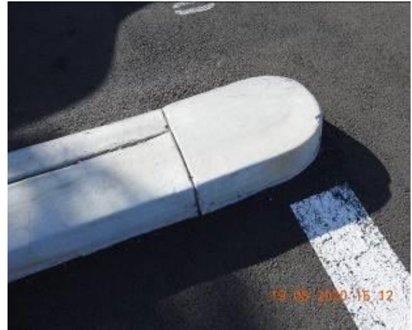
Figure 326 – Hairline cracking through car park kerb
