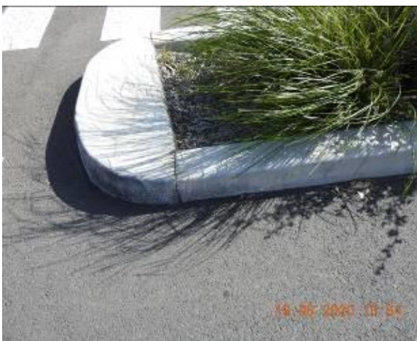
Figure 829 – Crack propagation through car park kerb
