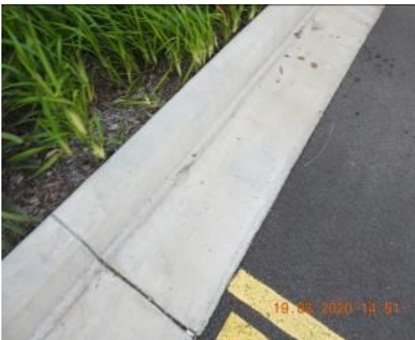
Figure 119 – Crack propagation through car park kerb and gutter
