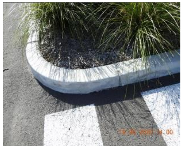
Figure 890 – Hairline cracking through car park kerb
