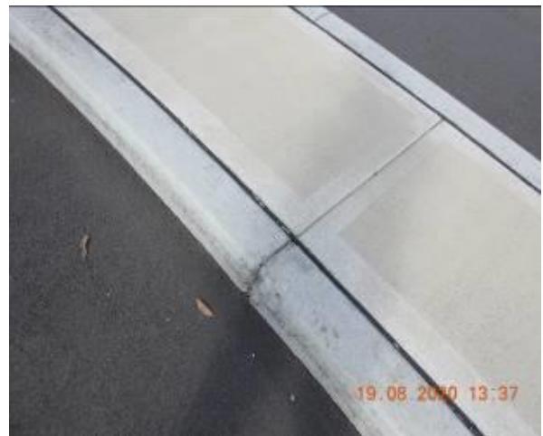
Figure 692 – Crack propagation through traffic island kerb
