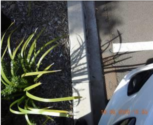
Figure 849 – Crack propagation through car park kerb
