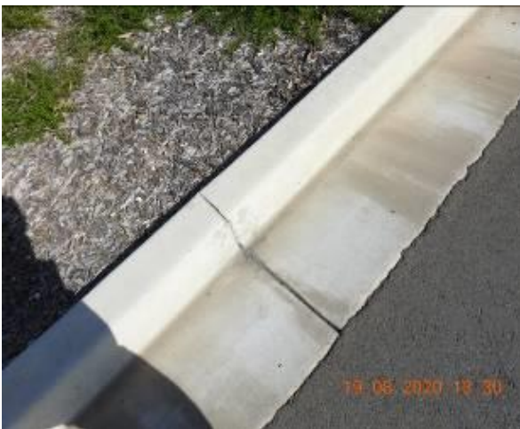
Figure 613 – Crack propagation through car park kerb
