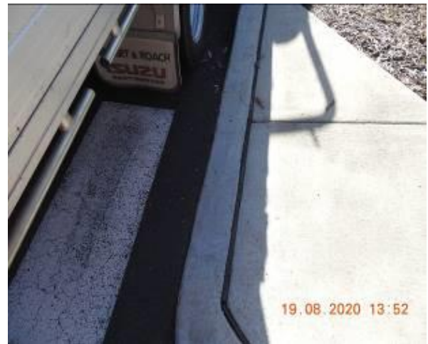
Figure 816 – Crack propagation through car park kerb
