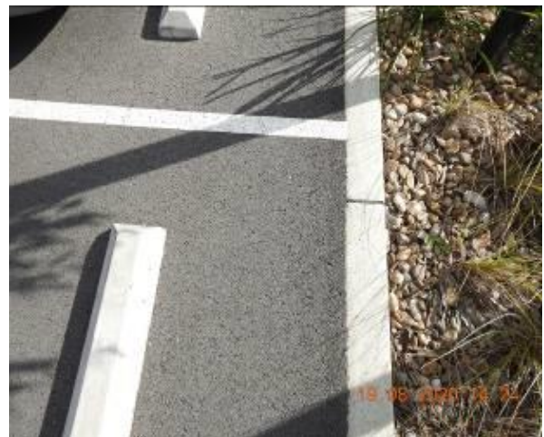
Figure 1160 – Crack propagation through car park kerb
