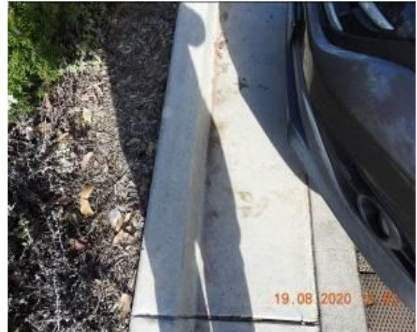
Figure 922 – Crack propagation through car park gutter
