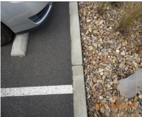
Figure 1099 – Crack propagation through car park kerb
