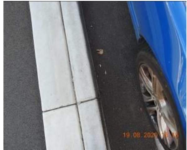
Figure 364 – Crack propagation through car park kerb
