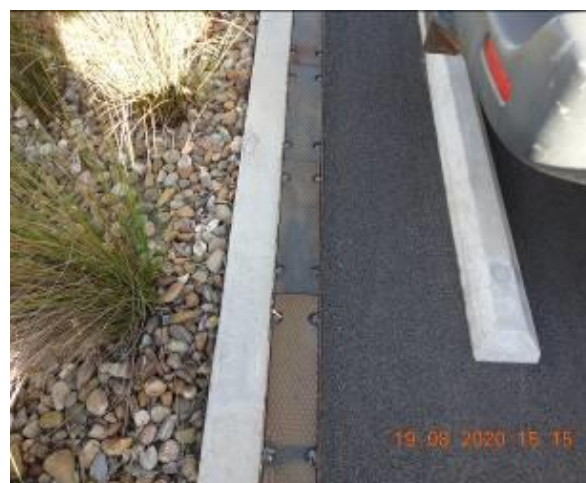
Figure 360 – Crack propagation through car park kerb and service pit
