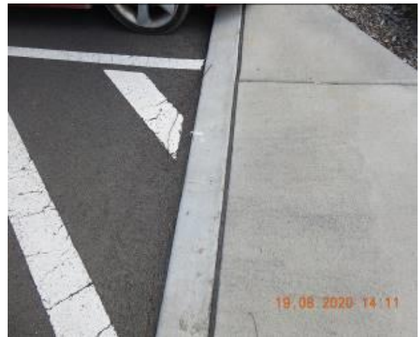
Figure 996 – Crack propagation through car park layback
