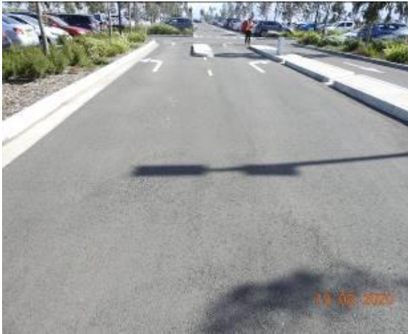
Figure 435 – Loss of material through car park pavement
