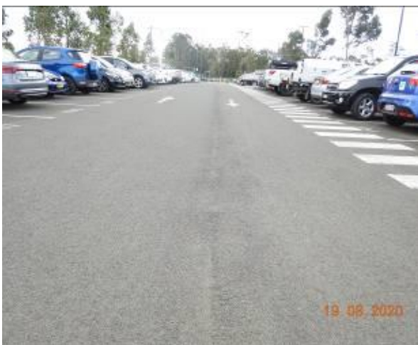
Figure 33 – Loss of material through car park pavement
