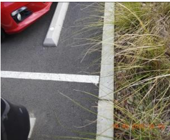
Figure 1081 – Crack propagation through car park kerb
