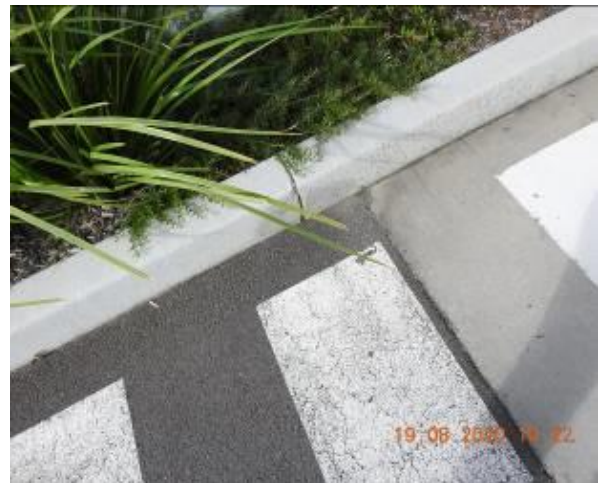
Figure 1128 – Crack propagation through car park kerb
