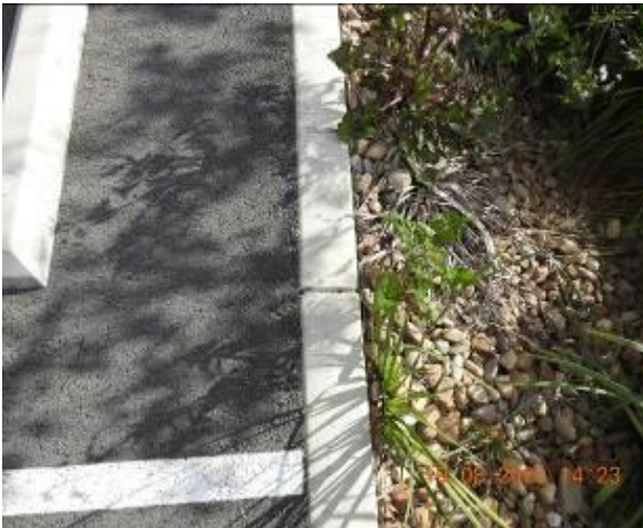
Figure 1139 – Crack propagation through car park kerb
