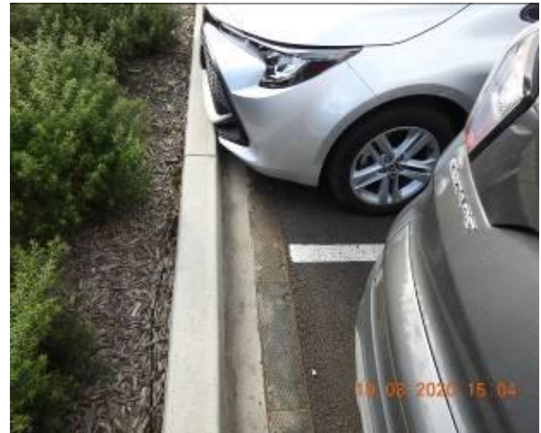
Figure 214 – Crack propagation through car park gutter
