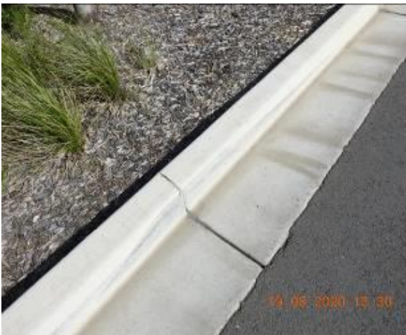
Figure 611 – Crack propagation through car park kerb
