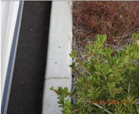
Figure 1017 – Hairline cracking through car park kerb
