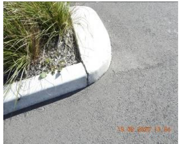
Figure 834 – Crack propagation through car park kerb
