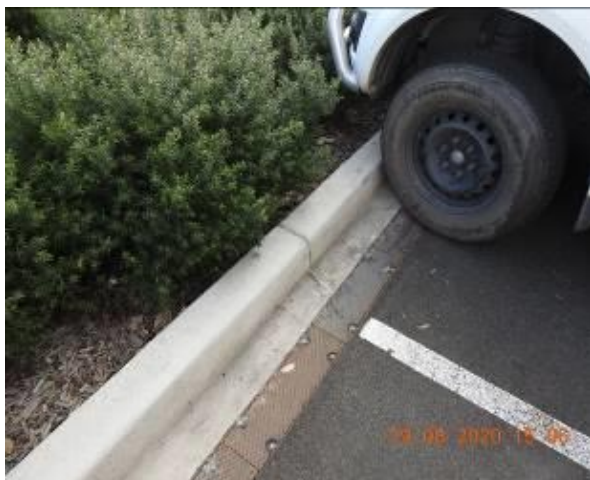
Figure 223 – Crack propagation through car park kerb and gutter
