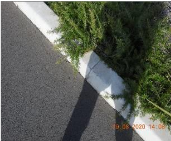
Figure 971 – Crack propagation through car park kerb
