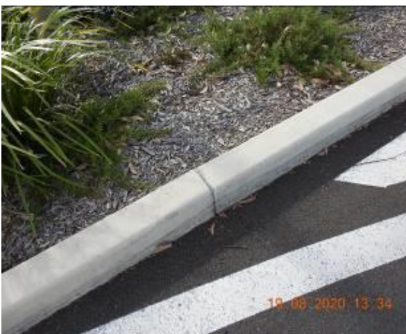
Figure 649 – Crack propagation through car park kerb
