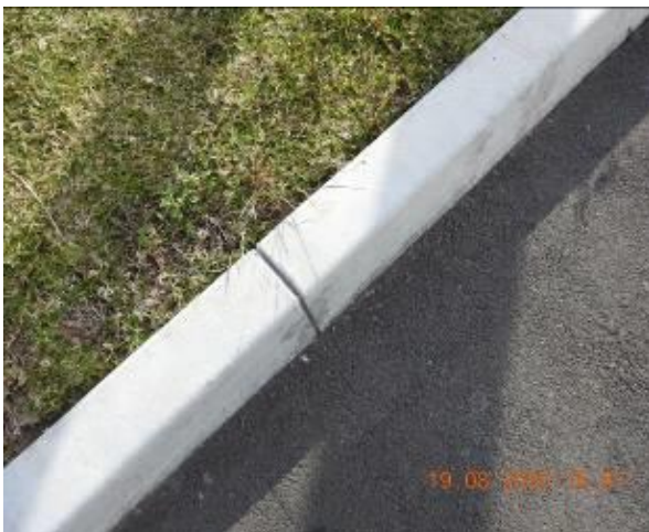
Figure 233 – Crack propagation through car park kerb
