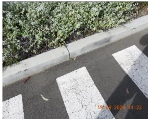
Figure 1130 – Crack propagation through car park kerb
