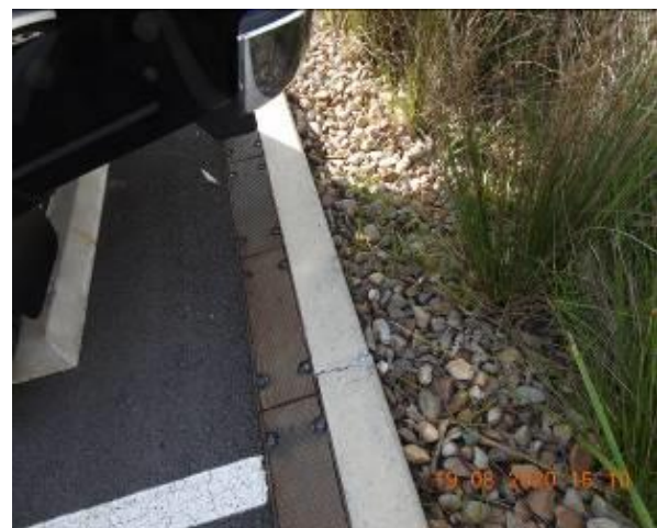
Figure 288 – Crack propagation through car park kerb and service pit
