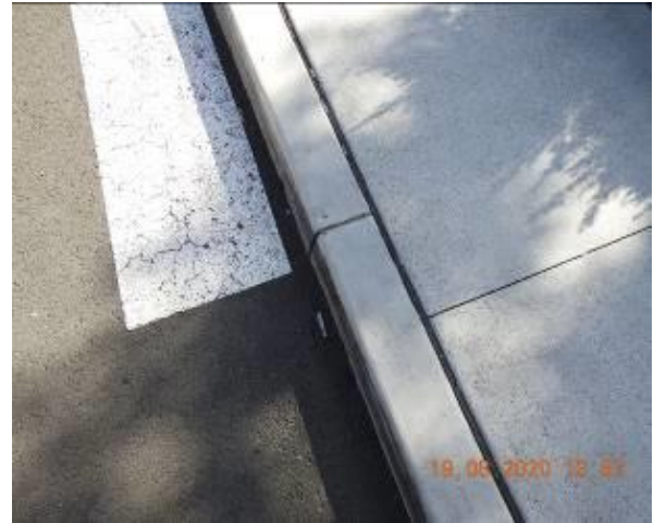
Figure 814 – Crack propagation through car park kerb
