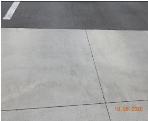
Figure 3 – Crack propagation through car park pavement
