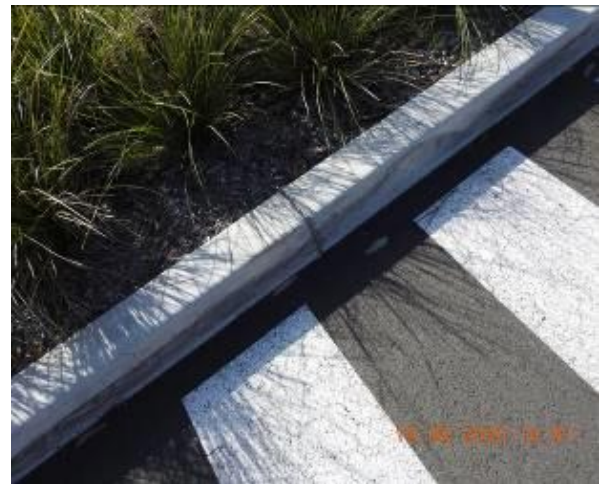
Figure 906 – Crack propagation through car park kerb
