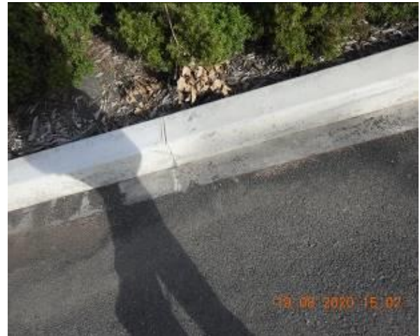
Figure 202 – Crack propagation through gutter
