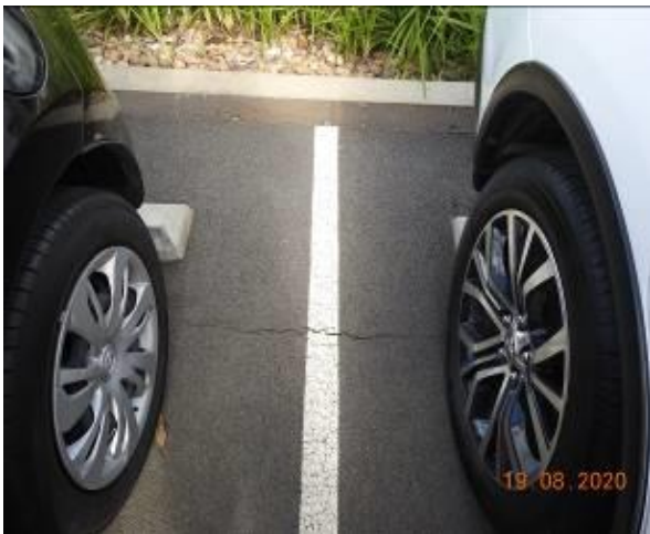
Figure 455 – Crack propagation through car park pavement
