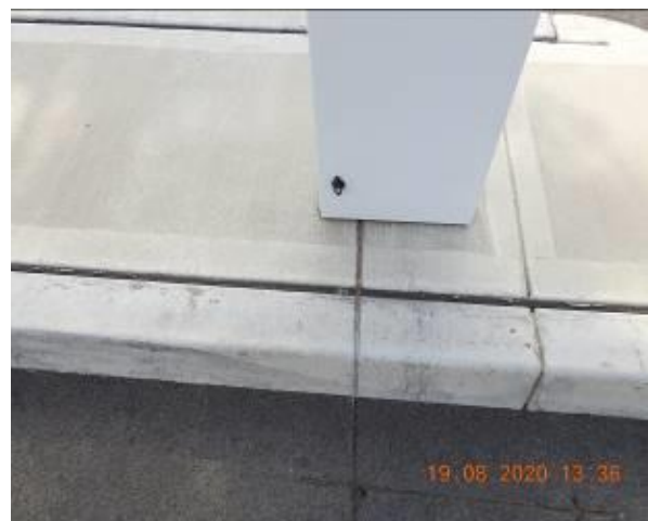
Figure 680 – Crack propagation through traffic island kerb
