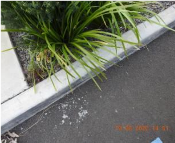
Figure 115 – Hairline cracking through car park kerb
