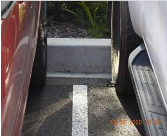
Figure 861 – Hairline cracking through car park kerb
