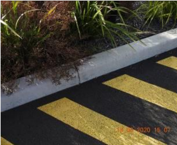
Figure 247 – Crack propagation through car park kerb
