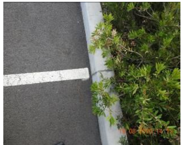
Figure 1010 – Crack propagation through car park kerb
