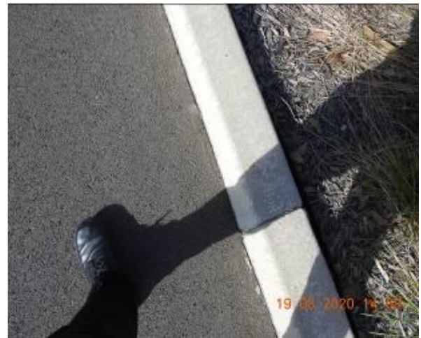
Figure 978 – Crack propagation through car park kerb
