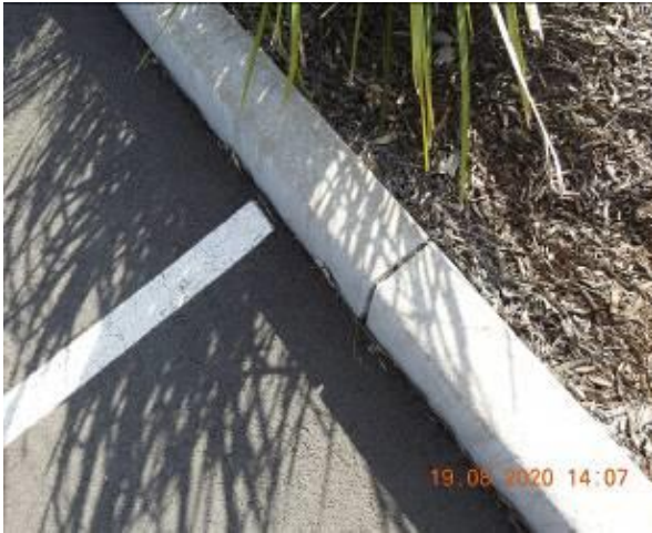
Figure 963 – Crack propagation through car park kerb
