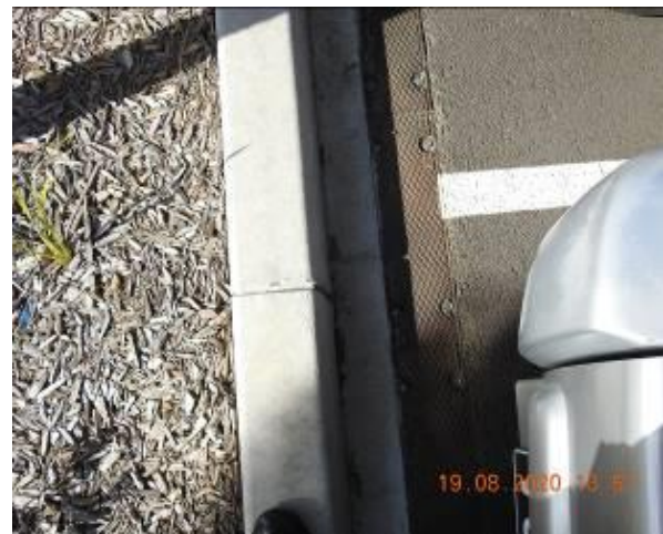
Figure 860 – Crack propagation through car park gutter
