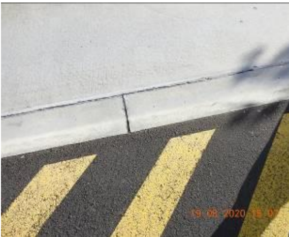
Figure 255 – Crack propagation through car park kerb
