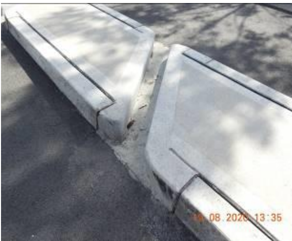
Figure 661 – Crack propagation through traffic island kerb
