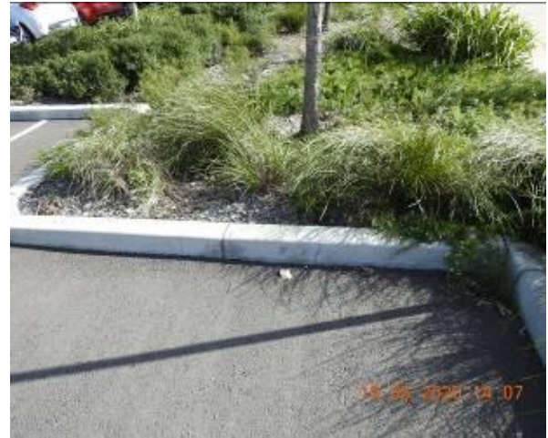
Figure 964 – Crack propagation through car park kerb
