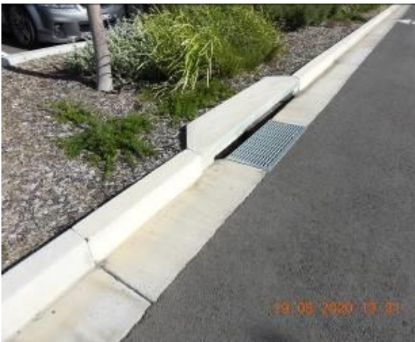
Figure 617 – Crack propagation through car park kerb and general condition of stormwater inlet pit
