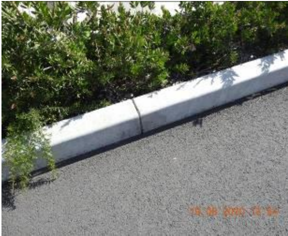
Figure 831 – Crack propagation through car park kerb
