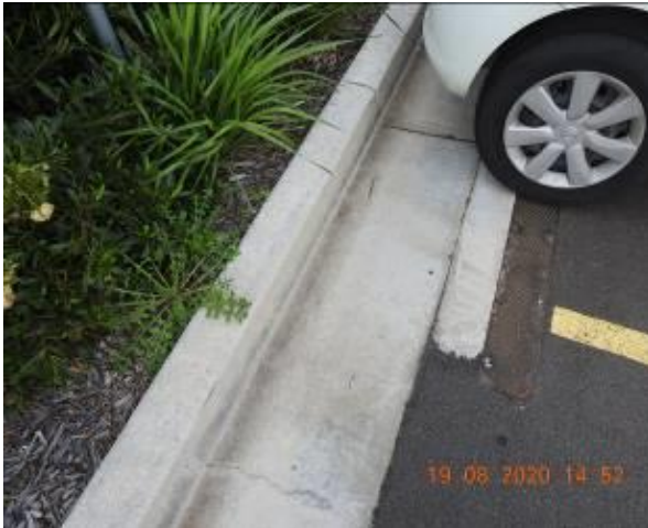
Figure 127 – Crack propagation through car park kerb and gutter
