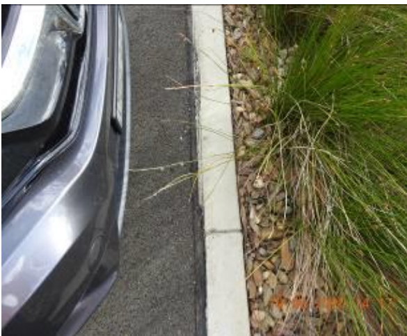
Figure 1051 – Crack propagation through car park kerb
