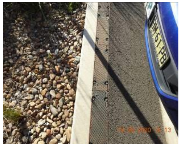
Figure 336 – Crack propagation through car park kerb and service pit
