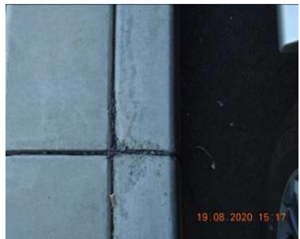
Figure 384 – Crack propagation through car park kerb
