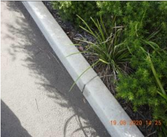
Figure 1173 – Crack propagation through car park kerb
