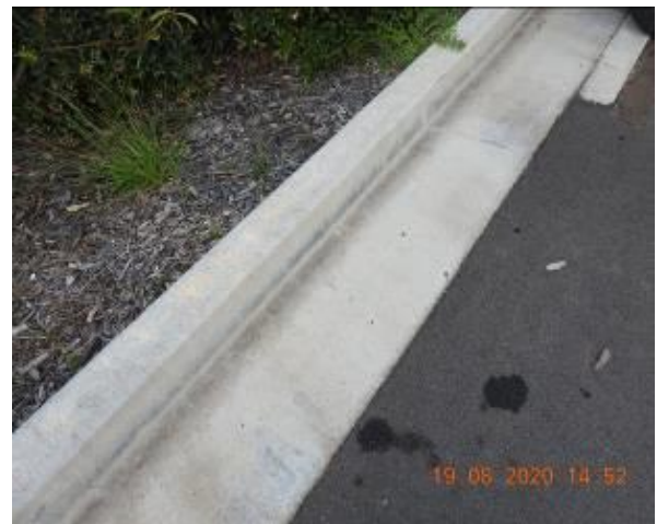
Figure 126 – Hairline cracking through car park kerb and gutter
