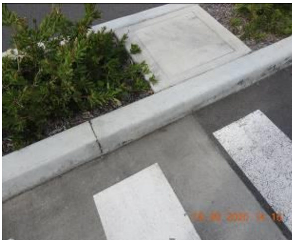
Figure 1045 – Crack propagation through car park kerb and general condition of service pit
