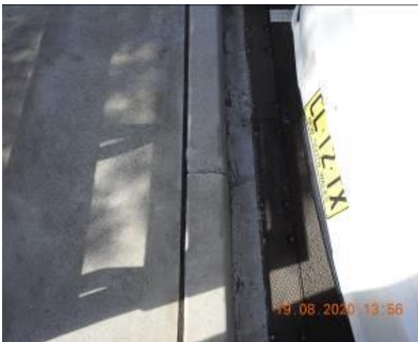
Figure 853 – Crack propagation through car park kerb and gutter
