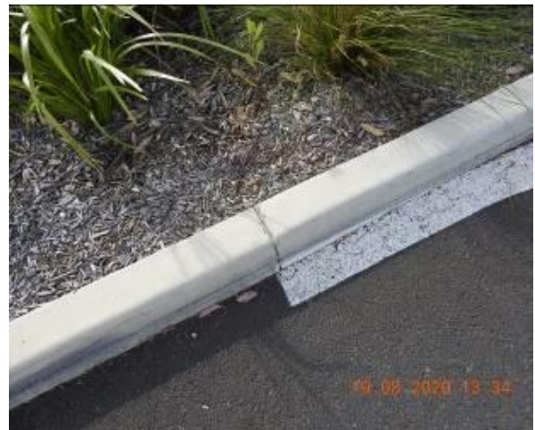
Figure 648 – Crack propagation through car park kerb
