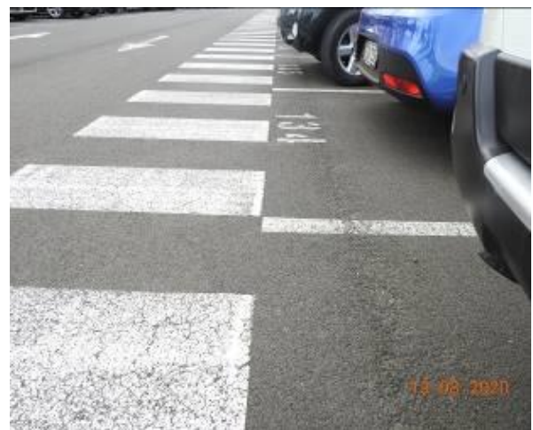
Figure 34 – Loss of material through car park pavement
