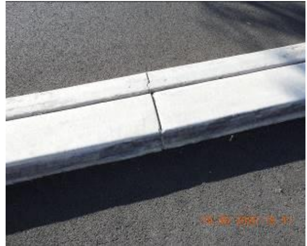
Figure 314 – Crack propagation through car park kerb
