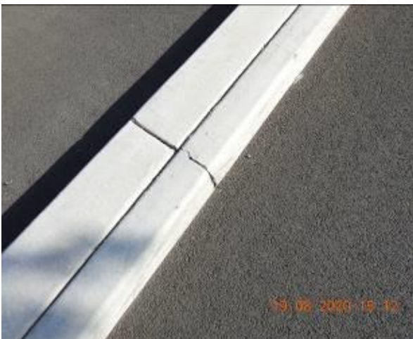
Figure 317 – Crack propagation through car park kerb
