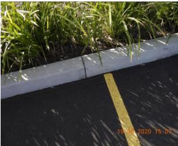
Figure 249 – Crack propagation through car park kerb
