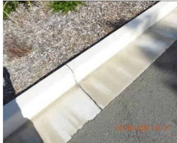
Figure 616 – Crack propagation through car park kerb
