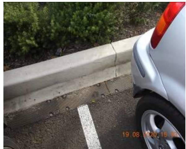
Figure 210 – Crack propagation through car park gutter
