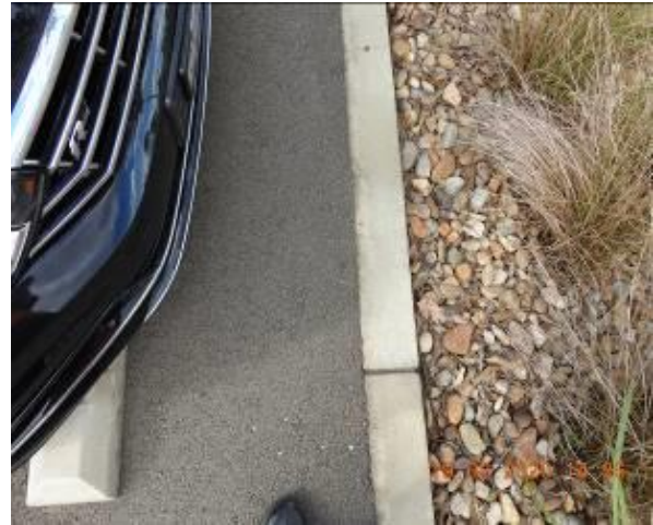
Figure 1180 – Crack propagation through car park kerb
