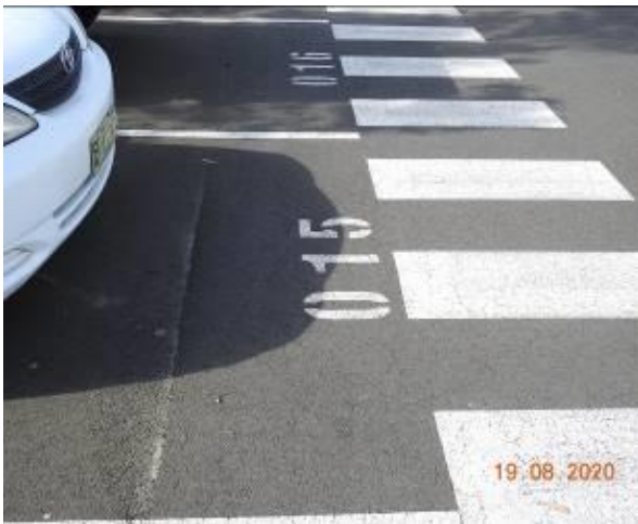
Figure 449 – Crack propagation through car park pavement
