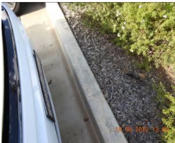
Figure 783 – Hairline cracking through car park kerb
