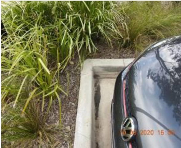
Figure 175 – Crack propagation through car park kerb
