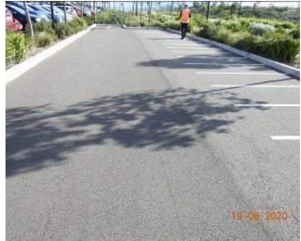
Figure 508 – Crack propagation through car park pavement
