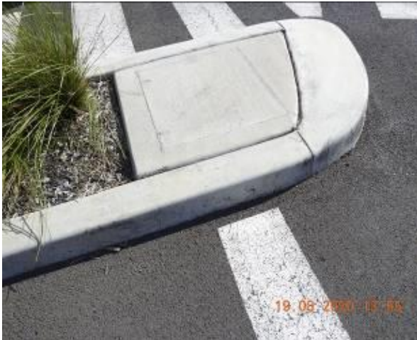
Figure 843 – Hairline cracking through car park kerb
