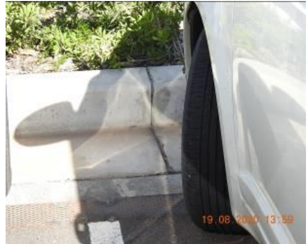
Figure 874 – Crack propagation through car park kerb and gutter
