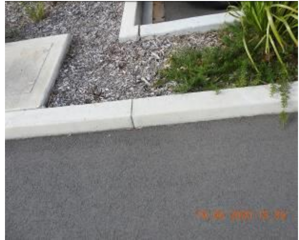
Figure 700 – Crack propagation through car park kerb
