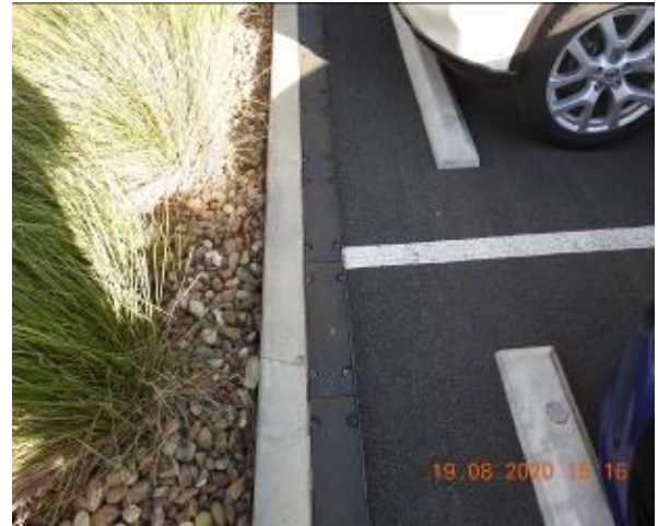
Figure 380 – Crack propagation through car park kerb and service pit
