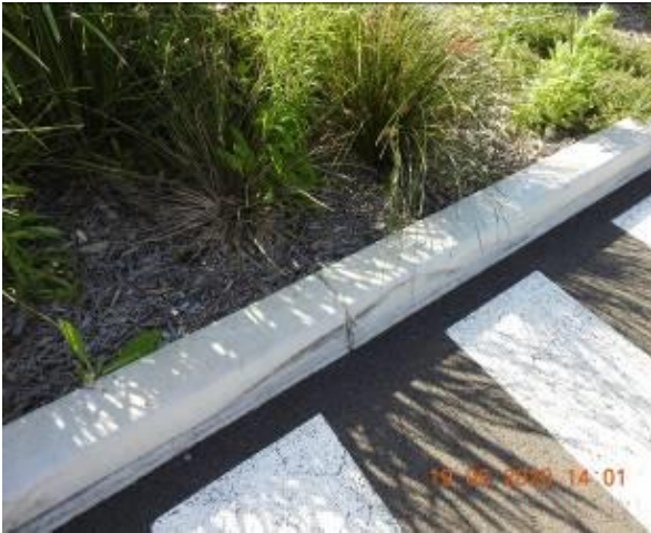
Figure 897 – Crack propagation through car park kerb
