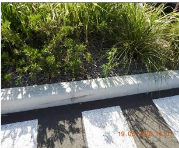
Figure 901 – Crack propagation through car park kerb
