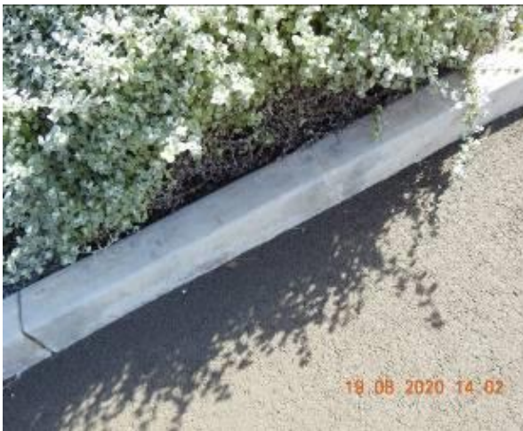
Figure 911 – Crack propagation through car park kerb
