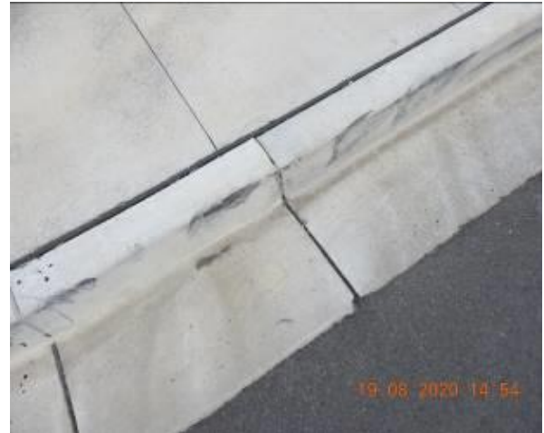
Figure 146 – Hairline cracking through car park kerb
