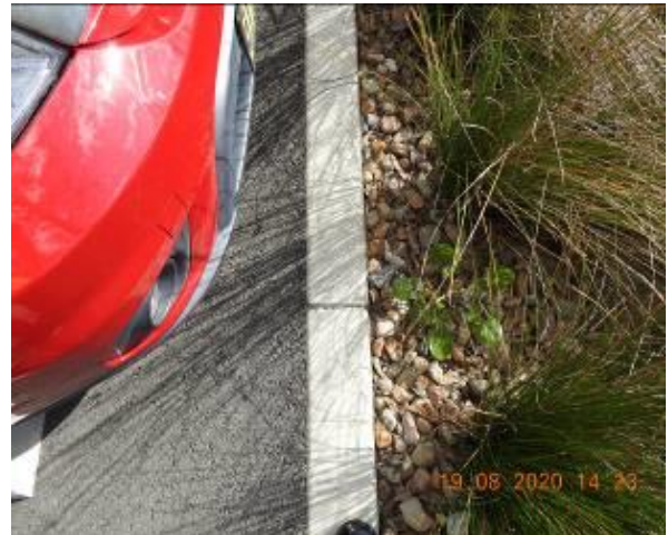
Figure 1140 – Crack propagation through car park kerb
