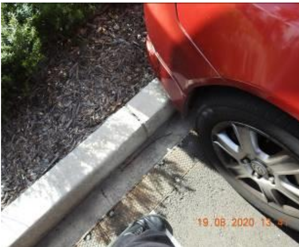
Figure 707 – Crack propagation through car park kerb and gutter
