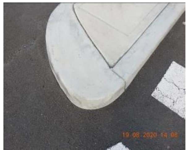
Figure 984 – Hairline cracking through car park kerb
