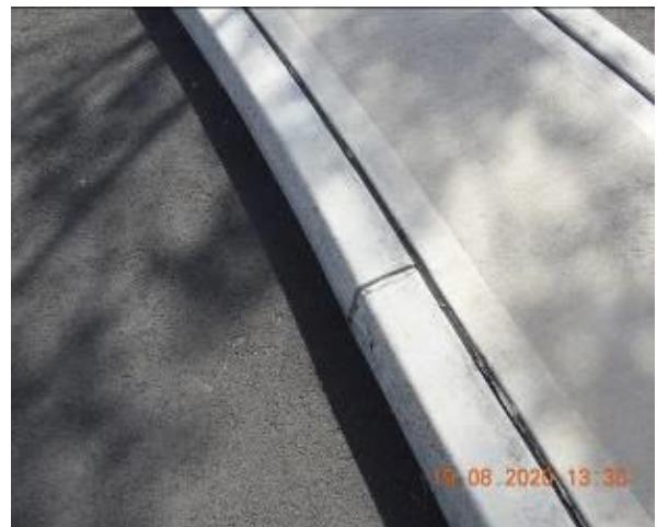
Figure 674 – Crack propagation through traffic island kerb
