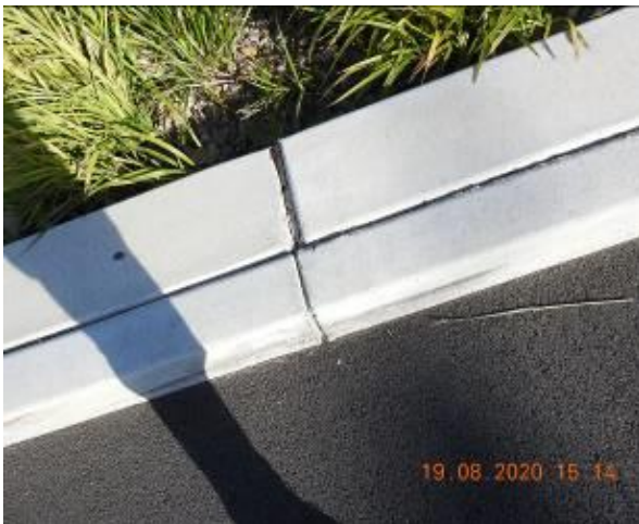
Figure 345 – Crack propagation through car park kerb
