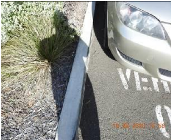
Figure 869 – Hairline cracking through car park kerb
