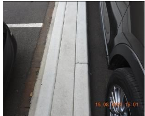
Figure 190 – Crack propagation through car park kerb
