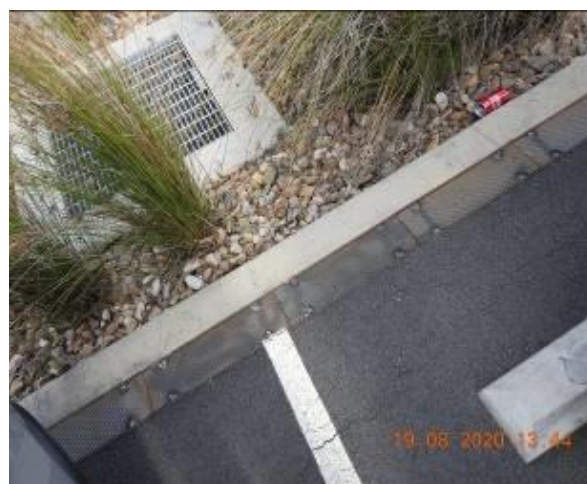
Figure 738 – Crack propagation through car park kerb and General condition of service pit
