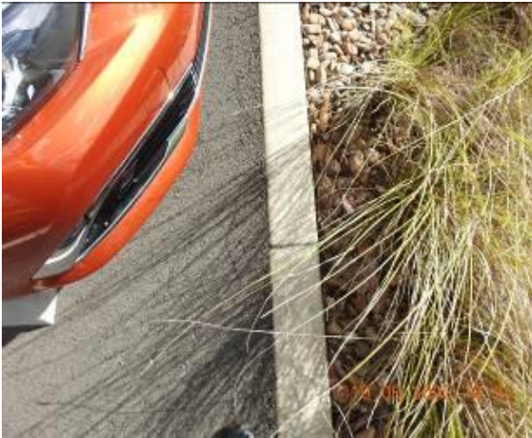
Figure 1149 – Crack propagation through car park kerb
