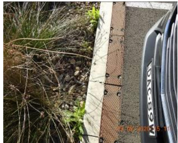
Figure 310 – Crack propagation and loss of material through car park kerb
