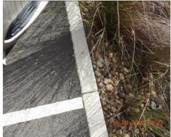
Figure 1138 – Crack propagation through car park kerb
