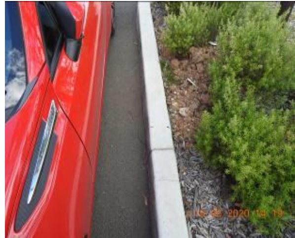
Figure 1084 – Crack propagation through car park kerb
