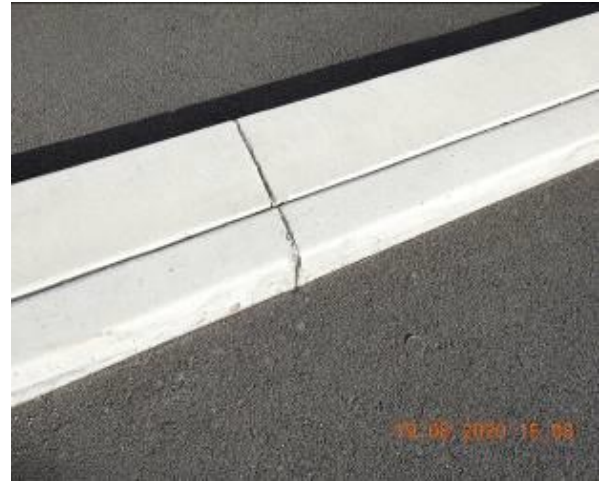
Figure 260 – Crack propagation through car park kerb
