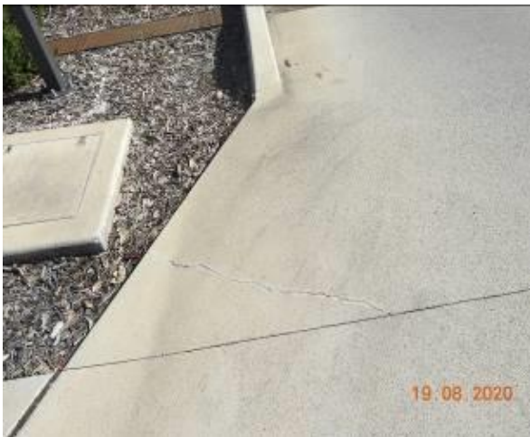
Figure 431 – Crack propagation through car park pavement
