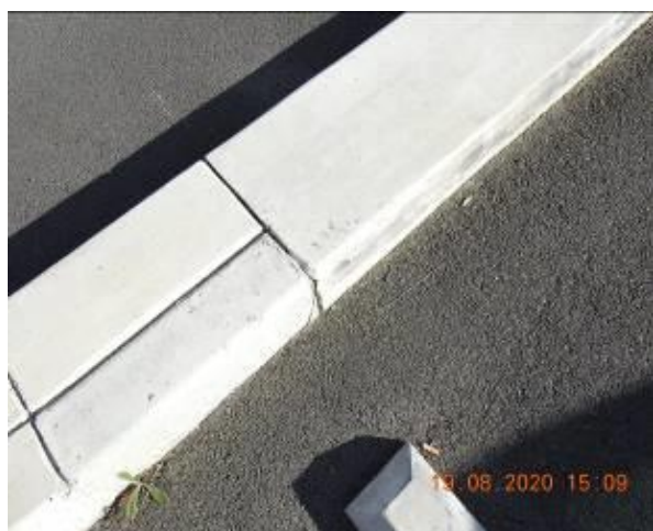
Figure 275 – Crack propagation through car park kerb
