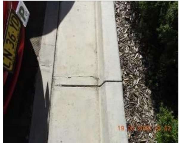
Figure 808 – Crack propagation through car park kerb and gutter
