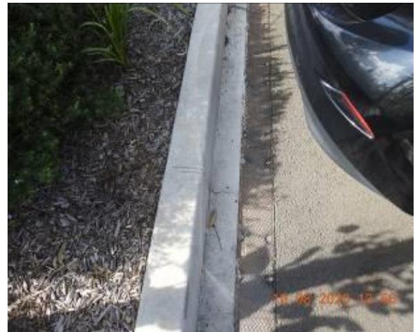
Figure 852 – Crack propagation through car park gutter
