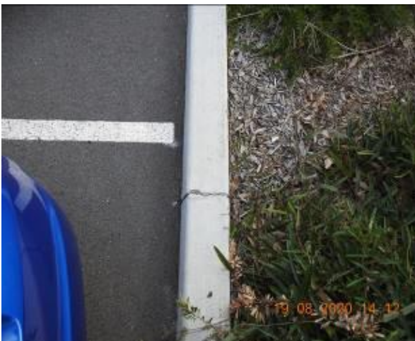
Figure 1009 – Crack propagation through car park kerb
