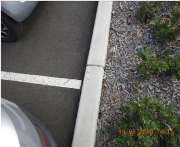
Figure 999 – Crack propagation through car park kerb
