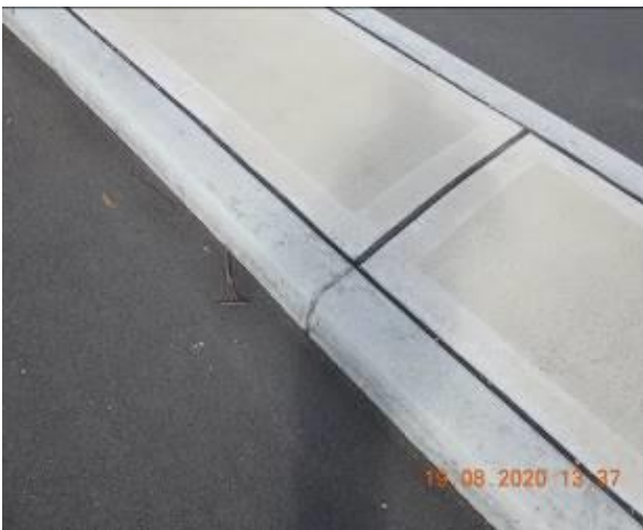
Figure 691 – Crack propagation through traffic island kerb
