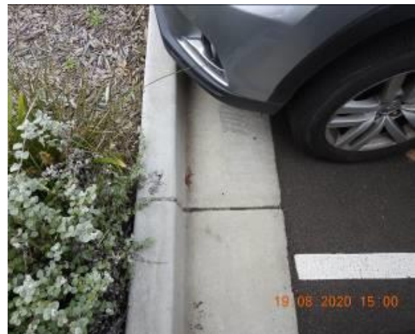
Figure 168 – Crack propagation through car park kerb
