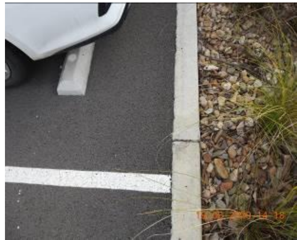
Figure 1068 – Crack propagation through car park kerb
