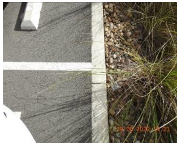
Figure 1154 – Crack propagation through car park kerb
