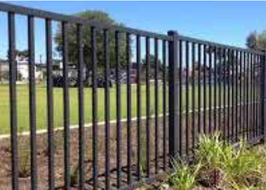
FENCE TYPE 1 -1200MM CHILD SPACE FENCE IN ACCORDANCE WITH THE 'EVERYONE CAN PLAY GUIDELINES'
