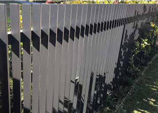
FENCE TYPE 2B-1200MM ALUMINUM BOUNDARY/ SECURITY FENCING.
