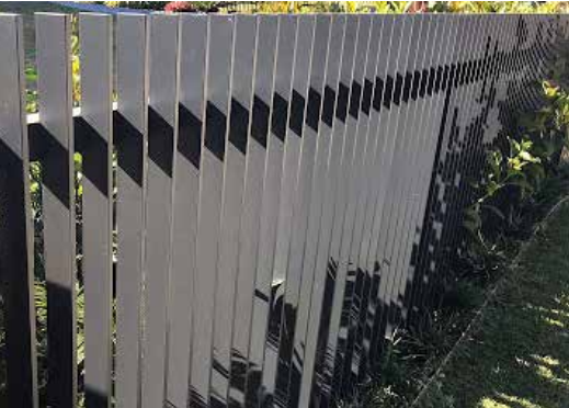
FENCE TYPE 2A-1500MM ALUMINUM BOUNDARY/ SECURITY FENCING. TO BE INSTALLED ON THE BOUNDARY LINE
