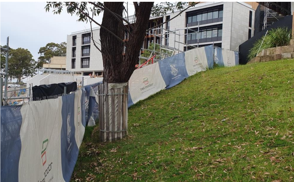
Figure 1-6 Adjacent to construction are, one tree protected in accordance with the flora fauna management plan.
