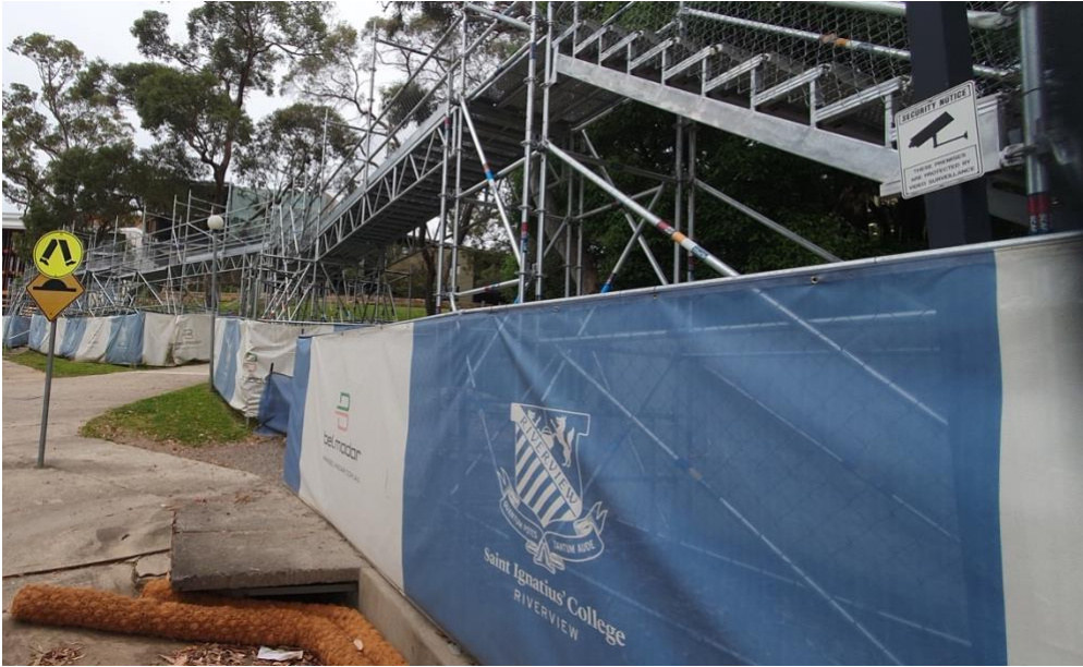
Figure 1-9 Construction site access separated from Pedestrians' walkway.
