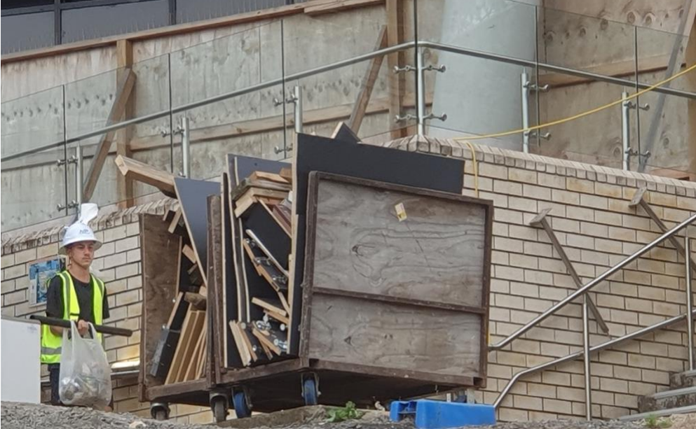
Figure 1-15 Demolition waste separation for daily removal.
