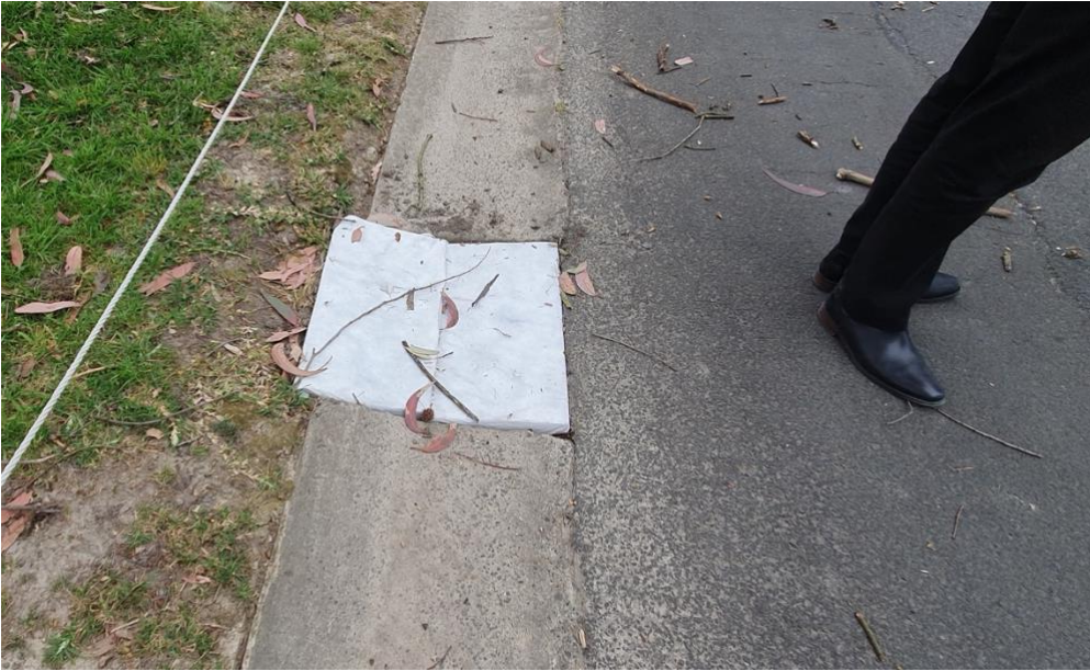
Figure 1-5 Stormwater pits geo-fabric in place and well maintained.
