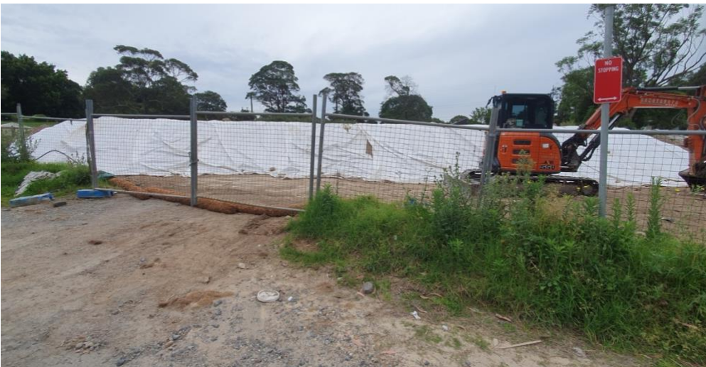
Figure 1-4 Geo-fabric covering stockpiles, sediment fence and coir logs in place
