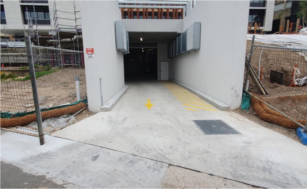
Figure 1-7 Wingaru - basement building access
