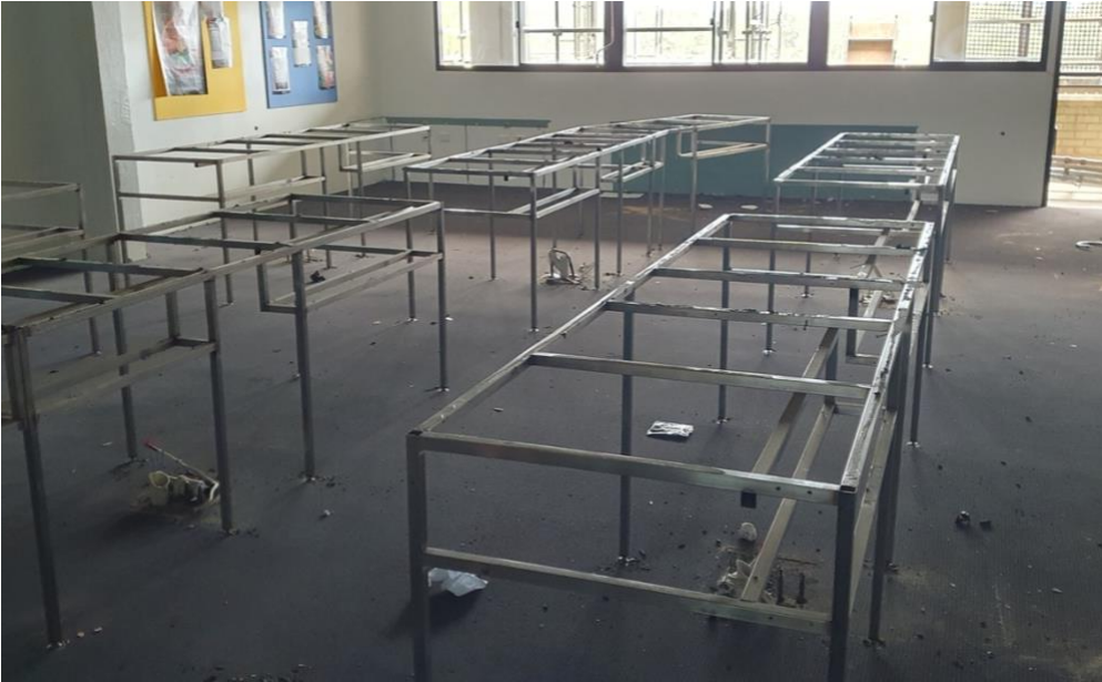
Figure 1-11 O'Neil building internal demolition.
