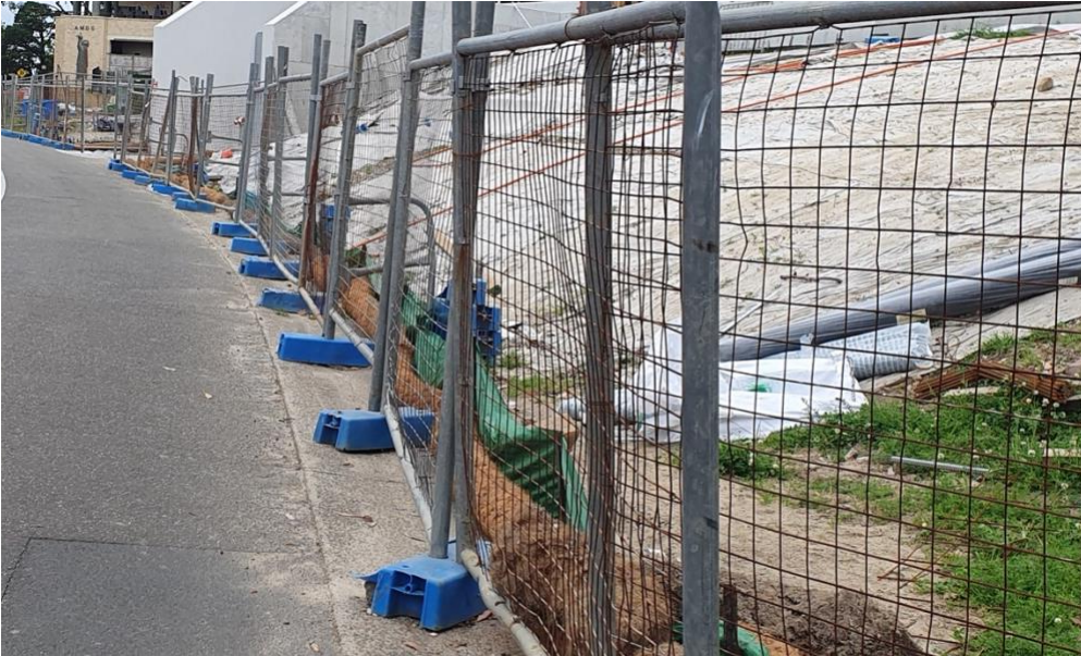
Figure 1-3 Geo-fabric covering slope, sediment fence in place.
