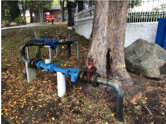
80mm METER AND RPZD ASSEMBLIES
