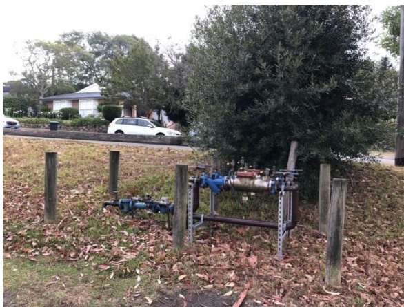
65mm METER AND RPZD ASSEMBLIES
