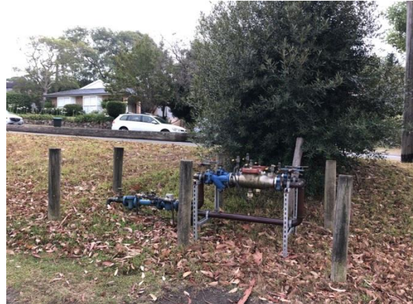
65mm METER AND RPZD ASSEMBLIES
