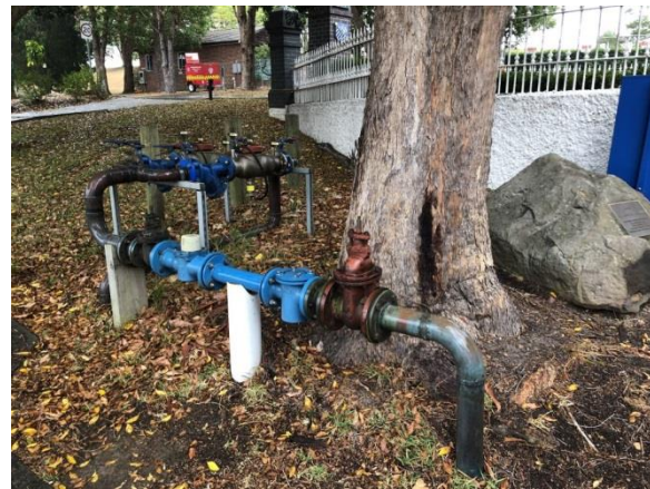
80mm METER AND RPZD ASSEMBLIES
