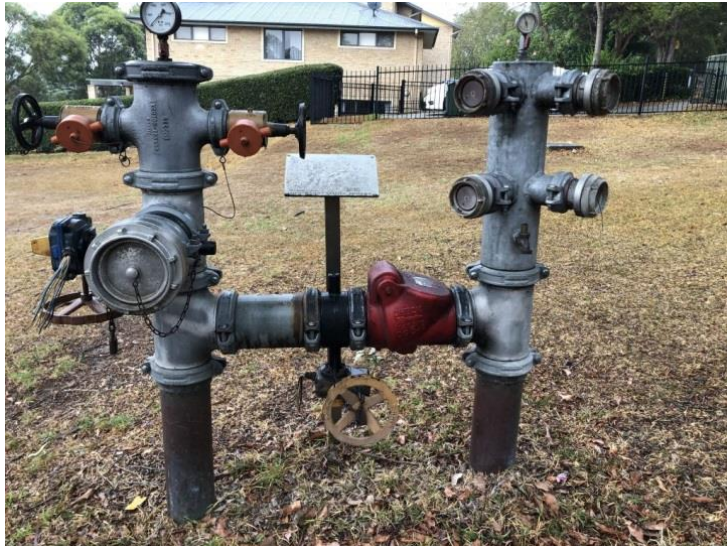
Fire Hydrant Tank Suction and Booster Pump Assembly
