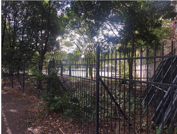
Figure 11: View east from the south west end of the study area showing the fencing, vegetation and concrete tennis/ basketball courts. Proposed new entrance for sporting facilities
