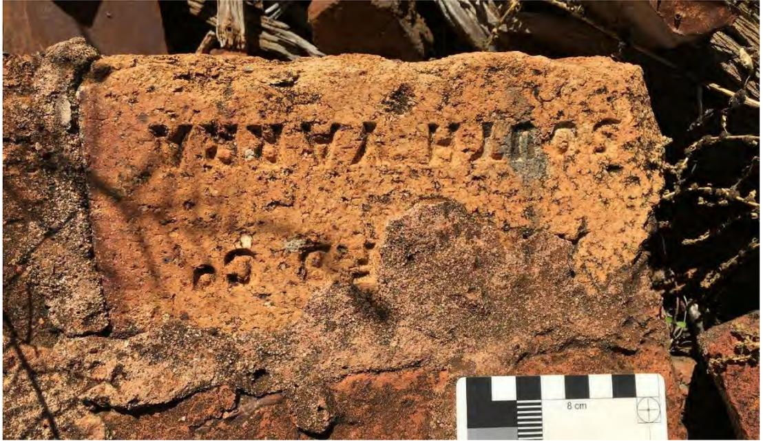
**Plate 5.8** Upended bricks, joined with concrete mortar. Inscribed “... F B Co / SOUTH YARRA”
