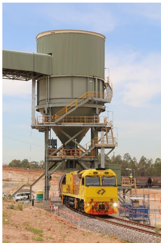
Plate 2-1 Mount Pleasant Operation Stage 1 Train Load-out Facility
