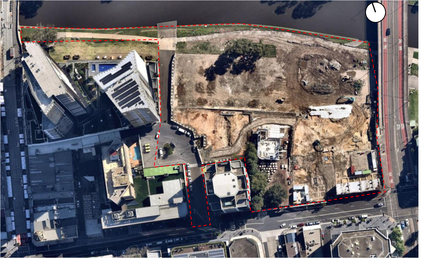
Figure 1-2 The site in mid-October 2021 with the site generally cleared. (Source: Near Map)
