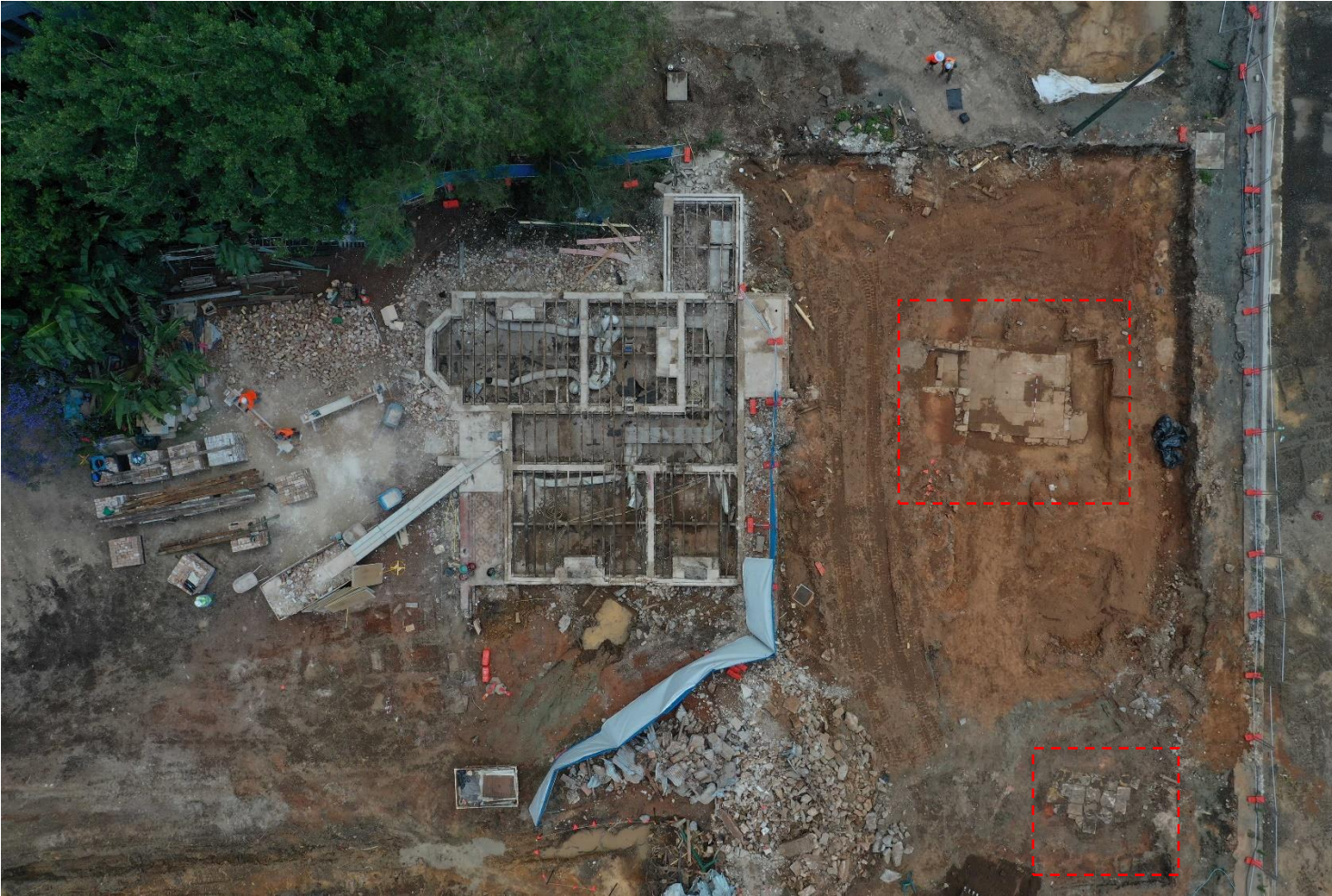
Figure 4-2 Aerial view of the two sandstone features to be subject to salvage excavation and removal (indicated in red outline).
