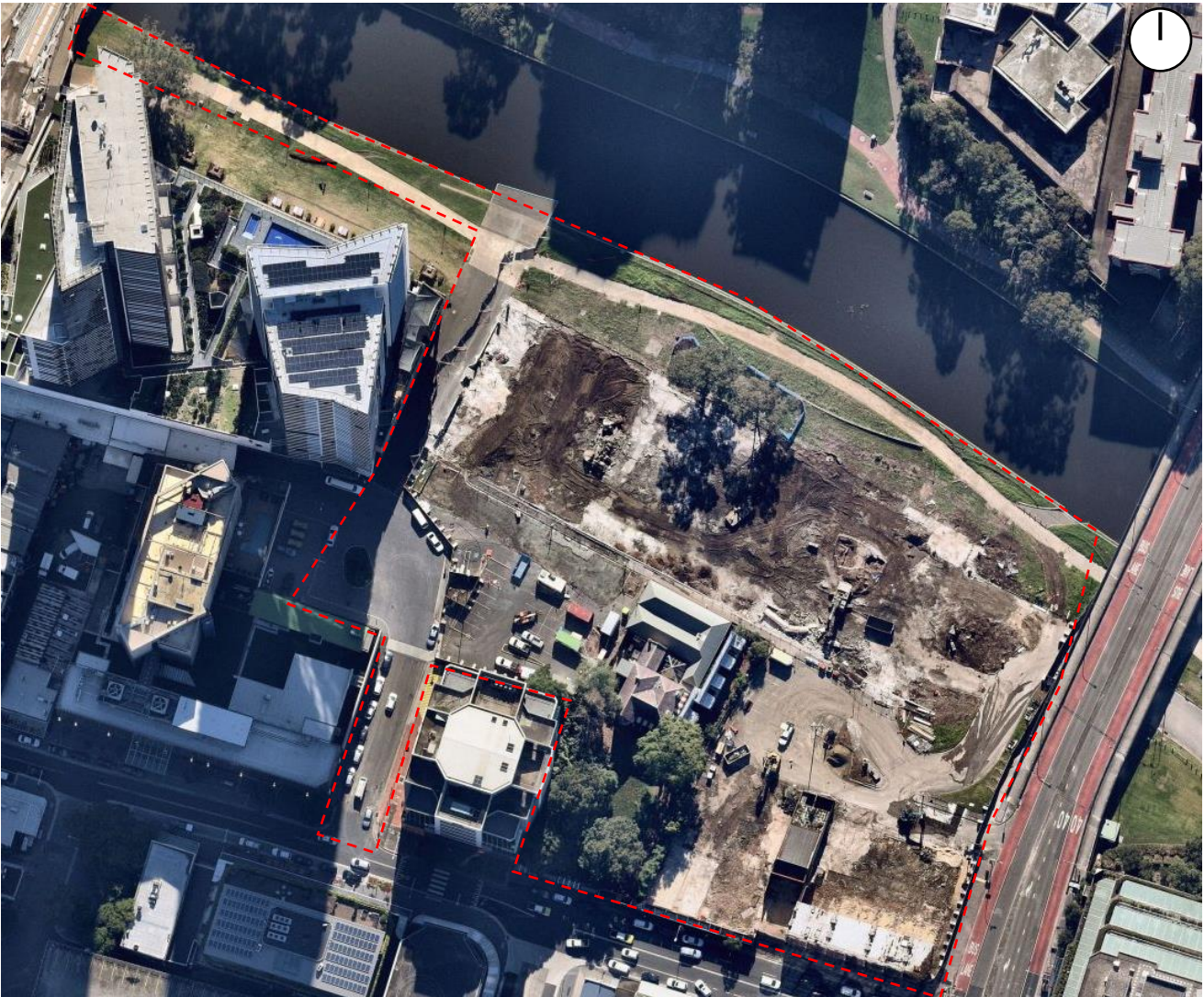
Figure 1-2 The site in early June 2021 with the car park in the process of demolition. (Source: Near Map)
