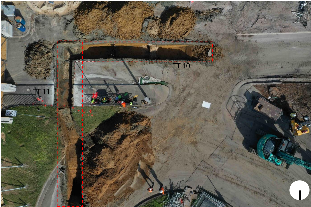
Figure 2-4 Aerial photo showing TT 10 and TT 11.
