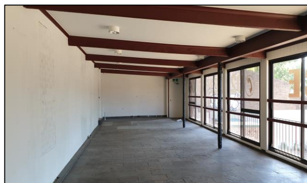
Figure 4-4 First floor rear addition with evidence of former windows infilled on the left wall (Source: Advisian, 2020).
