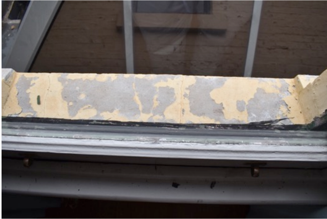
Figure 73 The photograph was taken looking out a window on the first floor to the courtyard. The external window sill shows deterioration and cracked paint. Source: Christopher Roehrig 30 March 2017.
