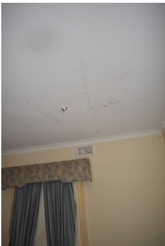
Figure 80 Portion of the ceiling of F.9 illustrates flaking paint and deterioration due to the ingress of water. Source: Christopher Roehrig 30 March 2017.
