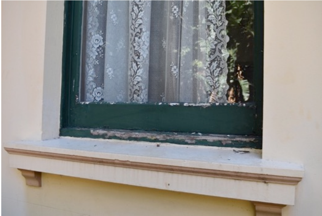
Figure 21 Seen in the photograph is base of one of the windows on the ground floor level. The window frame shows deterioration and flaking paint. Source: May Willard 6 April 2017.
