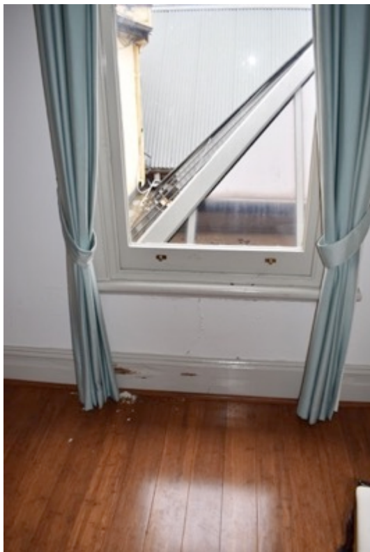
Figure 72 The photograph at the rear of the first floor hallway looks out a double hung window north towards the rear of the property. Visible through the window is the glazed canopy of the courtyard. Water marks are visible on the skirting board below the window. Source: Christopher Roehrig 30 March 2017.
