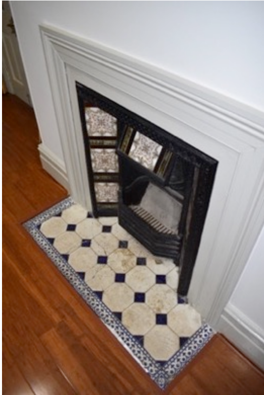
Figure 62 Shown in the image is the fireplace located within F.1. The cast iron insert with decorative tiles or original and intact, although the fireplace hearth has been replaced with a timber architraves. The original mantle pieces were stolen during the transfer of ownership between Telstra (PMG) and Michael and Frank Agostino in 1986. Source: Christopher Roehrig 30 March 2017.
