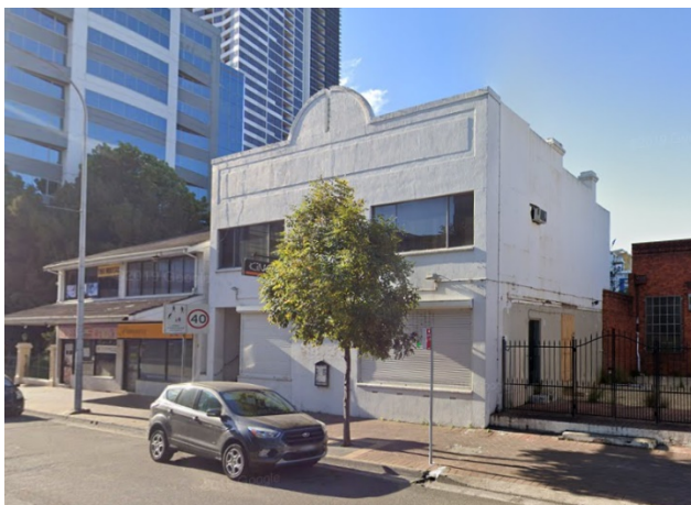
Figure 10 Retail building at 40 Phillip Street
