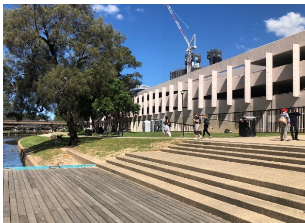
Figure 4 Riverfront carpark building (riverfront side)
