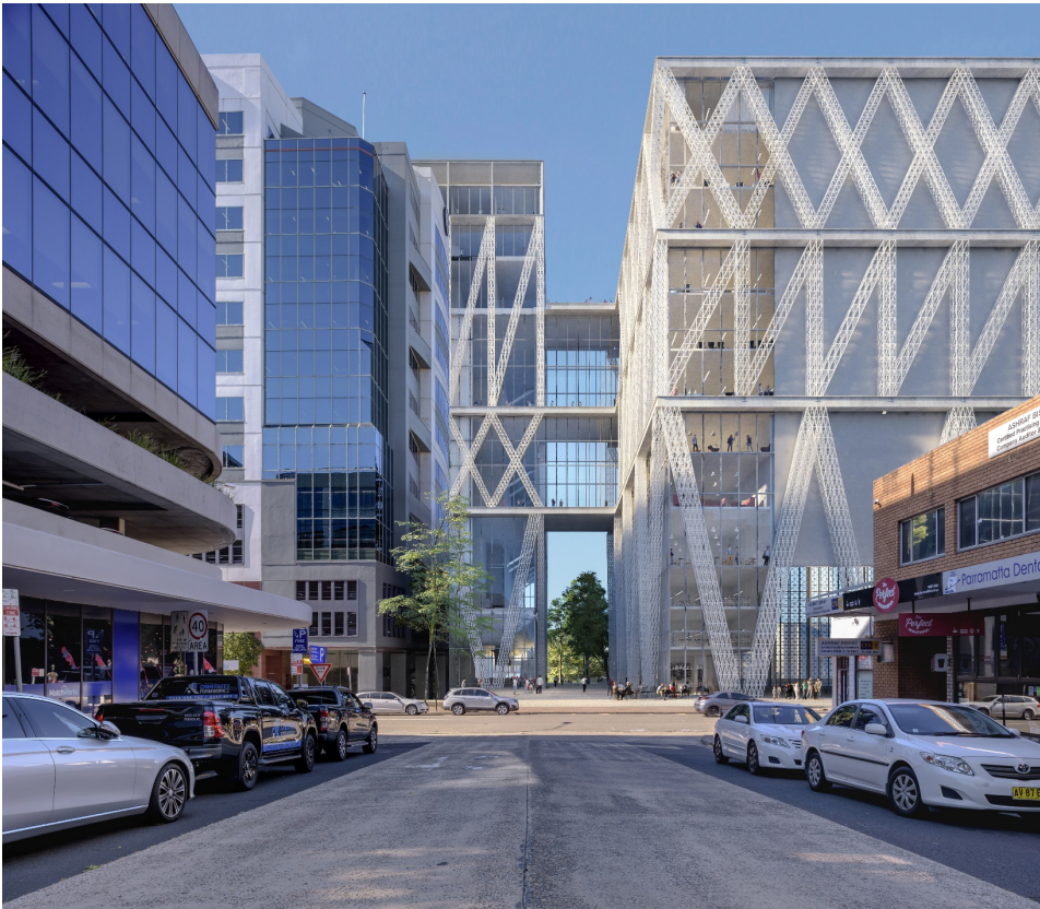
Figure 37 Indicative photomontage of the proposed Powerhouse Parramatta as viewed from Horwood Place (future Civic Link)
