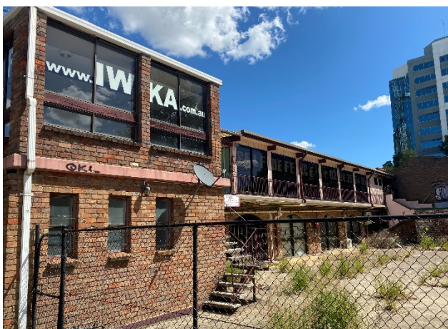
Figure 12 Rear of St Georges Terrace and other retail buildings
