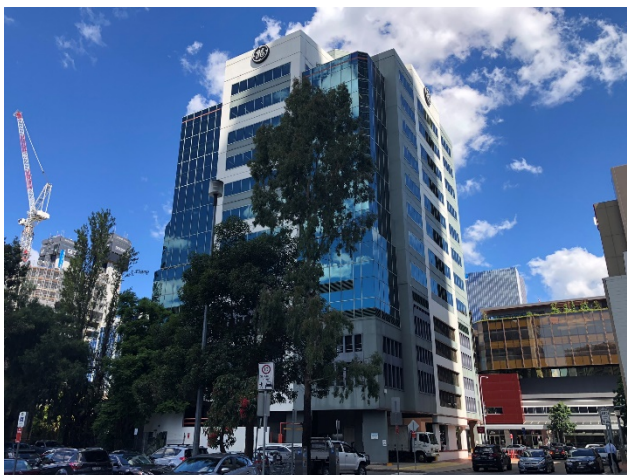
Figure 31 GE Office Building
