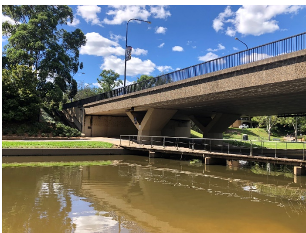
Figure 33 Barry Wilde Bridge, and pedestrian bridge beneath
