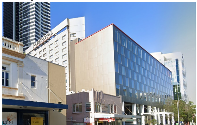
Figure 30 Park Royal Hotel, as viewed from Phillip Street
