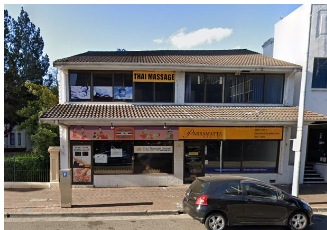
Figure 11 Retail building at 36 Phillip Street
