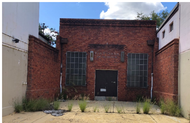
Figure 9 Substation building (42 Phillip St)
