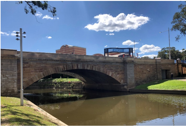
Figure 25 Lennox St Bridge and the Riverside Theatre behind
