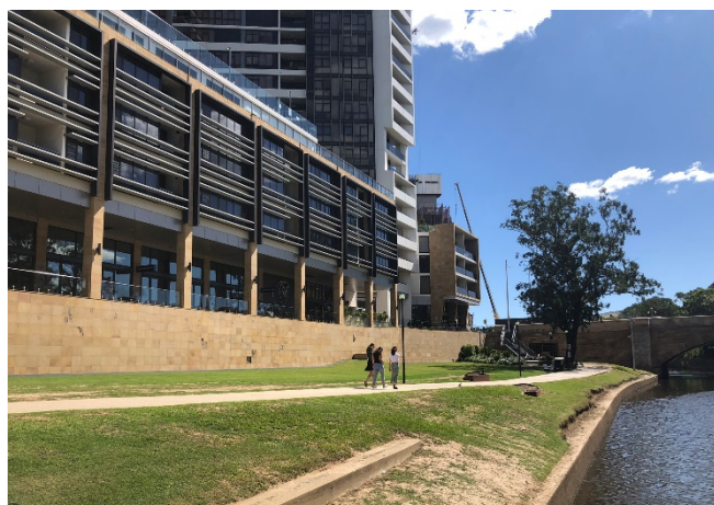
Figure 13 Riverfront portion of the site extending to Church Street
