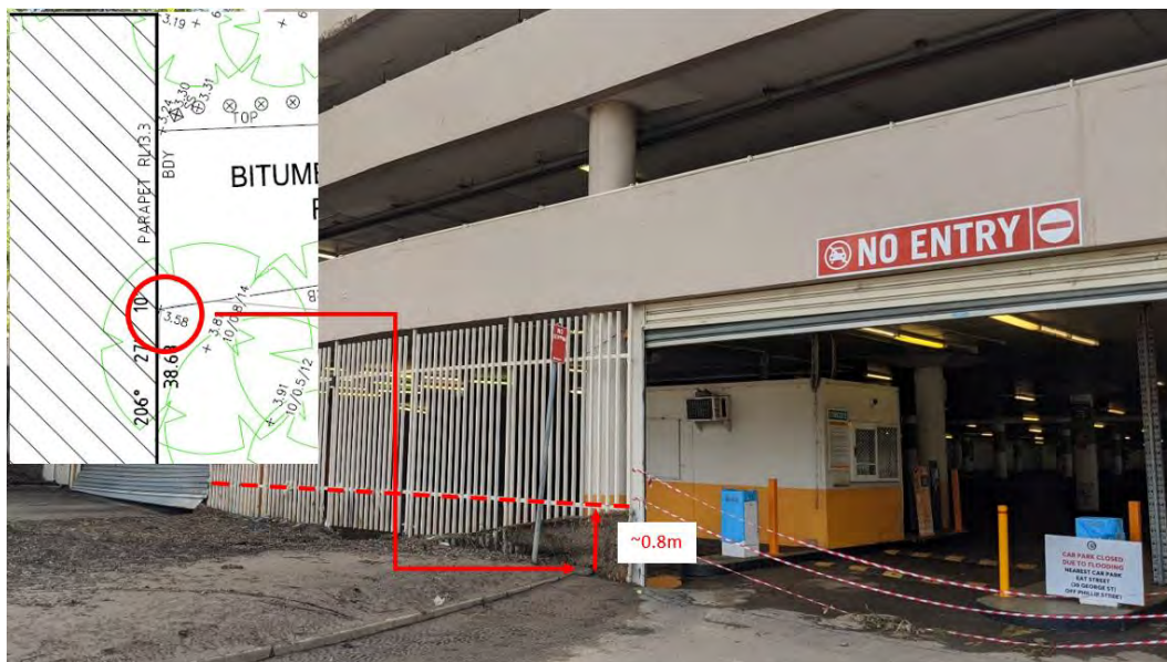
Figure 11: Photograph of debris line on the façade of the Riverside car park following the February 2020. Arup estimate the peak flood level as 4.4 mAHD on the development site
