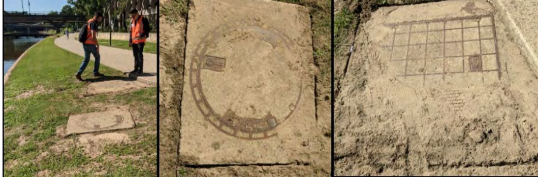
Figure 22: Existing GPT near Ø600 mm trunk outlet
