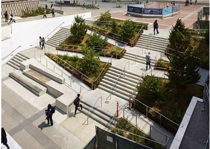
Stainless Steel Balustrades and Planting through stairs
