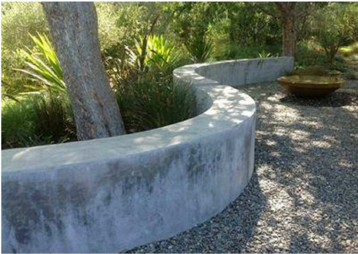
Curved Concrete Walls
