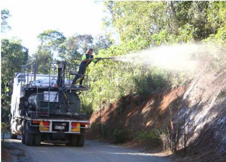
Figure 3-1 Hydromulch application (Catchments & Creeks Pty Ltd, 2010)
