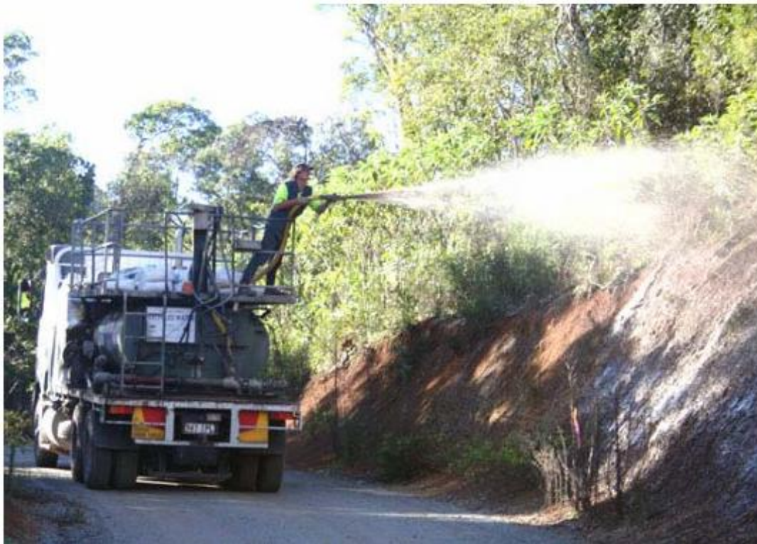
Figure 3-1 Hydromulch application (Catchments & Creeks Pty Ltd, 2010)
