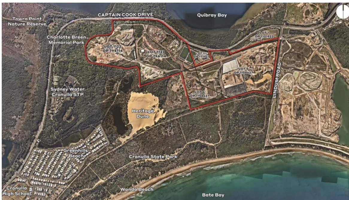
Figure 4 Aerial Photograph of the Site
