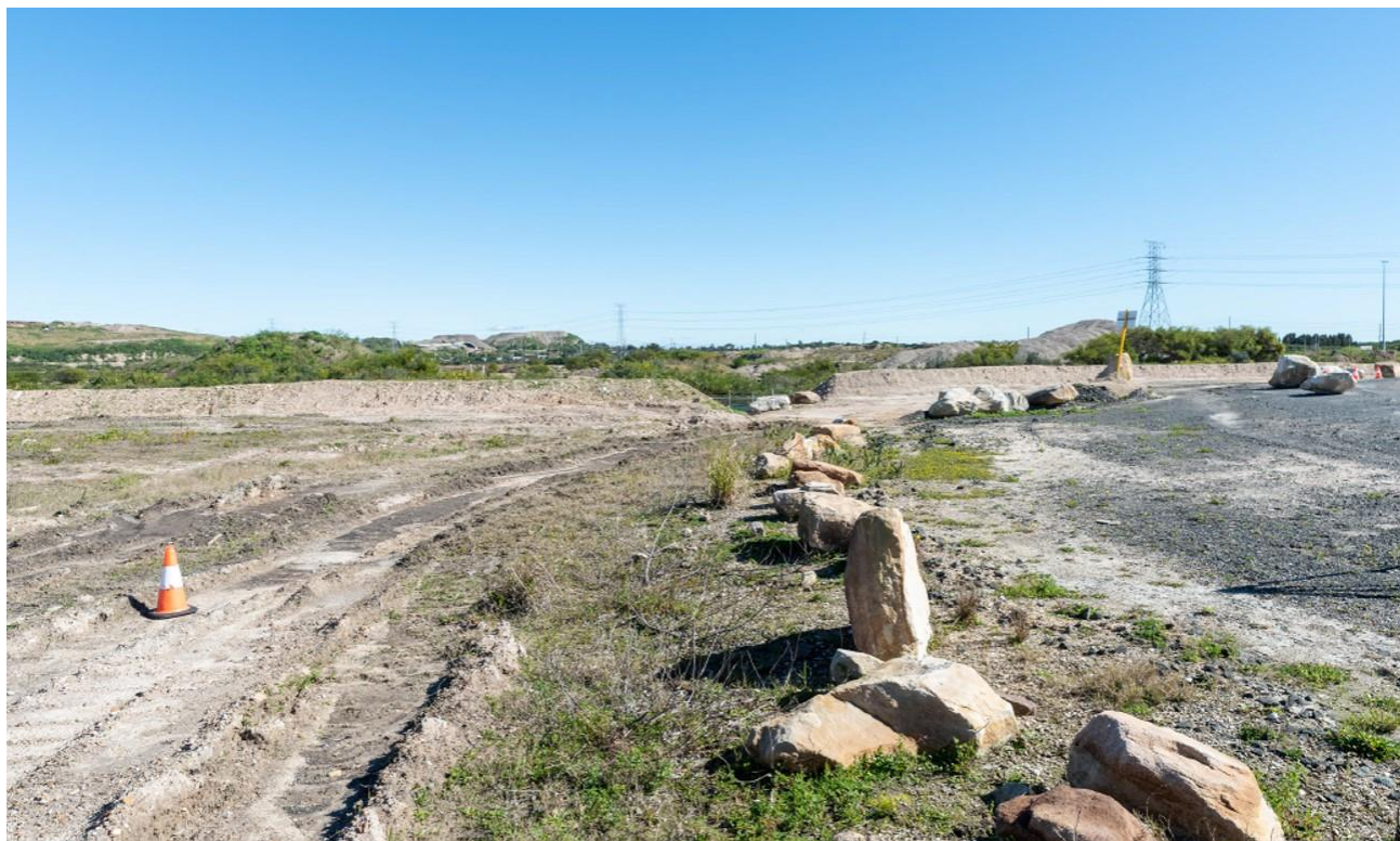
Figure 12 View 8: View looking west across Lindum Road which sits behind the soil batter
