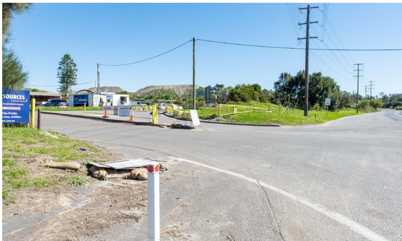
Figure 14 Existing site access arrangements with Captain Cook Drive, looking north-west
