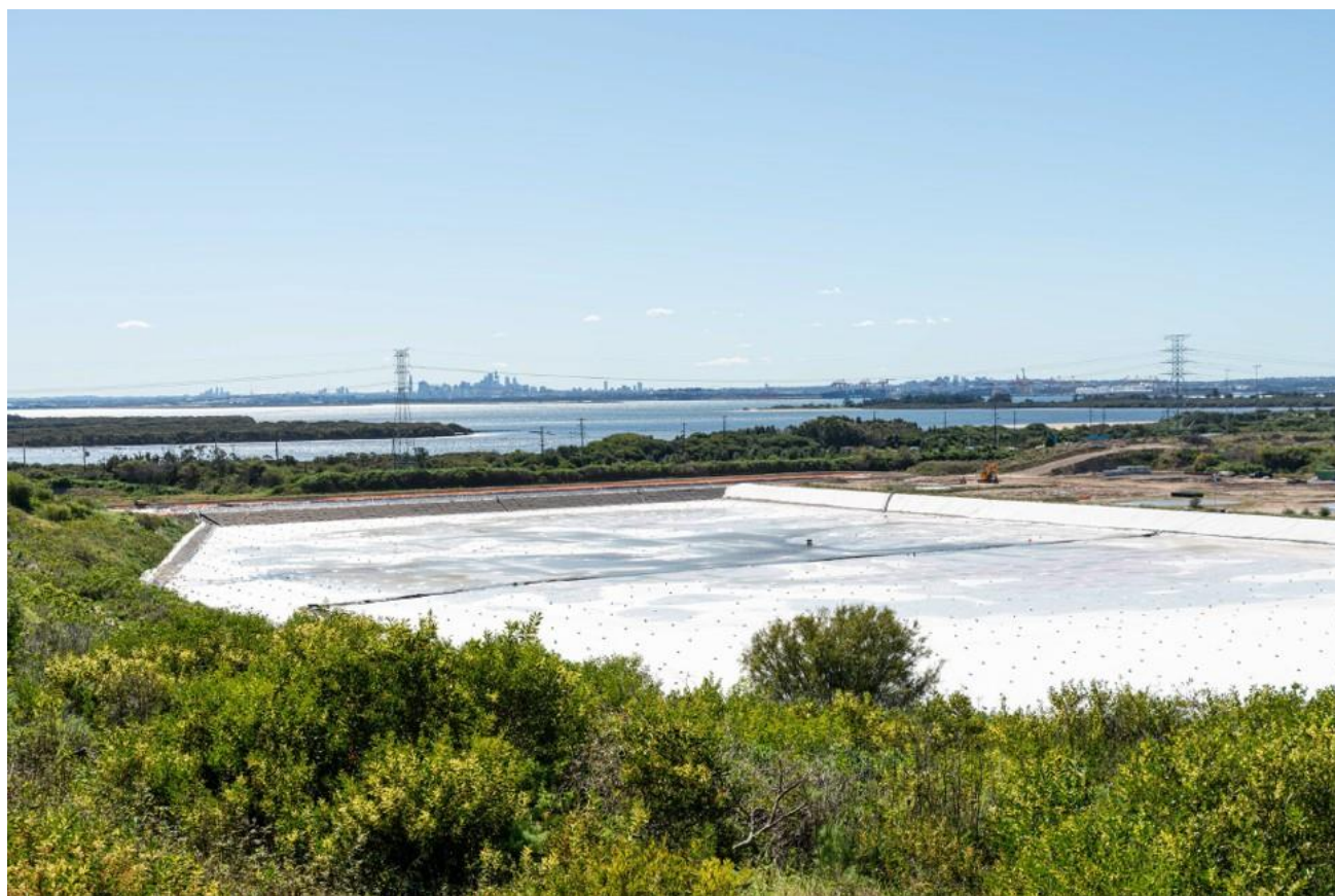
Figure 5 View 1: Looking north-east across Lot 5 in the foreground with the Towra Point Nature Reserve in the mid-ground and Botany Bay in the background
