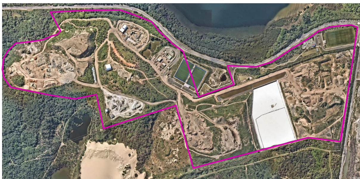
Figure 63 Aerial photograph showing the extent of vegetation clearance
