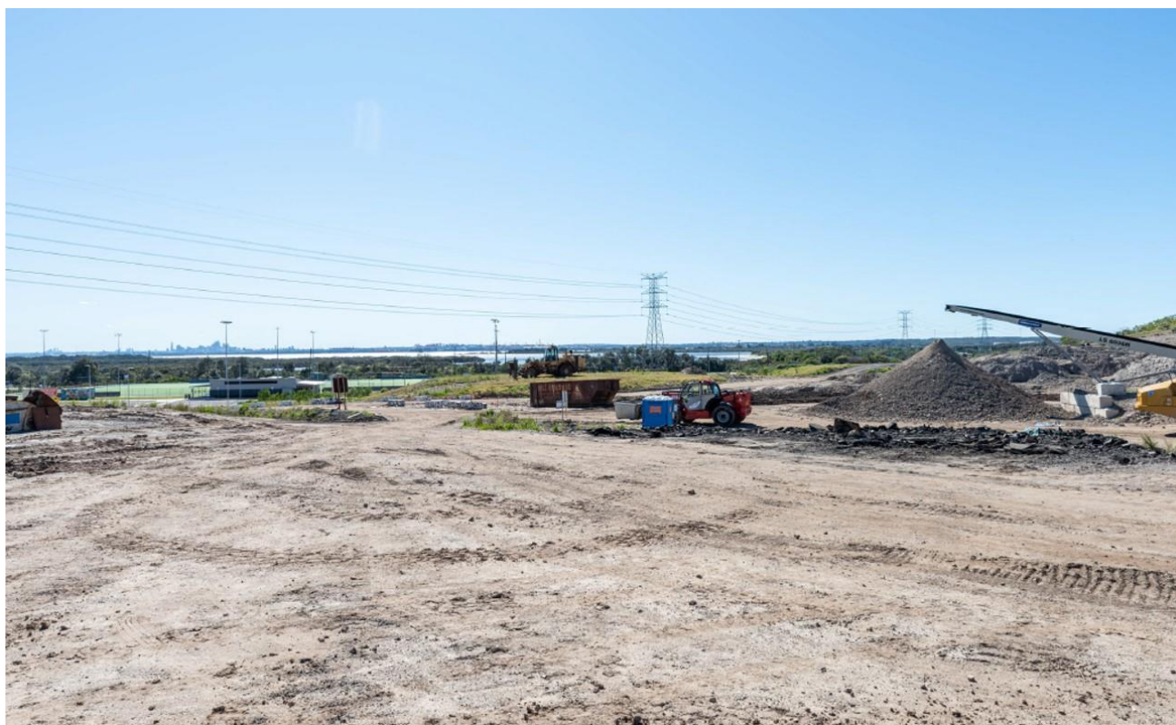
Figure 10 View 6: Looking north-east across the future playing fields on Lot 6, with the Heritage Dune behind
