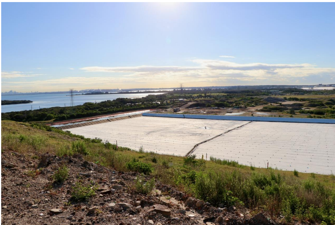
FIGURE 51: View over eastern part of the Proposal Site and new landfill cell (under construction)
