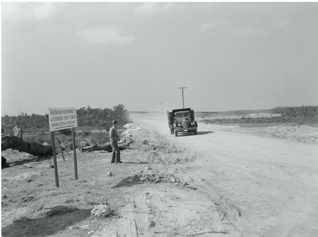
FIGURE 22: Caltex Oil Refinery Site on Captain Cook Drive (September 1953)
