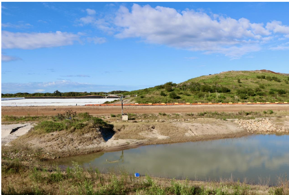
FIGURE 52: View from northern boundary access road towards new cell and fill mound
