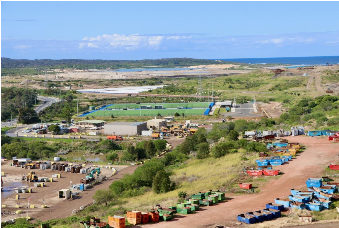
FIGURE 58: View across the Proposal Site from the western fill mound
