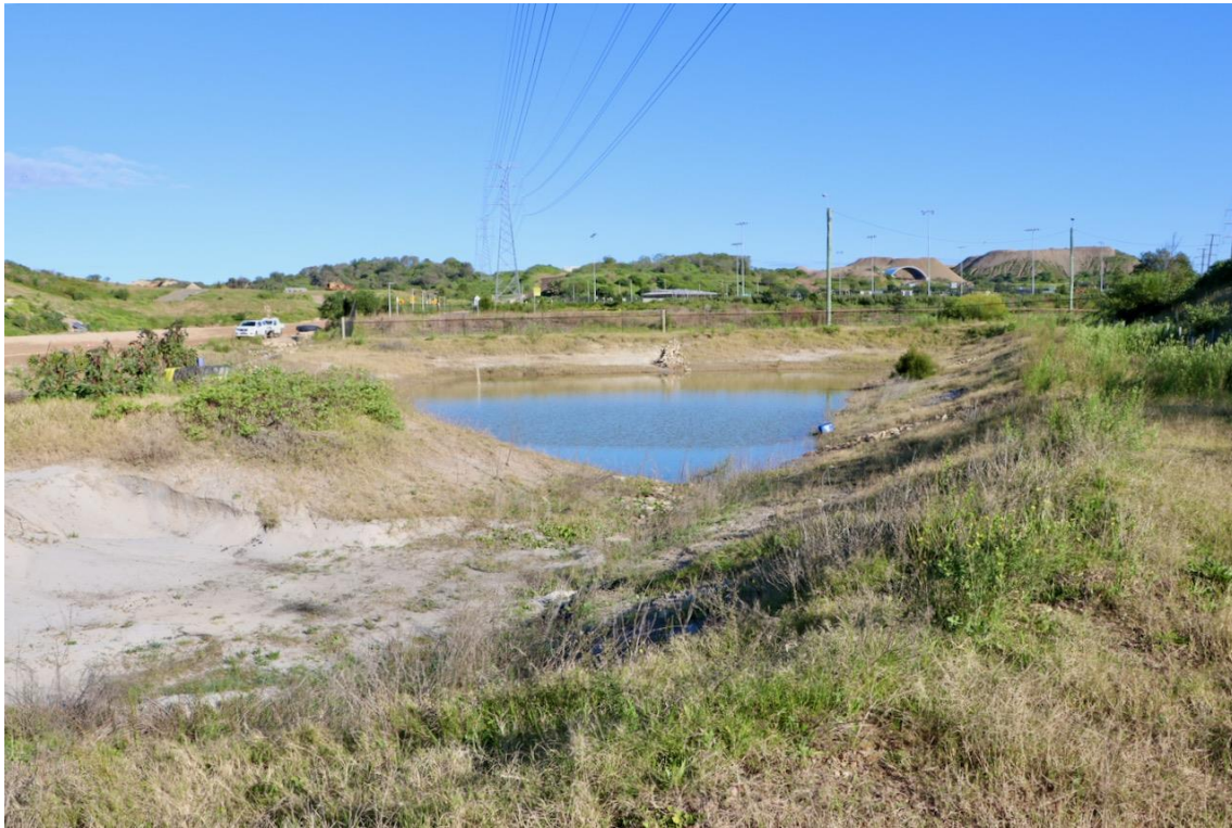
FIGURE 54: General view along HV powerline towards western part of Proposal Site/fill mounds View W – Dan Tuck 2020
