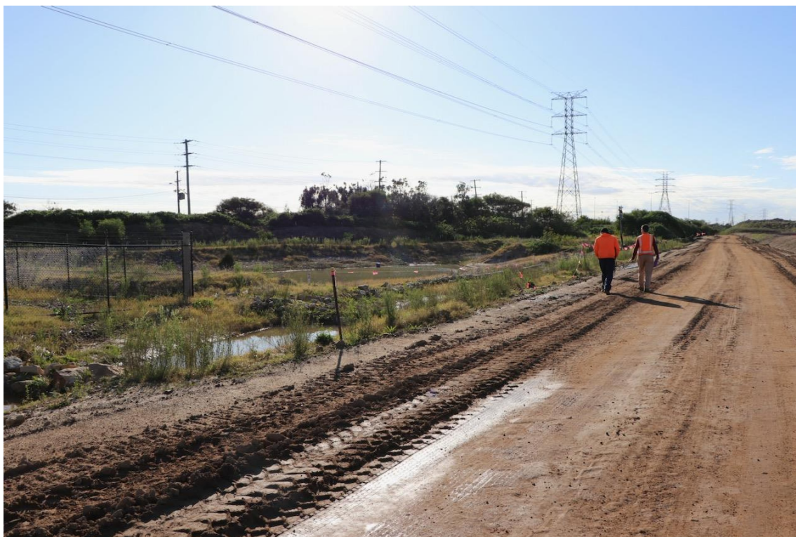
FIGURE 53: General view along one of the internal site access roads (HV powerline overhead)
