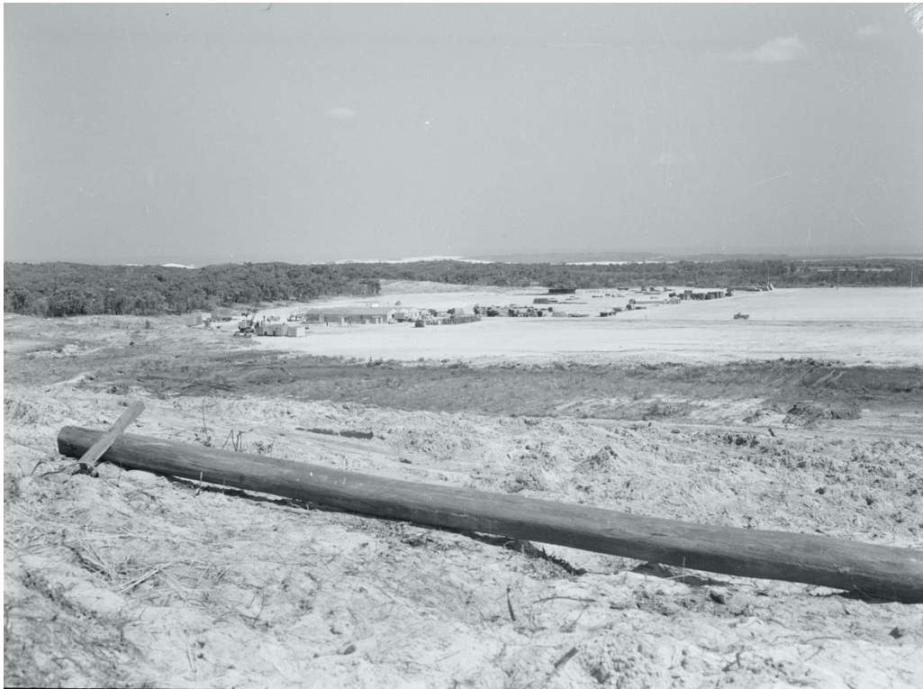
FIGURE 23: Caltex Oil Refinery Site (September 1953)
