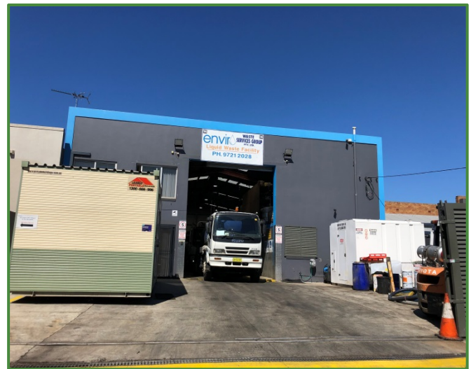
Figure 1: View of existing Enviro Waste facility (14 Kiora Crescent) from Kiora Crescent
