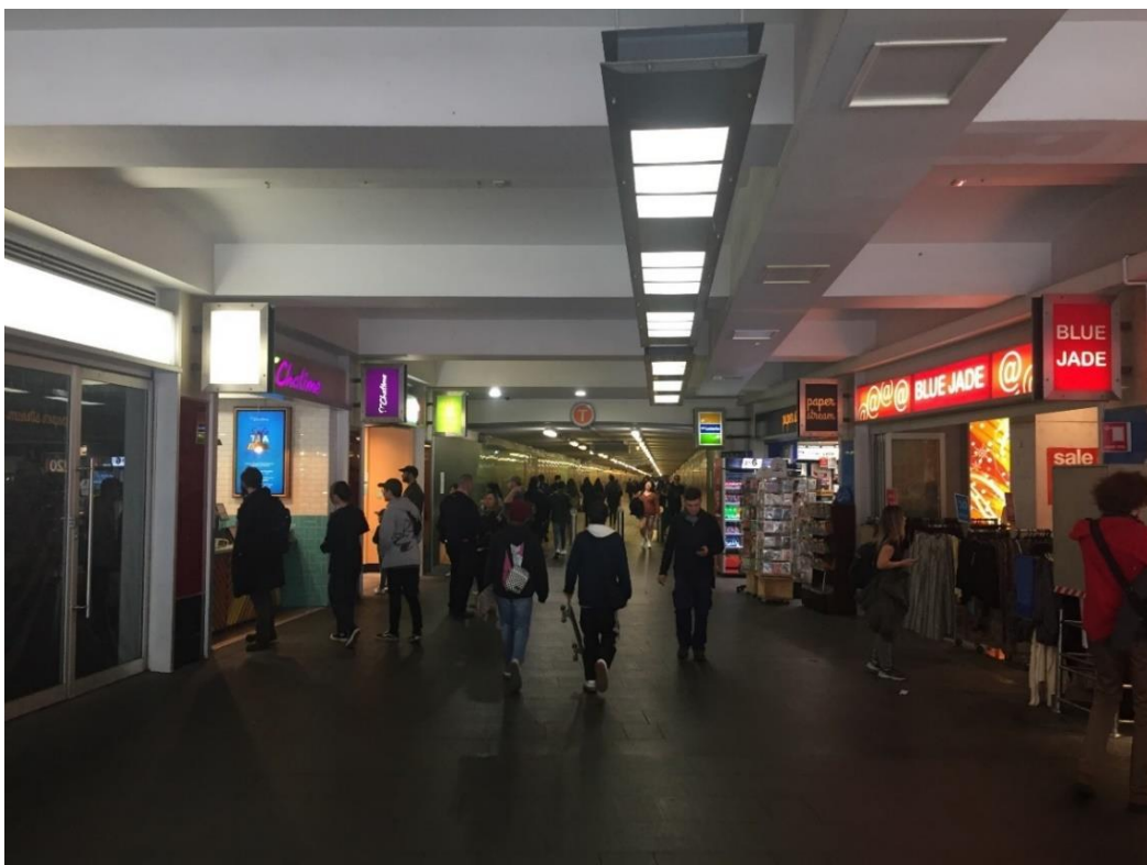
Figure 1-6: Existing Devonshire Street Tunnel (West)
