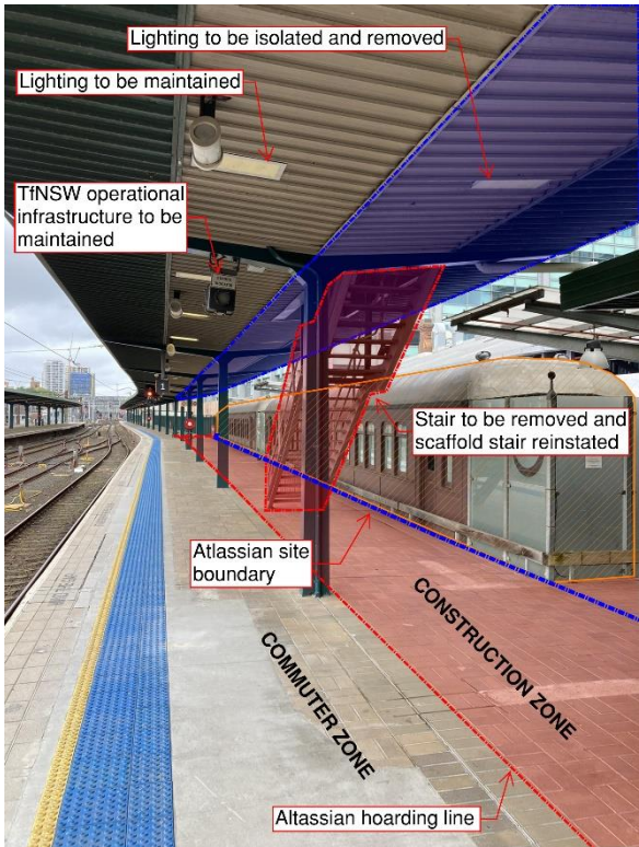
Figure 2-3b: Platform 1 awning modifications
