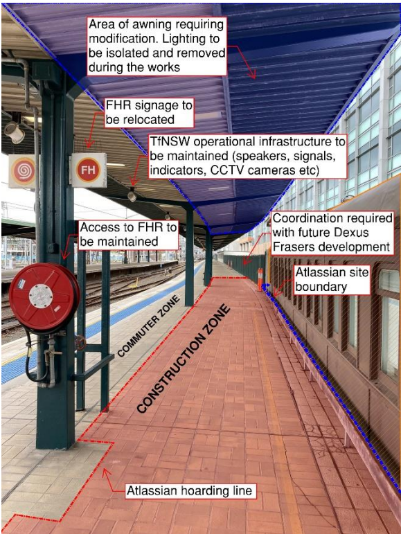
Figure 2-3a: Platform 1 awning modifications
