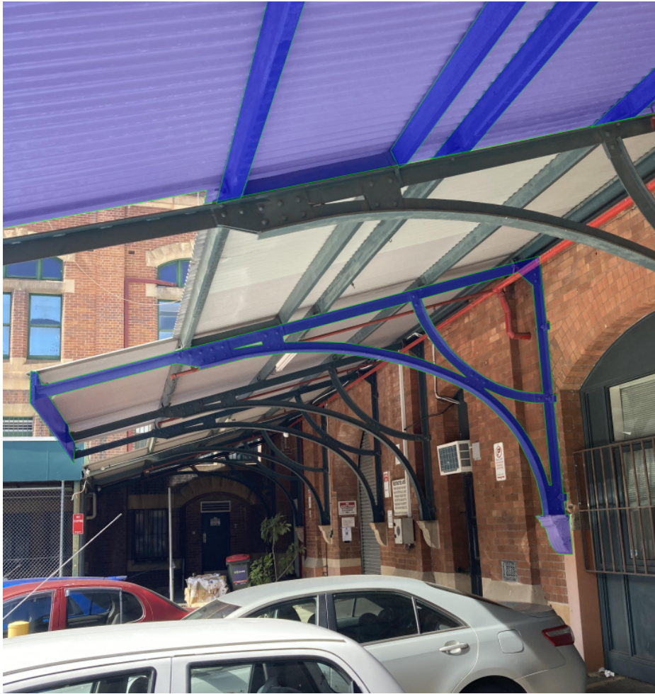
Figure 1-11: Southern awning structure
