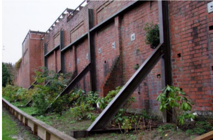
Figure 1-18: Heritage Wall Bracing Examples – Adina Hotel Side
