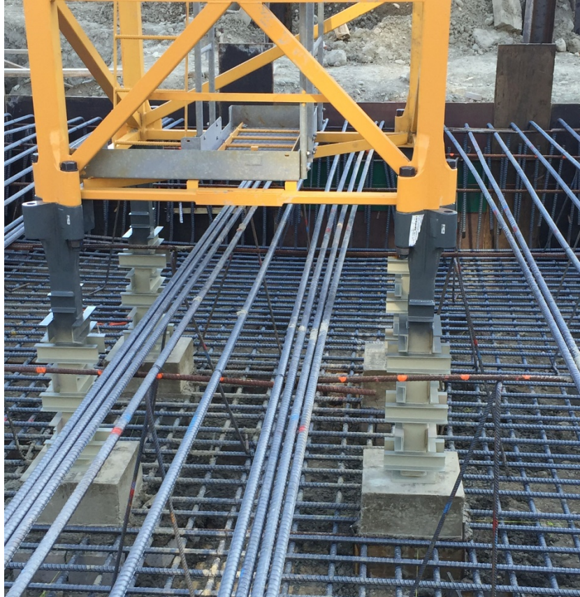
Figure 1-45: Tower Crane 2 Base
