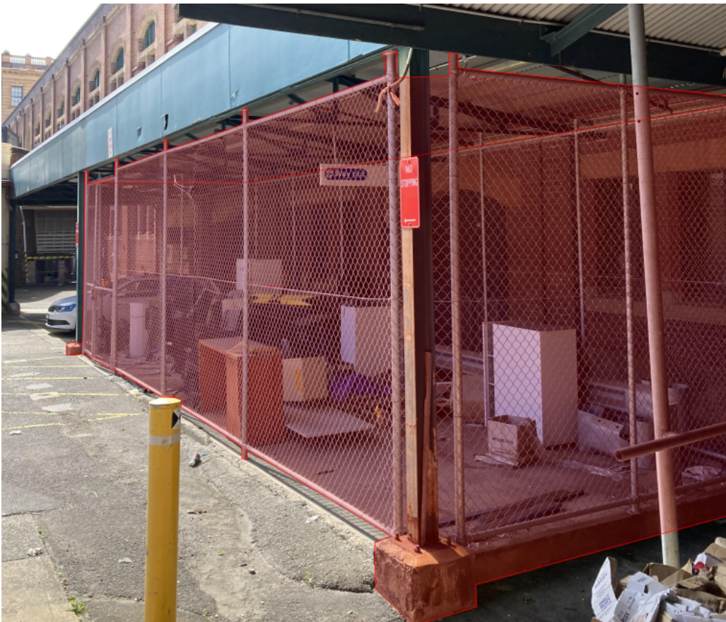
Figure 1-10: Ambulance Avenue chain-wire storage compound
