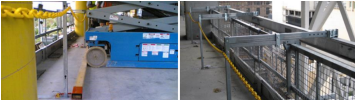
Figure 1-59a: Photographic Example of WorkRight Edge Protection System
