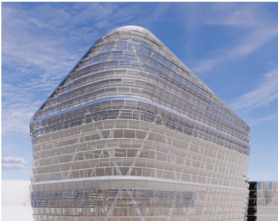
1.5 FIGURE 3 - PREVIOUS DESIGN: CROWN EXTERIOR FACADE TO BE FIXED GLASS LOUVRES - VIEW FROM NORTH WEST
