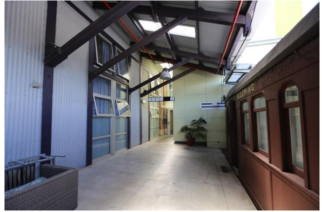
Figure 15 – Southern elevation of amenities addition to the east of the shed.
