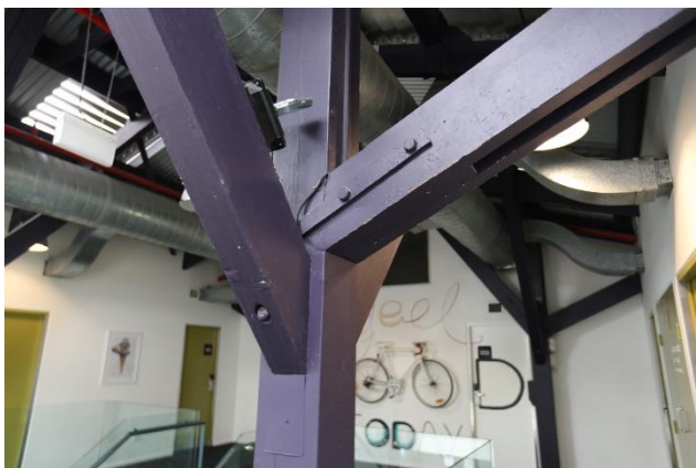
Figure 5 – Detail of timber post and struts
