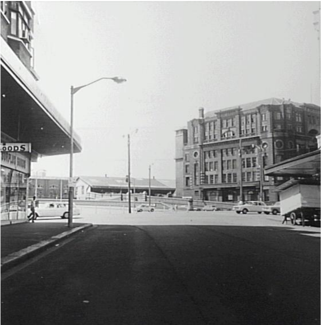
Figure 92 – View south-east along Quay Street toward the Inwards Parcels Shed and the Parcels Post Office on 13 January 1970.
