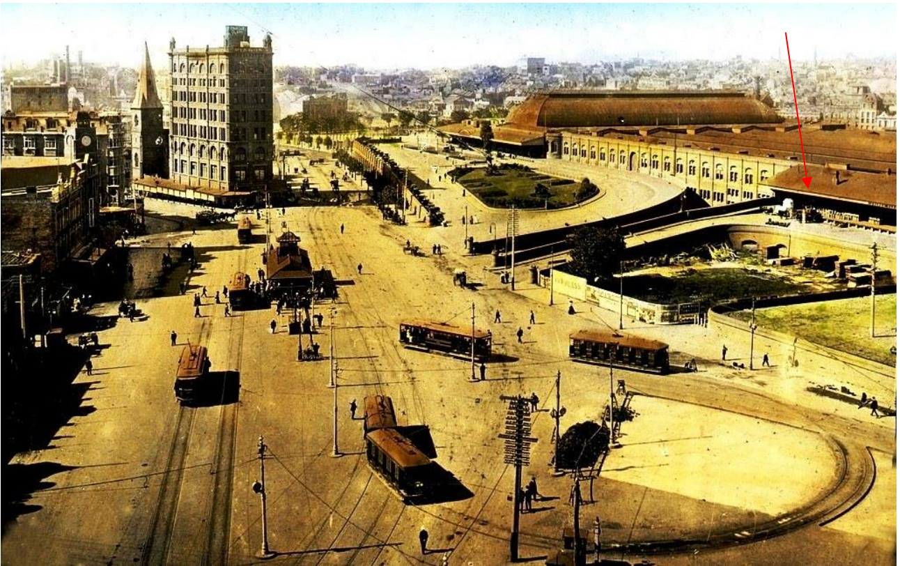
Figure 85 – c. 1906-1913 view of Railway Square, with the Inwards Parcels Shed indicated by the red arrow at the right. Source: Flickr
