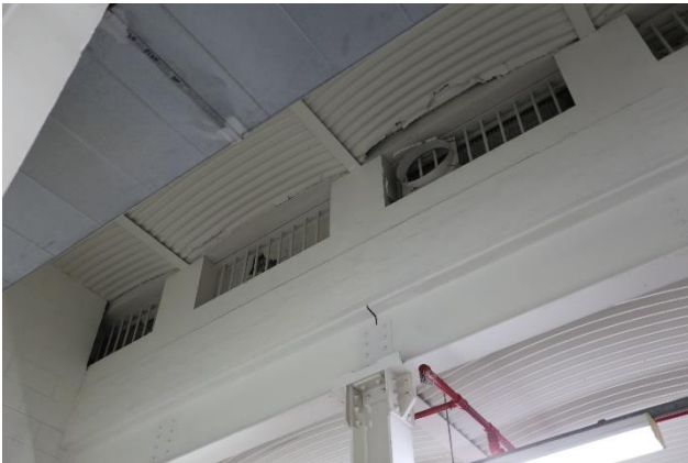
Figure 56 – Basement lights, with early bars and glazing still intact
