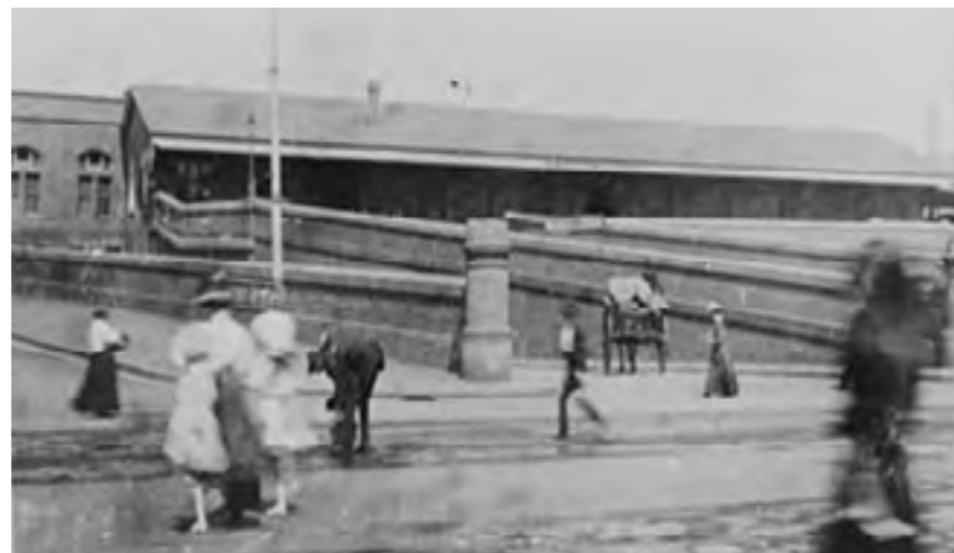
Figure 4 Sydney Central Railway Station site, during the construction of the Parcels Post Office, c.1906-1913. View from Pitt Street east towards the west elevation of the Parcels Shed. Source: National Archives of Australia, Series No. C4076, Control symbol, HN16075B
