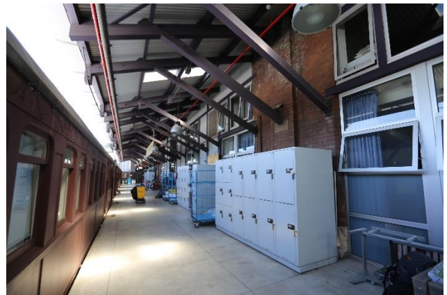
Figure 17 – Concrete platform at the east of the building, looking south.
