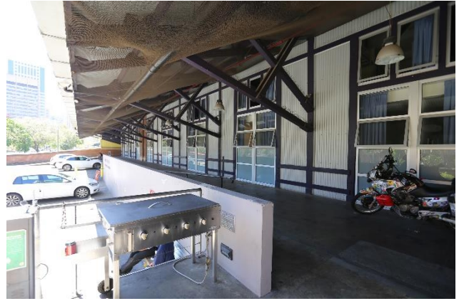
Figure 9 – West elevation of the shed, with the timber expressed frame and new aluminium windows
