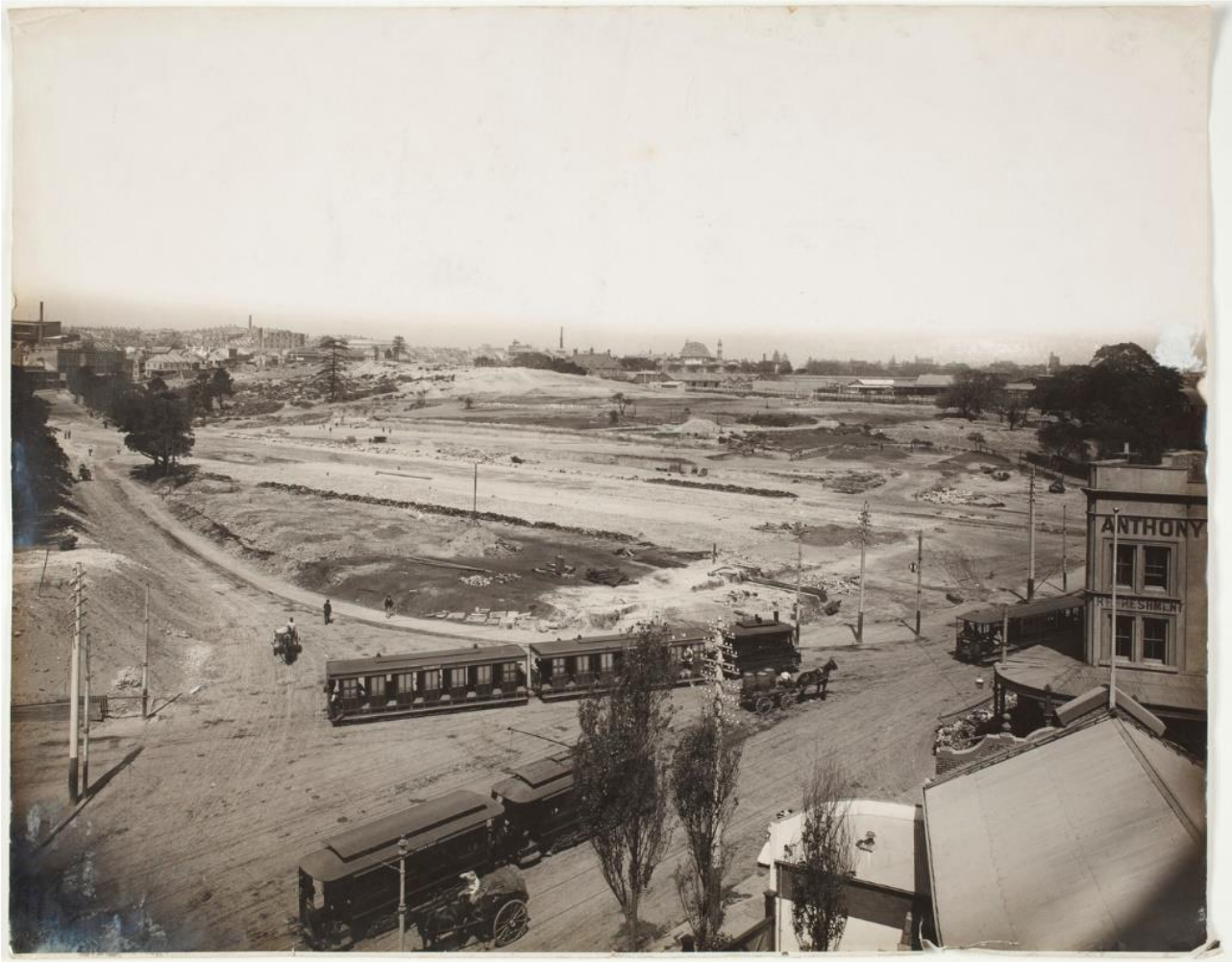
Figure 76 – Looking back towards Redfern Station, cleared land for Central Station Source: State Library of NSW, IE11306447
