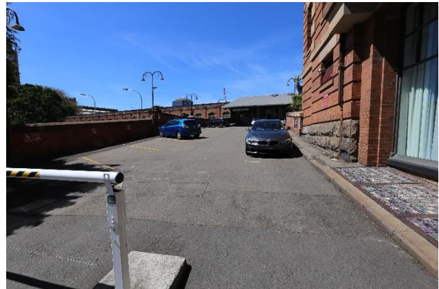
Figure 41 – Upper Carriage Lane, with the southern side of the Lower Carriage Lane retaining wall at left and the Former Parcels Post Office at the right.
