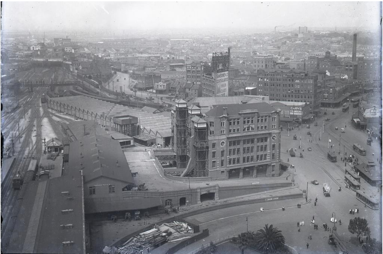
Figure 88 – Photograph of Central Station showing Inwards Parcels Shed, c. 1910s. The Parcels Post Office is located immediately on its right Source: OCP Architects, Heritage Report – Atlassian YHA, Railway Square (2017) , p. 15
