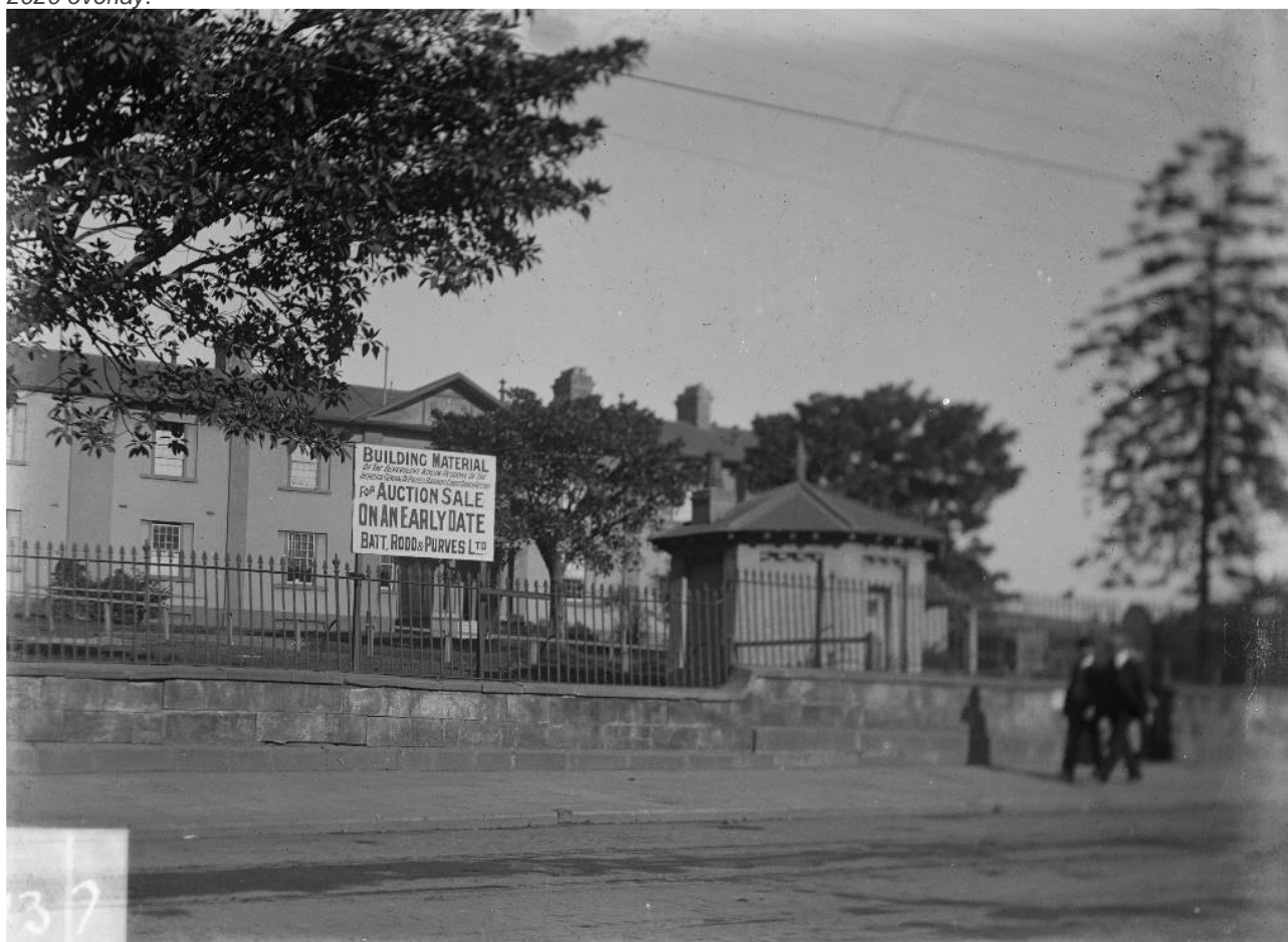
Figure 69 – Benevolent Asylum on Pitt Street, sign for the auction of building material in forefront in preparation for the demolition and construction of Central Station. Note the slight uphill incline
