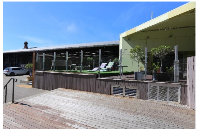
Figure 13 – Open deck area to the north of the dining and lounge addition
