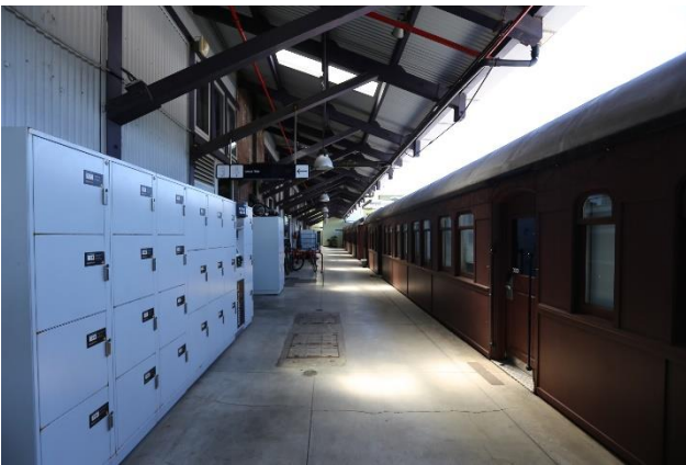
Figure 16 – Concrete platform at the east of the building, looking north.
