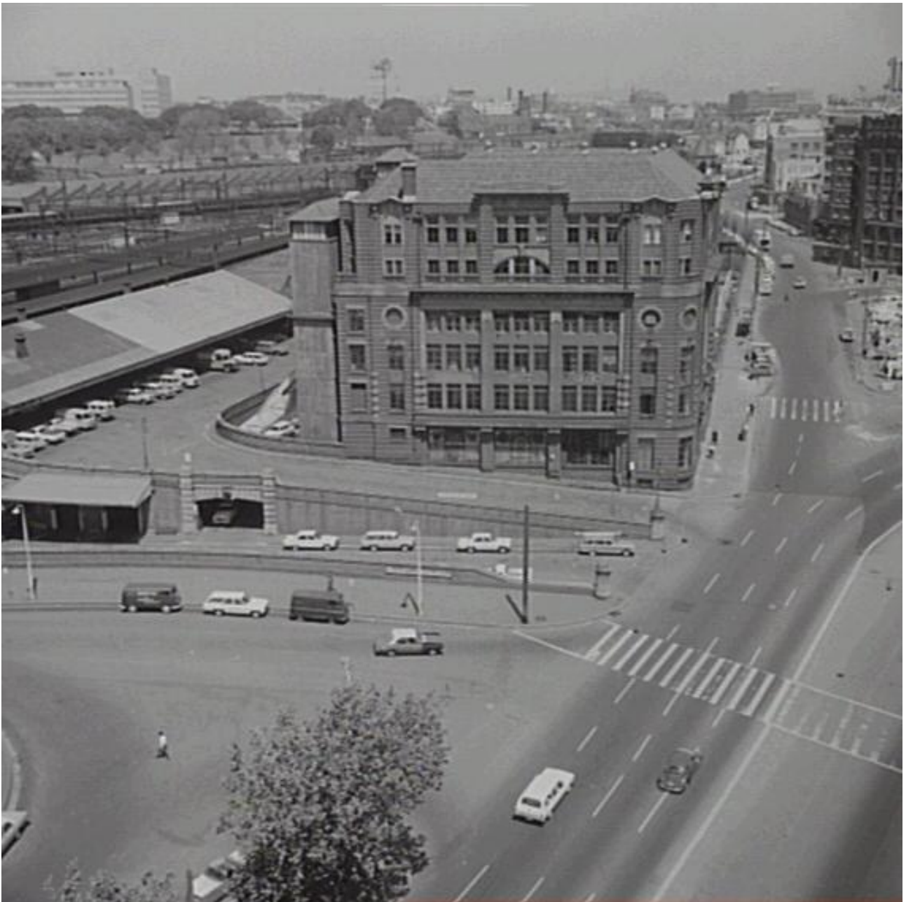
Figure 91 – View of Parcels Post Office and the Inwards Parcels shed on 10 October 1967 Source: City of Sydney Archives, NSCA CRS 48
