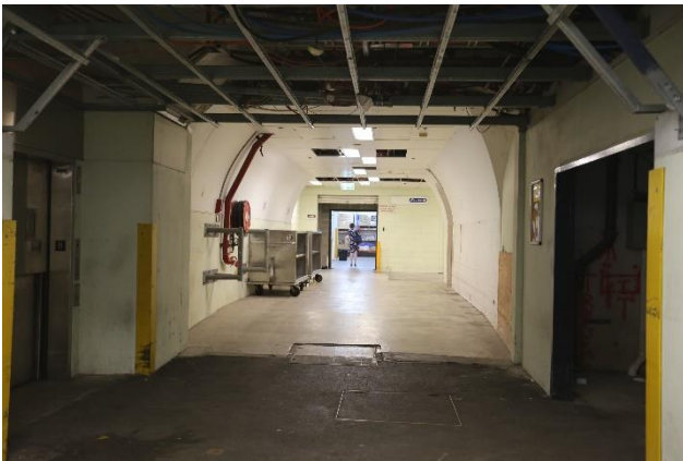
Figure 48 – Tunnel at north-east
