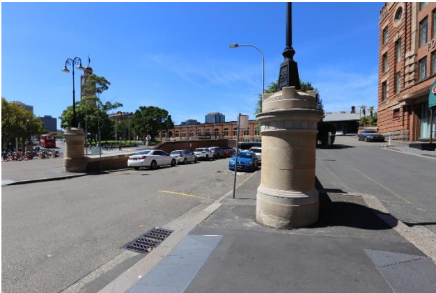
Figure 40 – Entrances to Lower (left) and Upper (right) Carriage Lanes and rounded sandstone piers.
