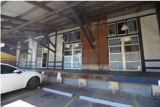
Figure 10 – Masonry piers on sandstone plinth at western elevation.
