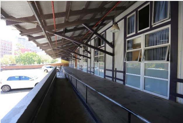
Figure 22 – Loading dock at east of building
