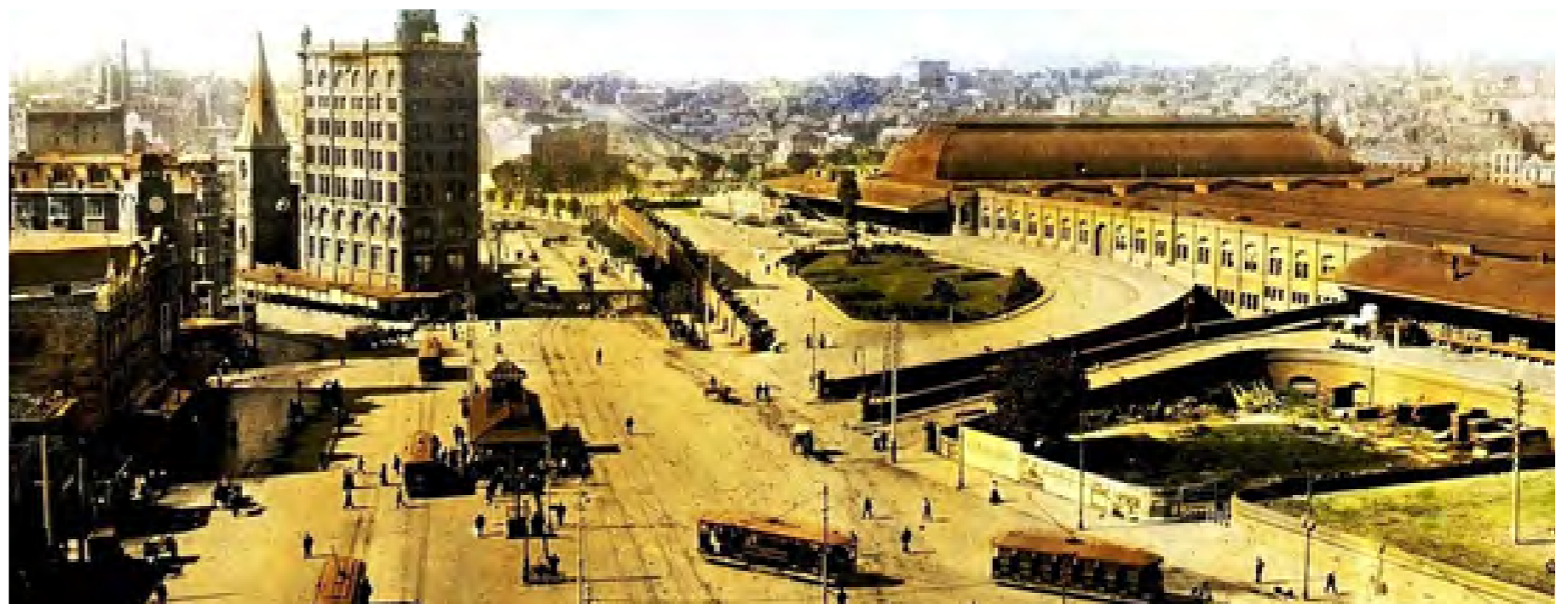
Figure 8 c. 1906-1913 view of Railway Square, with the Inwards Parcels Shed indicated by the red arrow at the right. Source: Flickr
