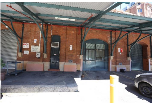
Figure 46 – Three arched openings that give access to the Former Small Parcels Bagging Room
