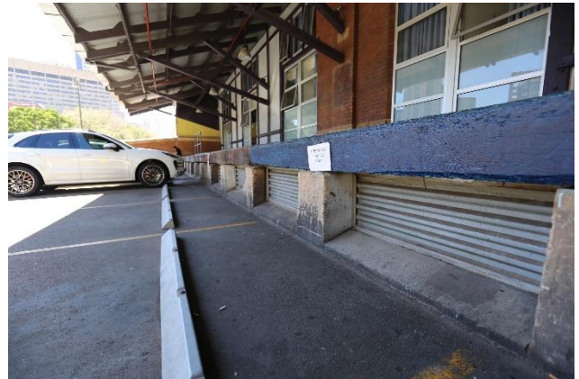
Figure 23 – Skylights under Loading dock and timber sleeper edging.
