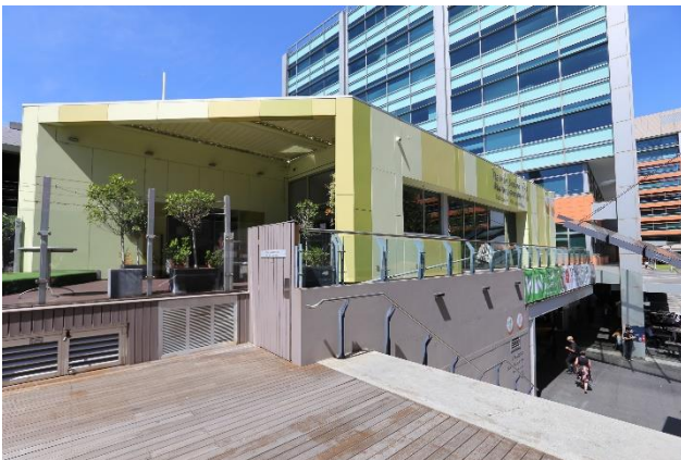
Figure 12 – Dining and lounge addition at south-west of building
