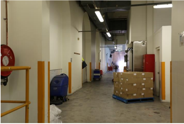
Figure 52 – Blind arches to the west of the coolrooms
