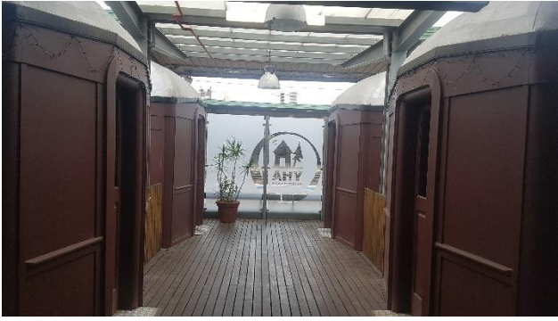
Figure 20 – Timber boarded platform and frosted glass screen.
