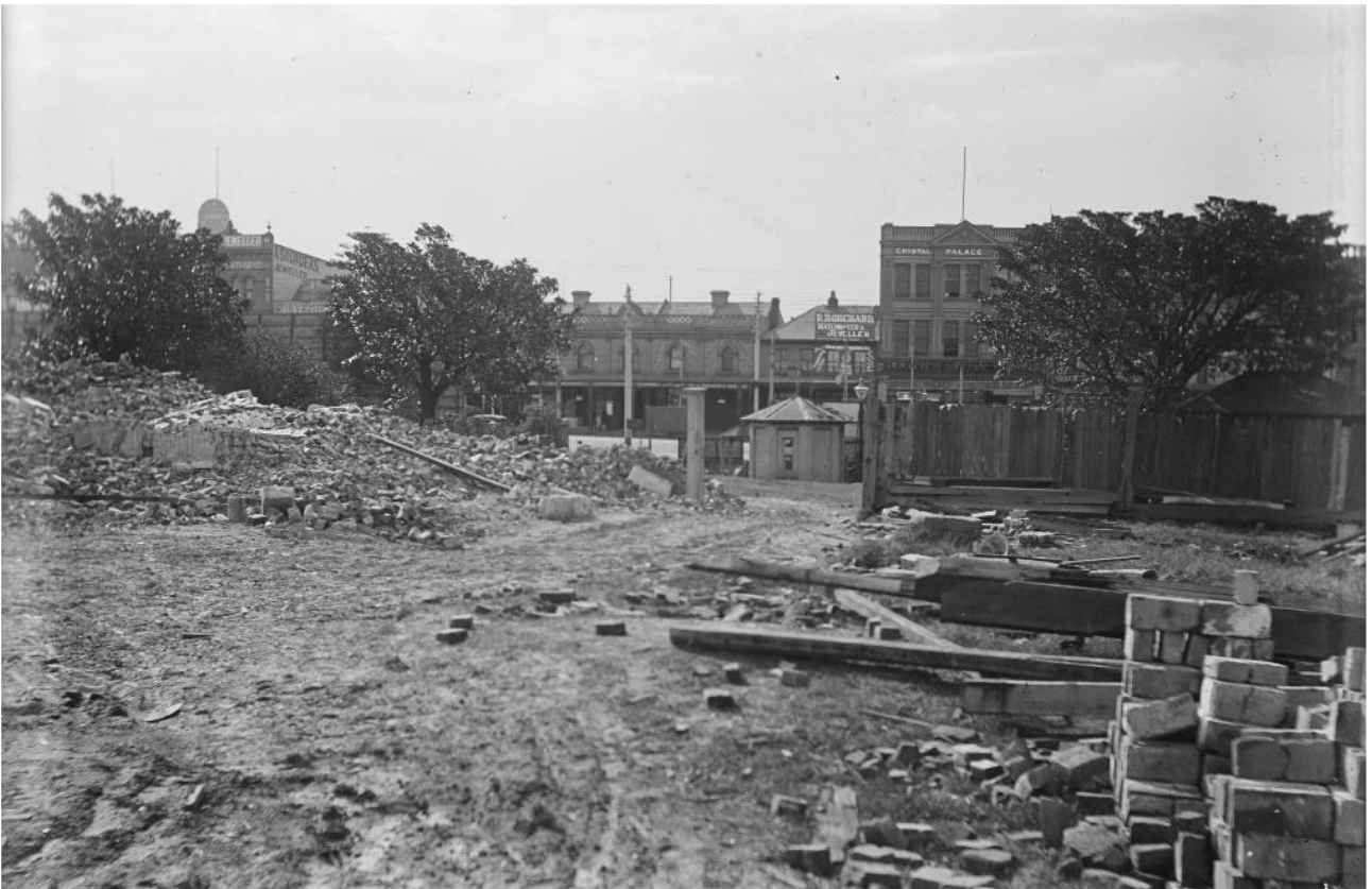
Figure 70 – 1901-1902 Benevolent Asylum after demolition, looking towards Pitt Street Source: State Library of NSW, IE8952327, Royal Australian Historical Society photonegatives
