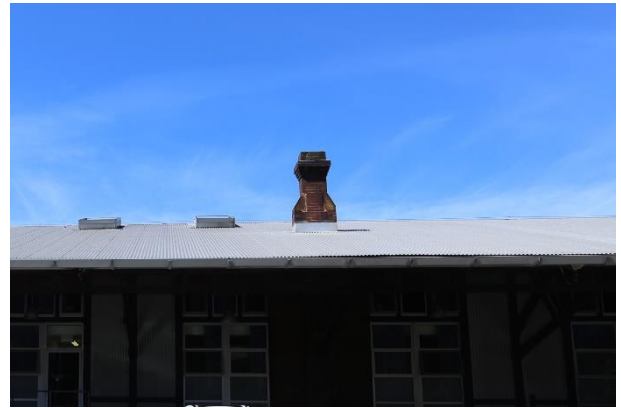
Figure 11 – Brick and sandstone corbelled chimney at west side of shed.
