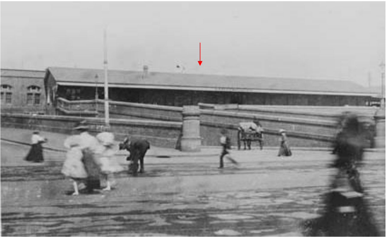
Figure 83 – Sydney Central Railway Station site, during the construction of the Parcels Post Office, c.1906-1913. The location of the Inwards Parcels Shed is indicated by the red arrow. Source: National Archives of Australia, Series No. C4076, Control symbol, HN16075B
