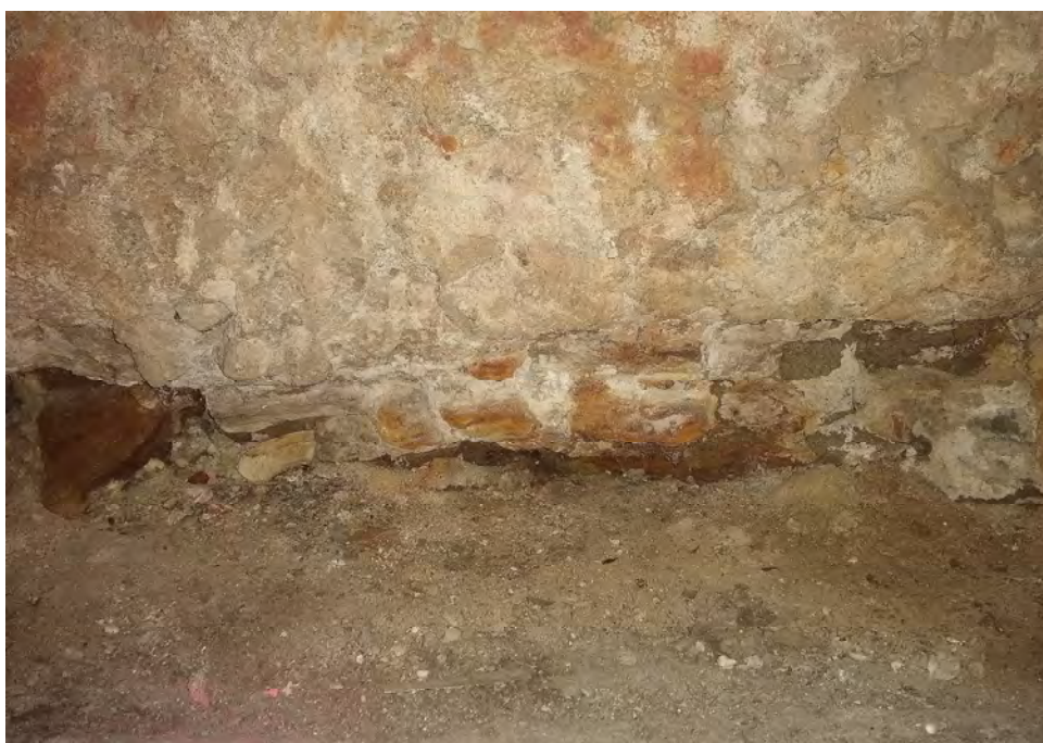
Photo 16 – View south-east within the Adina Hotel basement adjacent to Borehole W3, of sandstone exposed beneath the concrete underpin and just above the level of the basement floor slab.
