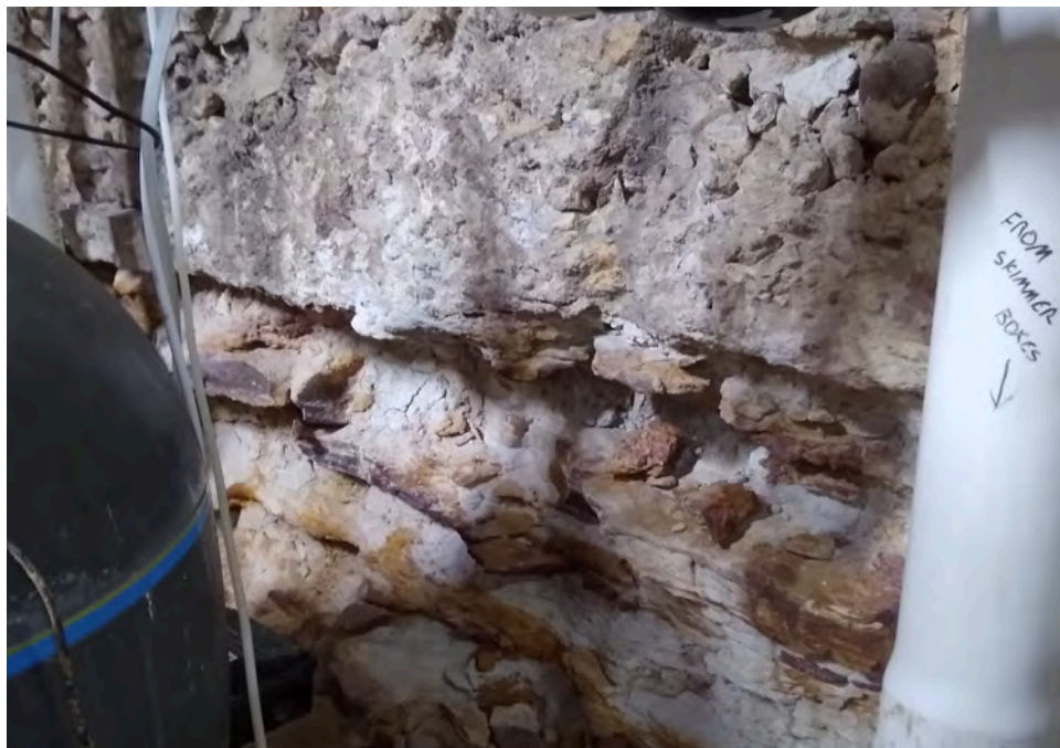
Photo 18 – View north of rock exposure observed adjacent to and west of the Adina Hotel basement entry ramp, of sandstone exposed beneath a concrete underpin. Multiple iron-cemented and clayey seams are present above the concrete floor slab.
