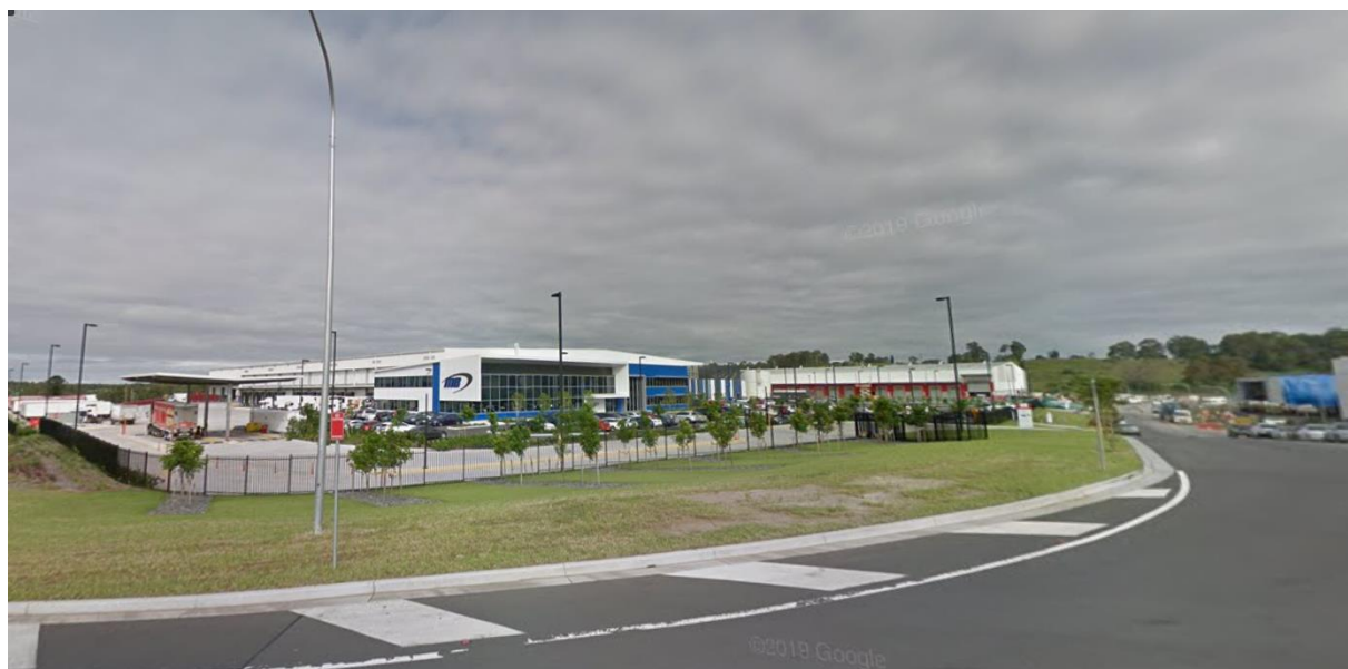
Figure 6 View to Horsley Drive Business Park Stage 1 development, looking south-west from Cowpasture Road / Burilda Close intersection
