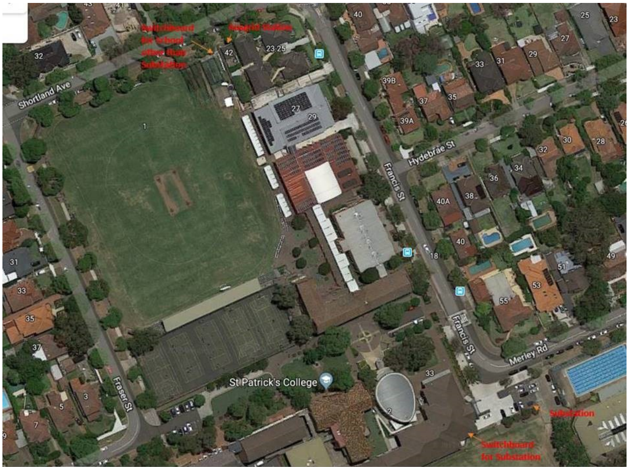
Figure 1 - Existing Power Supplies to the Site 1. Northern supply – Top of the image 2. Southern Supply – Bottom of the image
