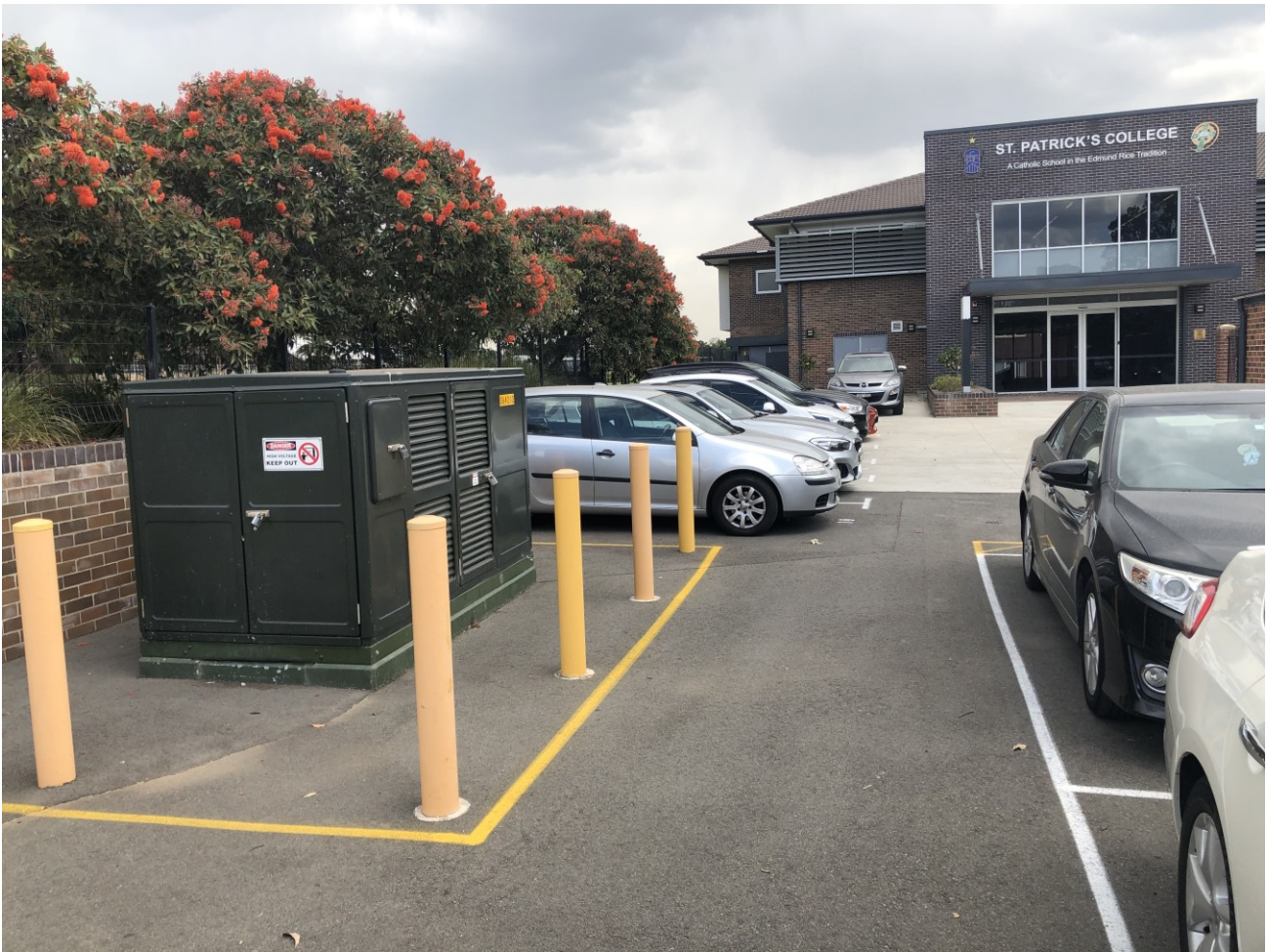
Figure 2 – Existing Kiosk substation (Southern supply) ARTS Building is in the background
