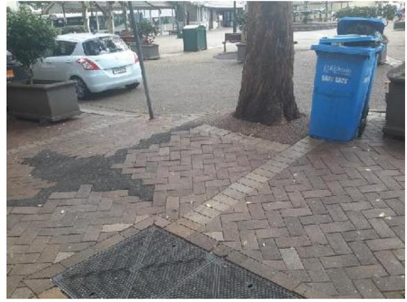
Uneven brick footpath, results in trip hazard due to tree roots AT-Strathfield Square
