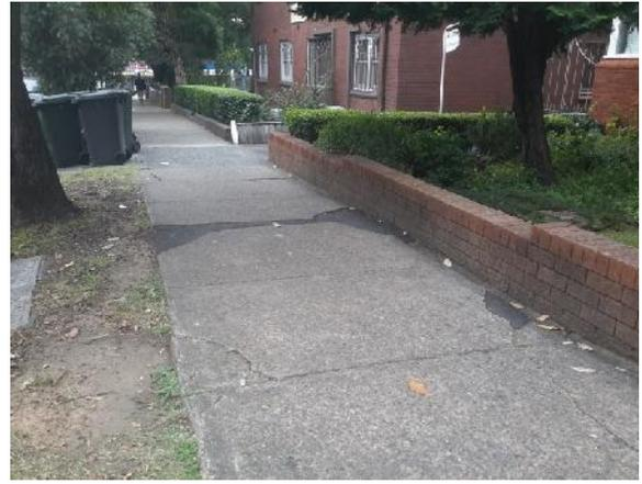
Cracked and uneven footpath on eastern side of The Boulevard
