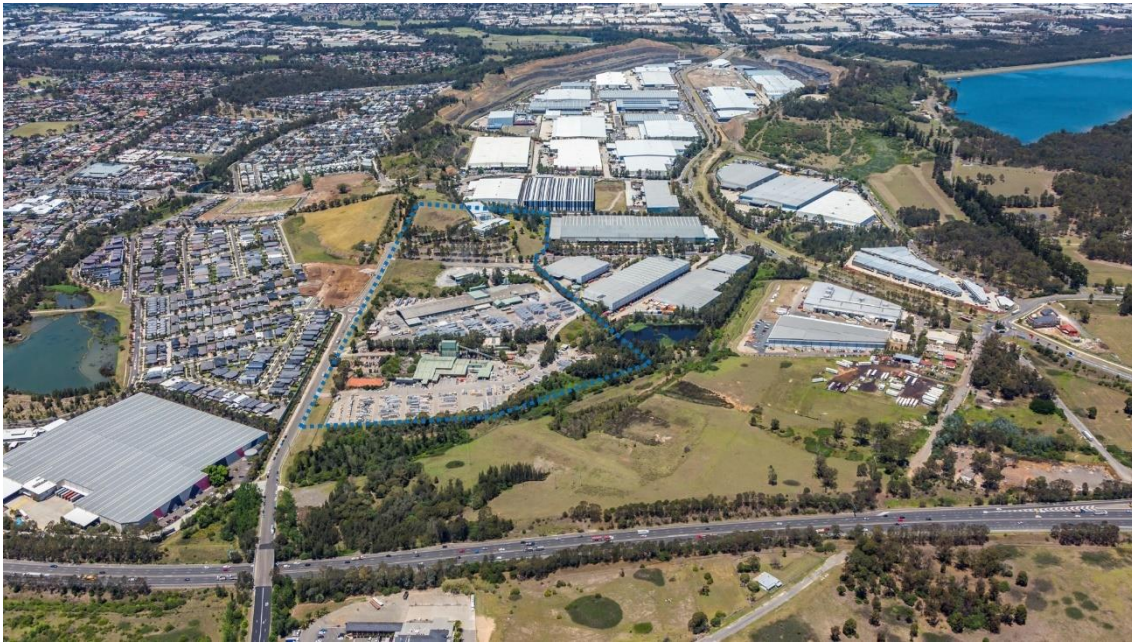
Figure 1: Aerial Image (Source: ISPT)
