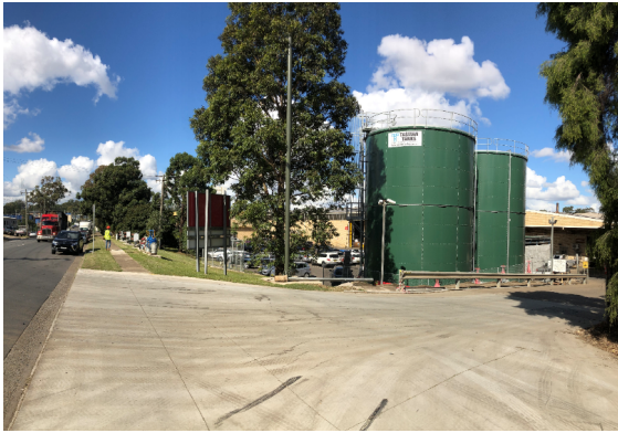
Central site entrance and fire hydrant water storage tanks.
