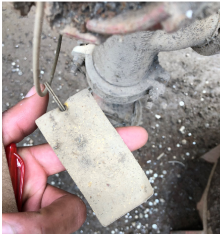
Unreadable maintenance tag (FH27).
