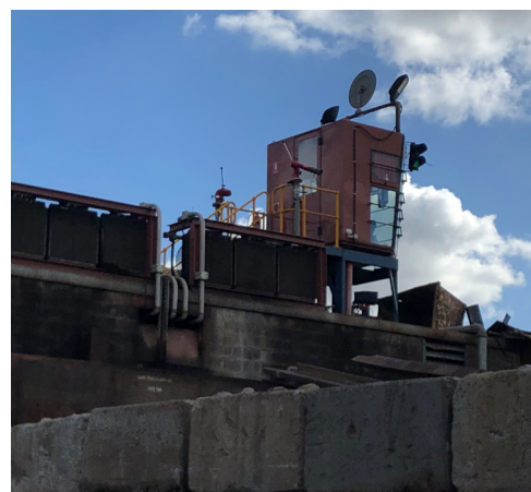
Existing water cannons at existing pre-shear
