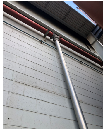
Supply from old sprinkler pipe for fire hydrant (FH30) not shown on block plan.
