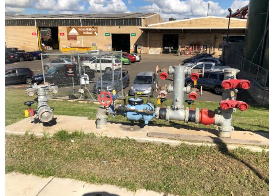
Fire hydrant booster assembly
