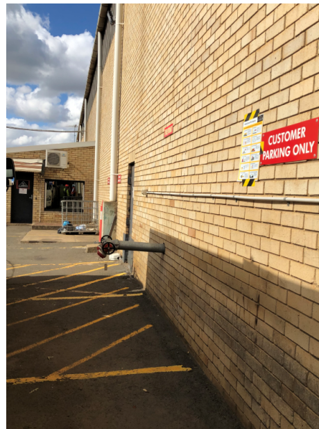
FH 3 missing adequate support and bollard
