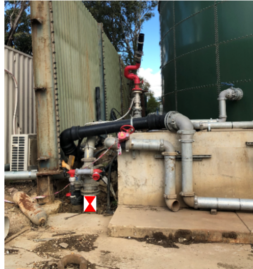
Isolation valve required for FH22 shown above
