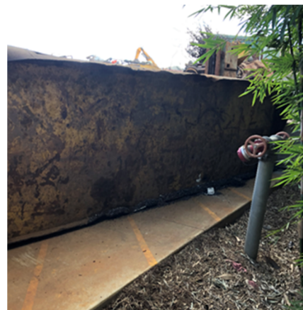
External fire hydrant obstructed by plant equipment
