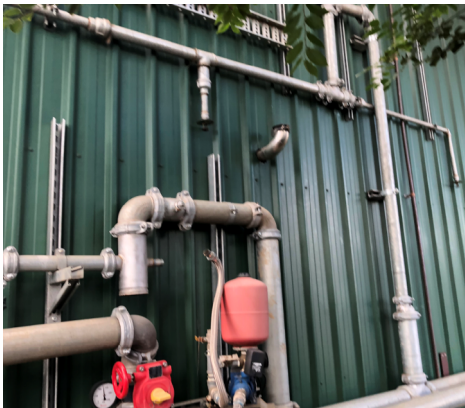
Drencher control valve.
