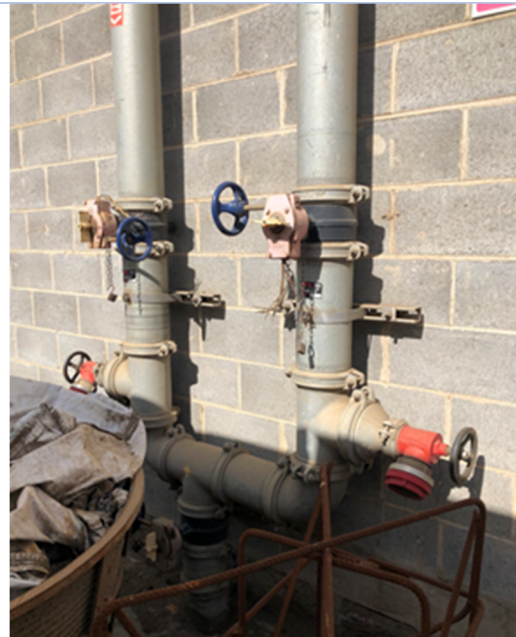
FH10 and FH11 obstructed by equipment
