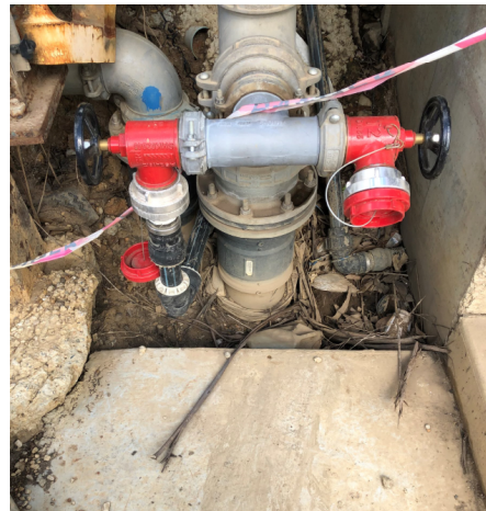
Fire hydrant installed too low (~600mm)
