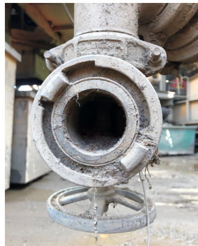
Fire hydrant (FH27) blocked with debris.
