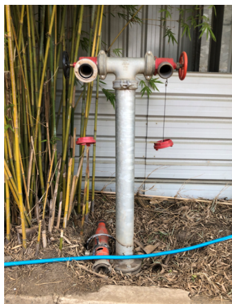
Existing external fire hydrant
