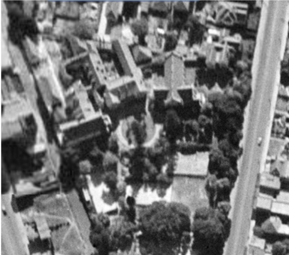
Figure 17: Aerial photograph showing the subject site in 1943. (Source: NSW LRS, SIX Maps).
