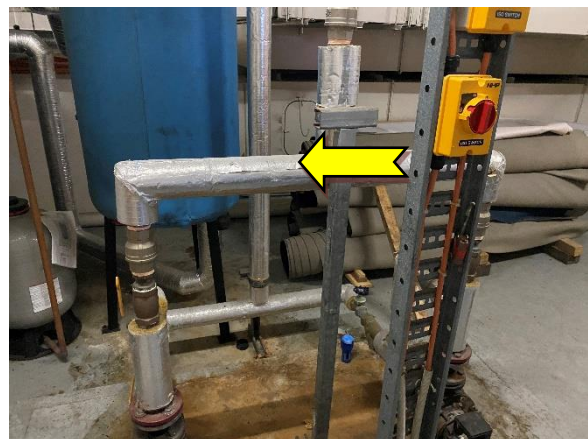
Photo 6 Interior: plant room, pipe work – suspected SMF containing external insulation material.
