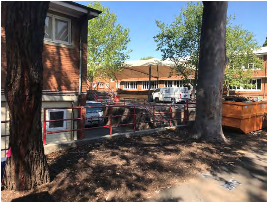
Photo12: Area adjacent to BH17 looking south west
