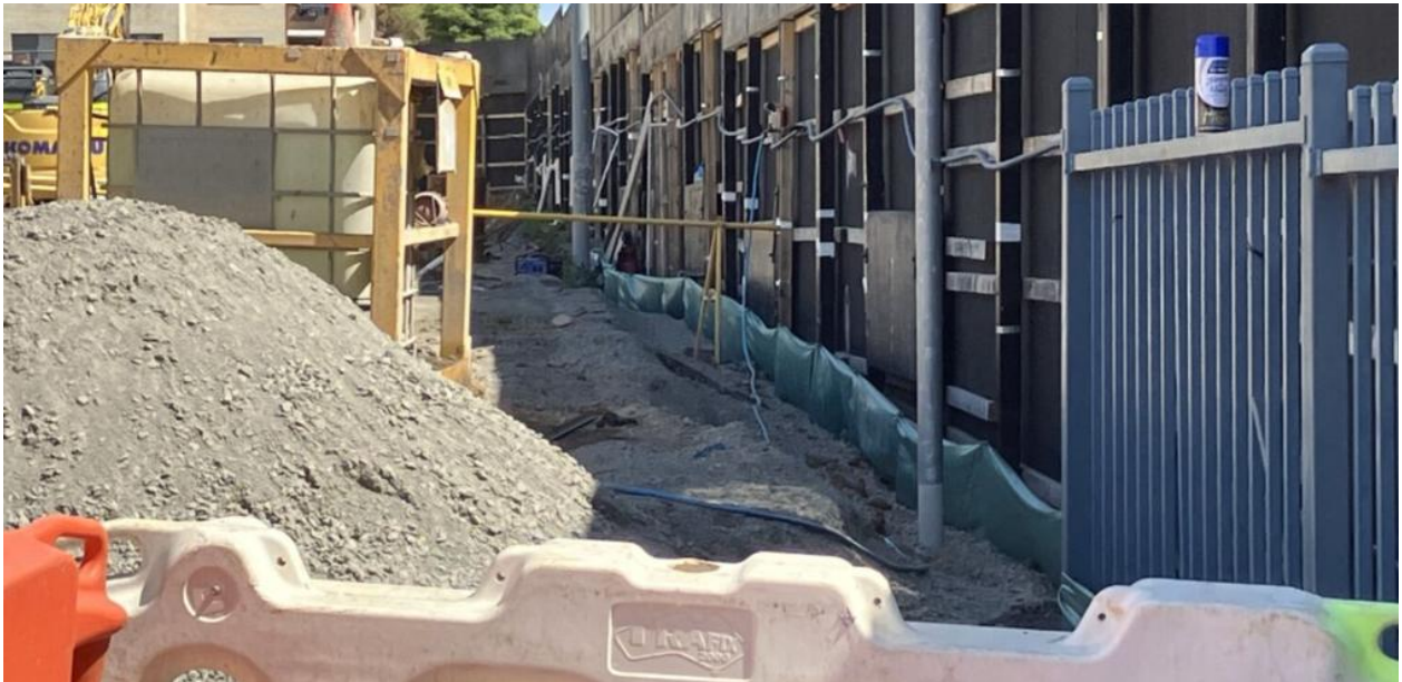
Sediment fencing at hoarding alongside Campbell Street.
