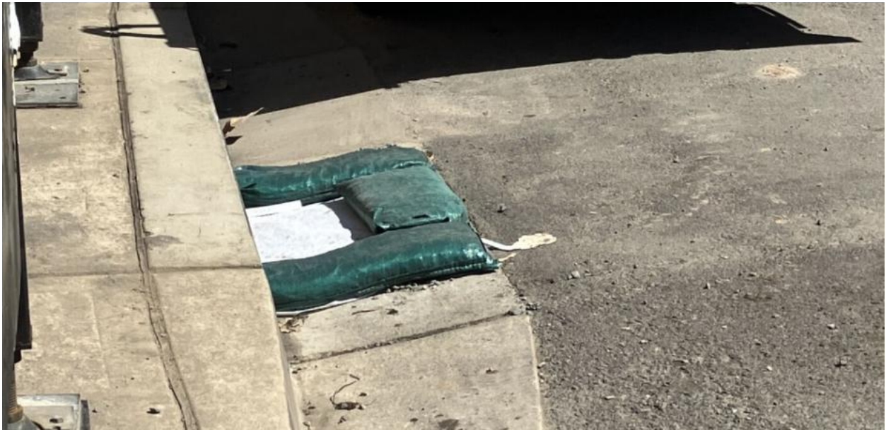
Good protection measures in place on Campbell Street
