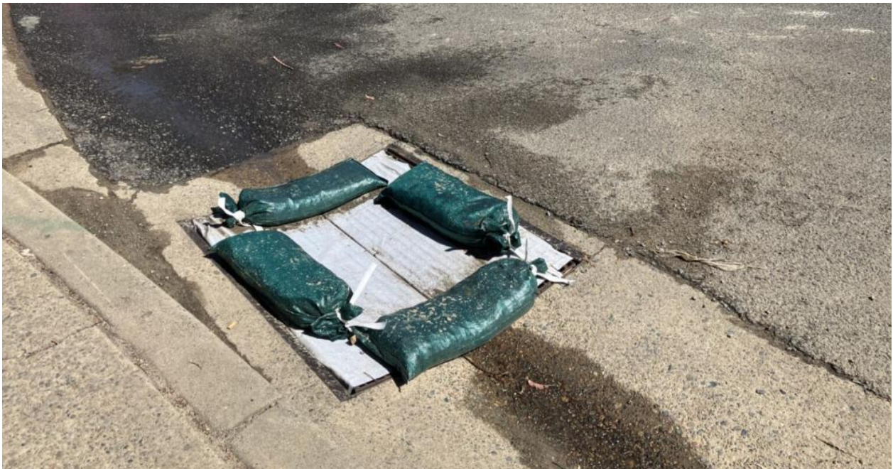
Effective controls demonstrated at Campbell Street
