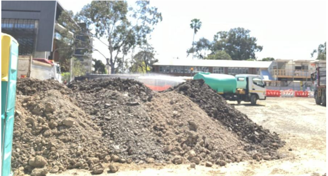
Water cart deployed during inspection to manage dusty conditions (OBS-01)
