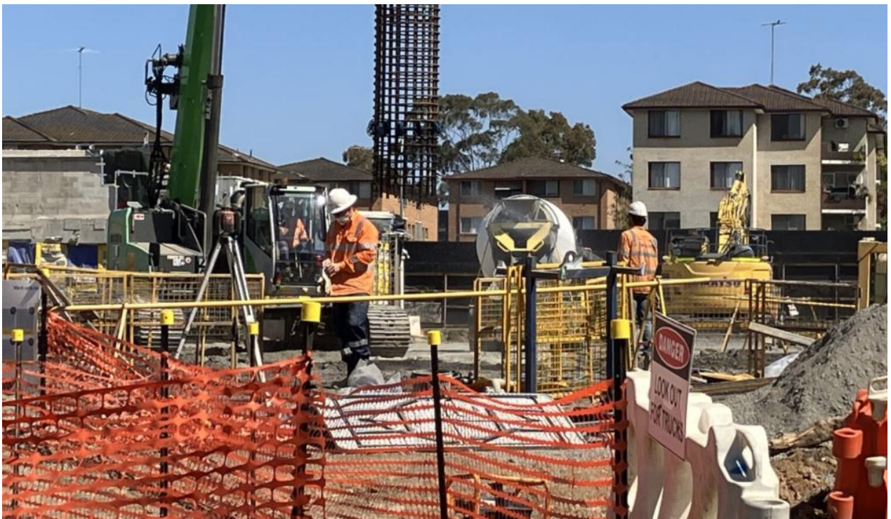
Worker using hose during piling works
