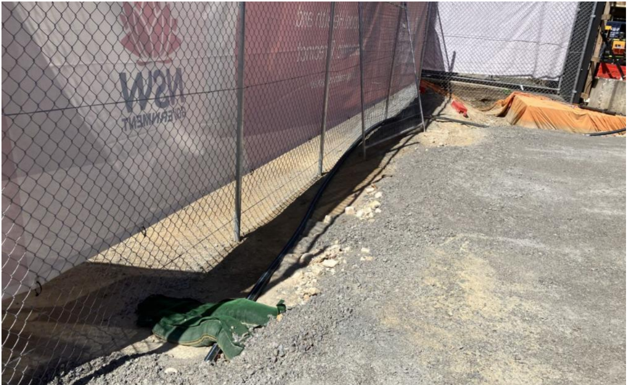
Water diversion in place.
