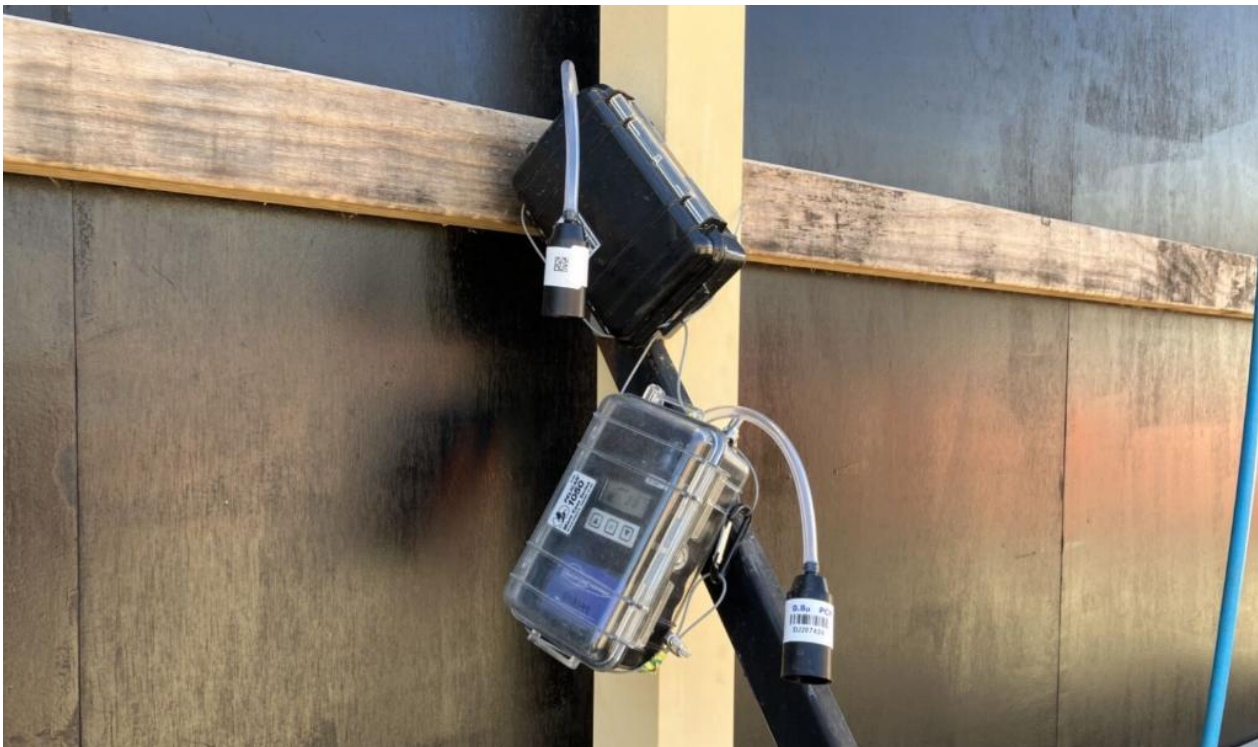
Ambient air monitors installed during demolition works
