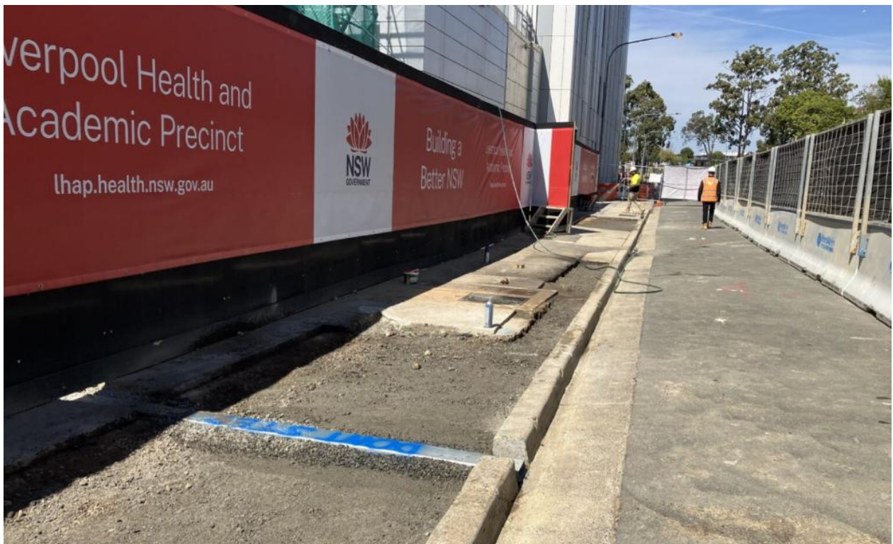
Upcoming concrete pour for remaining works at Goulburn Street
