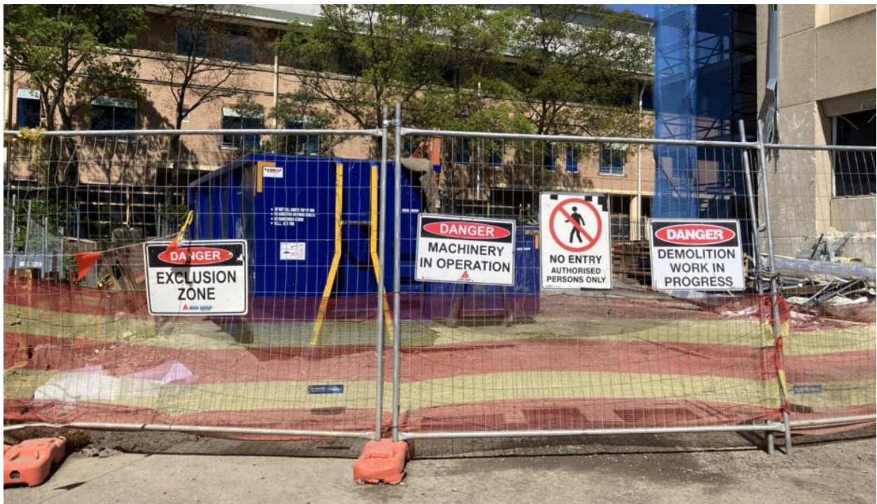
Delta Group exclusion zone for demolition of Alex Grimson building
