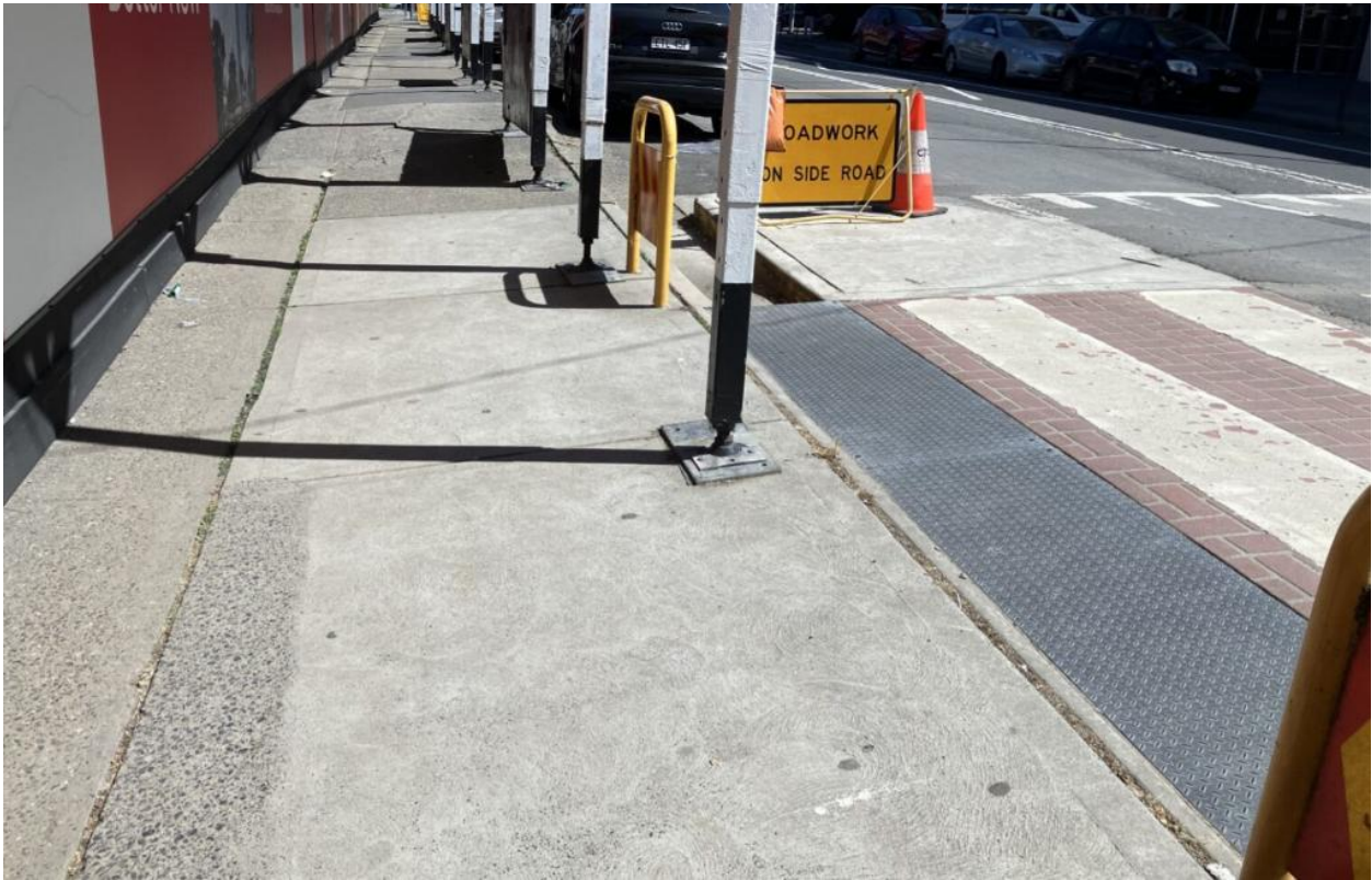
Traffic control signage in place at Campbell Street crossing
