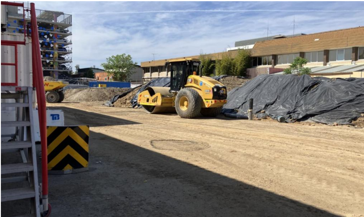
Future on-grade car park area currently used for laydown and storage
