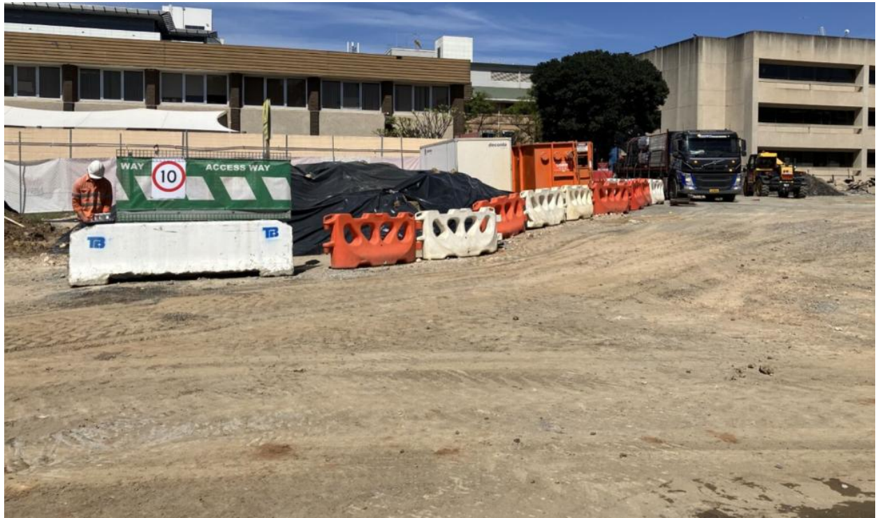
Consultant present onsite taking soil testing samples
