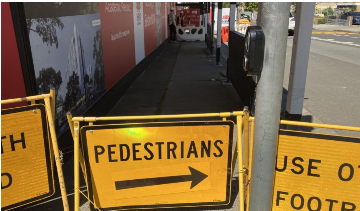
Pedestrian detour signage while works are occurring on Goulburn Street
