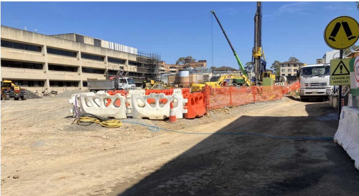
Heavy vehicle using designated route within site boundary
