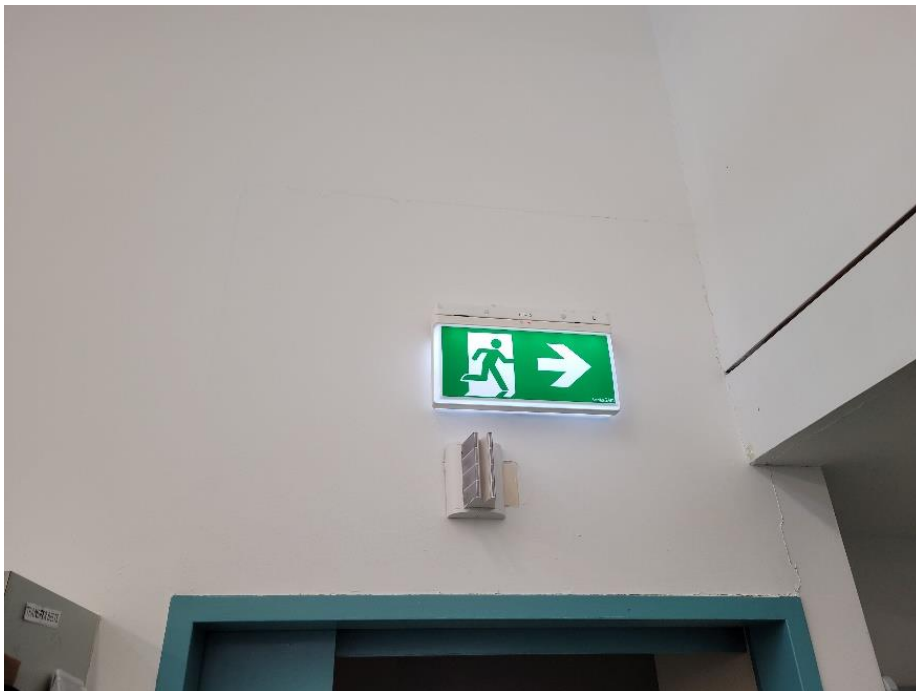
54. Vertical cracking along wall around door frame, continuing up to the higher section of wall
