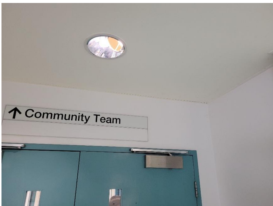
18. Crack in plasterboard at wall and ceiling junction
