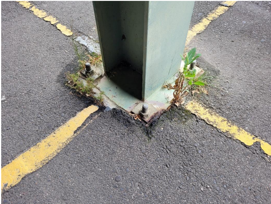
Existing Carpark 3. Signs of minimal ongoing maintenance
