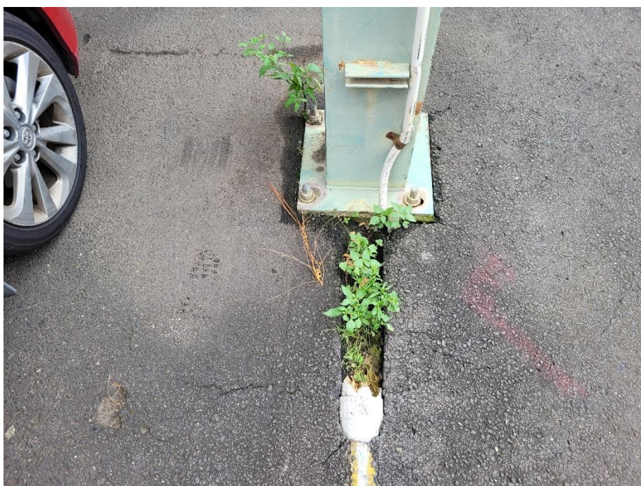
Existing Carpark 2. Signs of minimal ongoing maintenance
