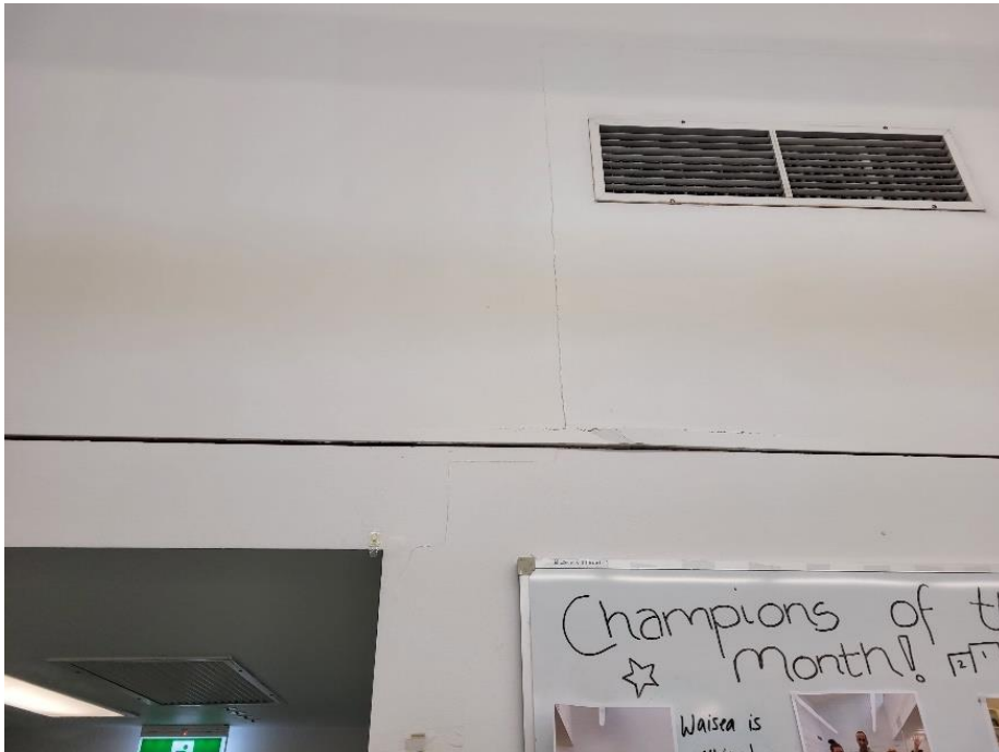
53. Vertical cracks in plasterboard in higher section of wall
