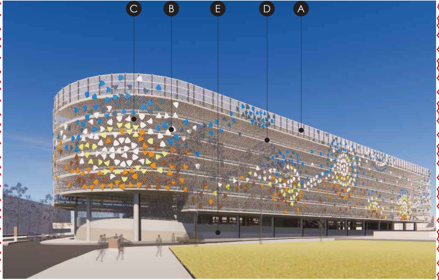
B ALUMINIUM PANELS FIXED TO TENSILE WIRE MESH COLOUR 01 DARK BLUE COLOUR 02 MID BLUE COLOUR 03 LIGHT BLUE COLOUR 04 WHITE COLOUR 05 GREEN COLOUR 06 LIGHT BROWN COLOUR 07 DARK BROWN
