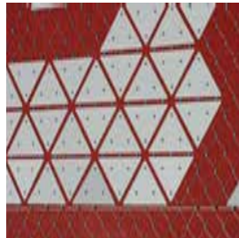
B ALUMINIUM PANELS FIXED TO TENSILE WIRE MESH COLOUR 01 DARK BLUE COLOUR 02 MID BLUE COLOUR 03 LIGHT BLUE COLOUR 04 WHITE COLOUR 05 GREEN COLOUR 06 LIGHT BROWN COLOUR 07 DARK BROWN
