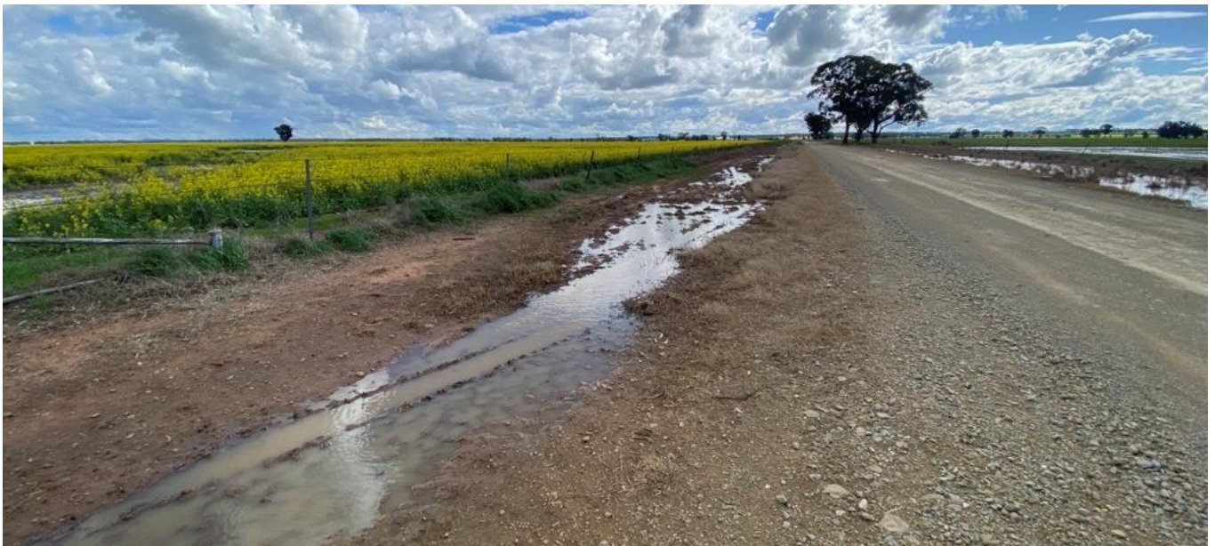
Photo 3 Existing Troubalgie Road, including table drains along either side of the road
