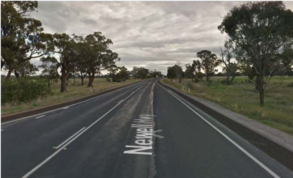
Figure 2-23: Street view of sight line from NB vehicle on Newell Highway to vehicle turning into Forest Road
