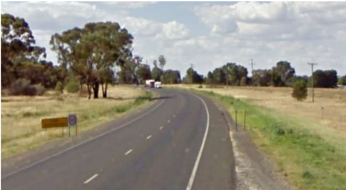
Figure 2-24: Street view of sight line from SB vehicle on Newell Highway to vehicle turning into Forest Road
