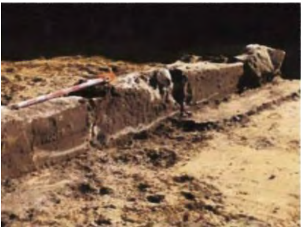
Figure 20 – stone and slurry footing
