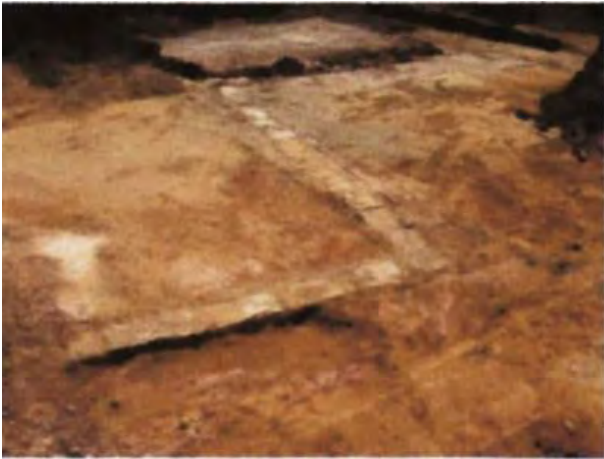
Figure 18 – sandstone footings
