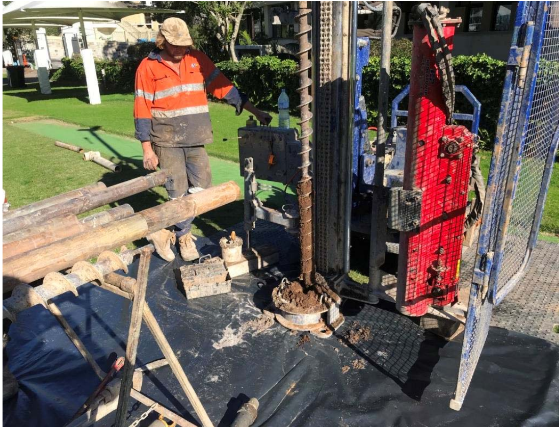
Photo 3 - Fill from BH106, rig set-up with track mats (11/07/2019)
