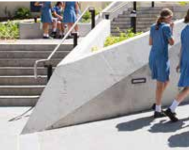
Off-form Concrete Retaining walls
