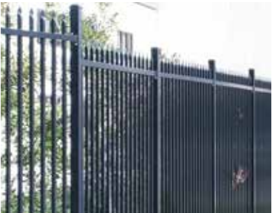
1.8m Security Perimeter Fence
