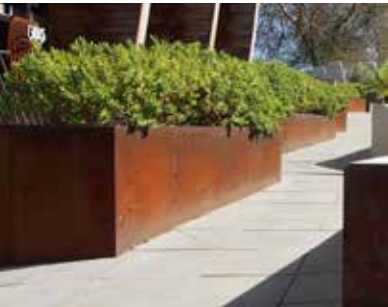
Corten Steel Retaining walls (up to 600mm)
