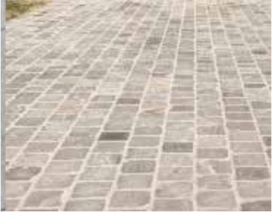
Large Format Stone Unit Pavers
