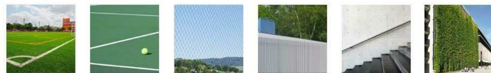
TURF COURT SURFACE FENCE BALUSTRADE CONCRETE GREEN WALL Synthetic multi-sport turf All-weather acrylic hardcourt surface Stainless steel tensile webnet fence Steel balustrade Off-form concrete floor and roof slabs Ref. to Landscape Arch Dwg.
