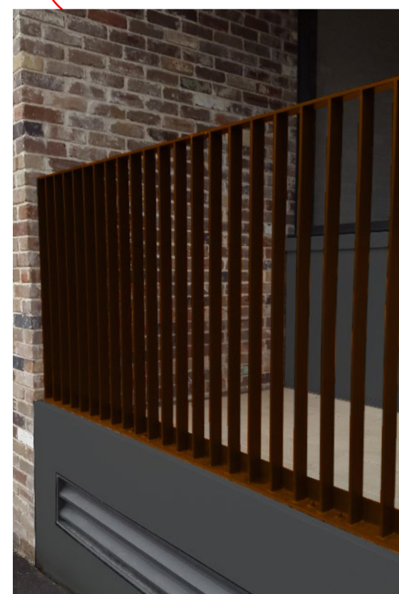
STEEL PALISADE FENCE
