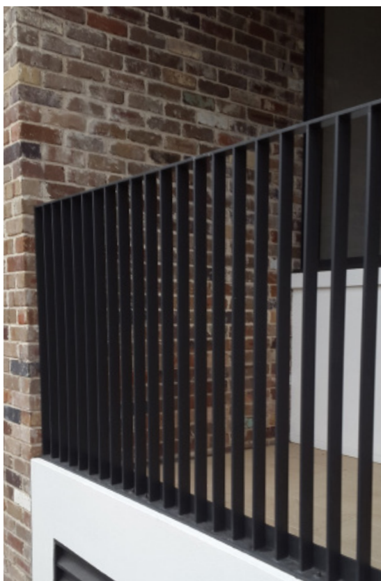
STEEL PALISADE FENCE
