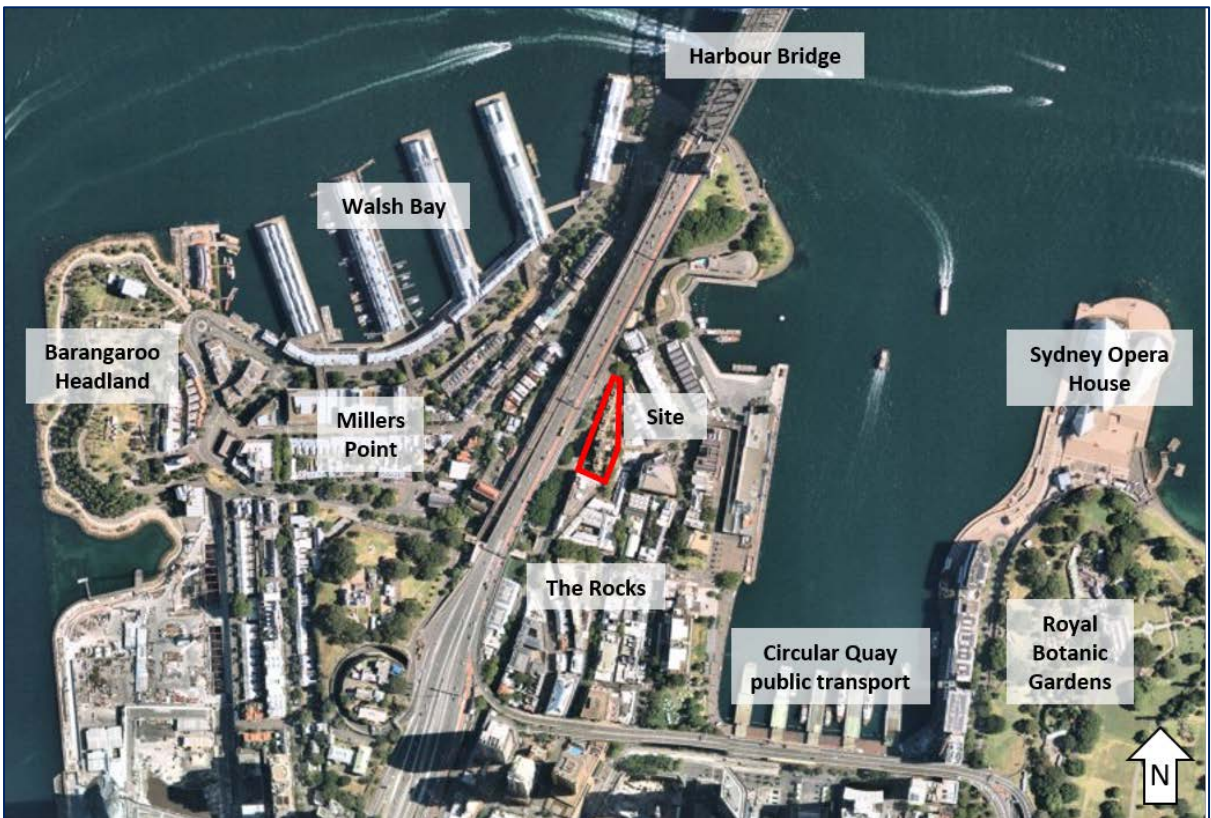
Figure 2 | Site location (Source: Nearmap)
