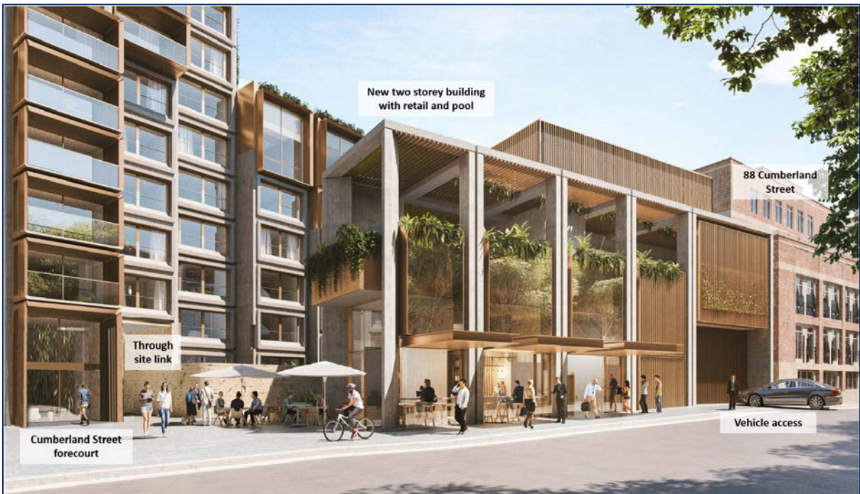
Figure 8 | Cumberland Street elevation, with public forecourt, through site link and new two storey building with retail tenancy, pool and vehicle access (Source: Applicant's FRtS Attachment B)
