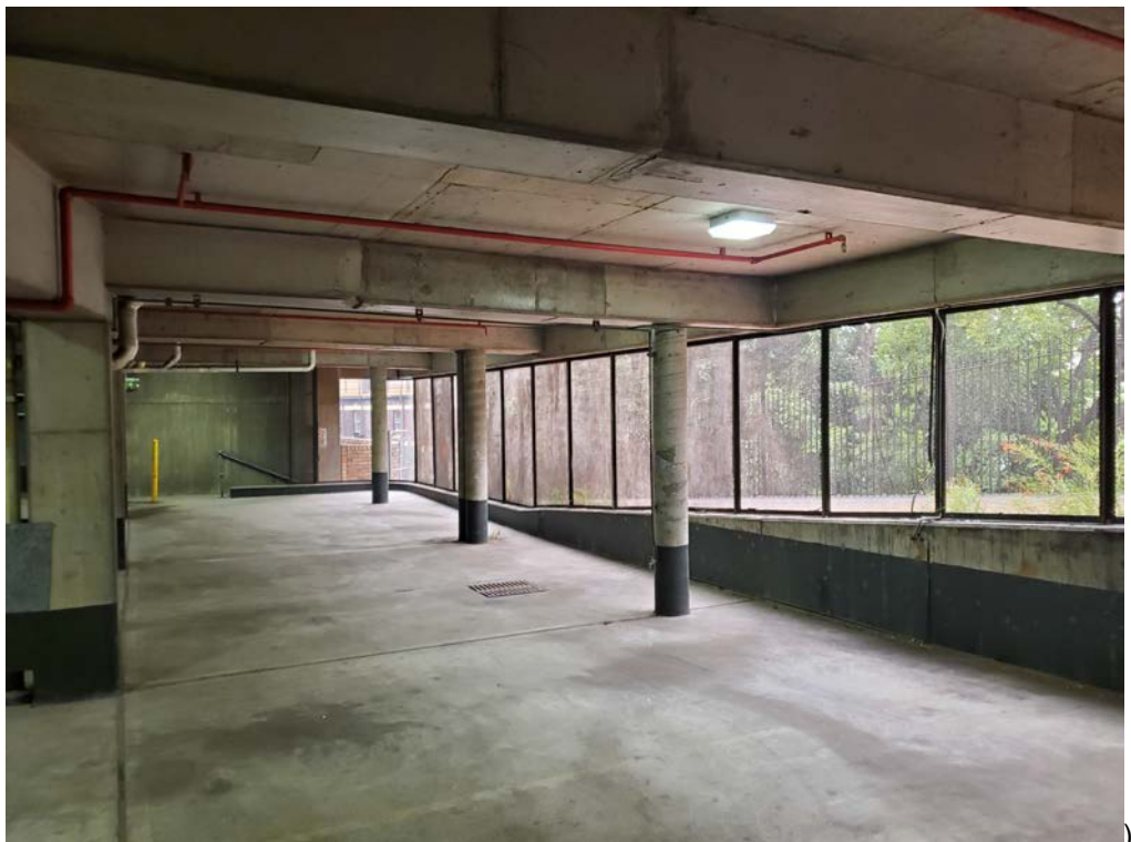
Photograph 2: First level basement (photo taken on 19/12/2019)
