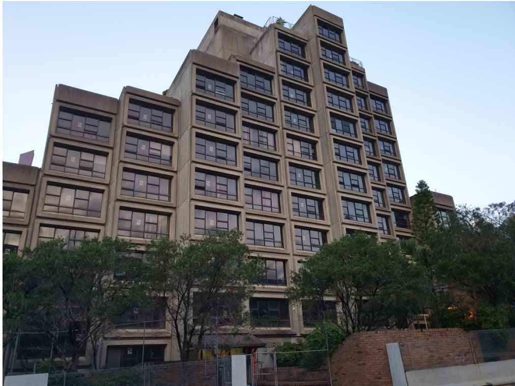
Photograph 1: Site overview, facing south-east (photo taken on 21/05/2020)
