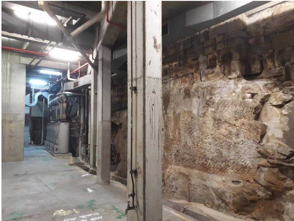
Photograph 3: Exposed sandstone bedrock in lower basement (photo taken on 05/06/2020)
